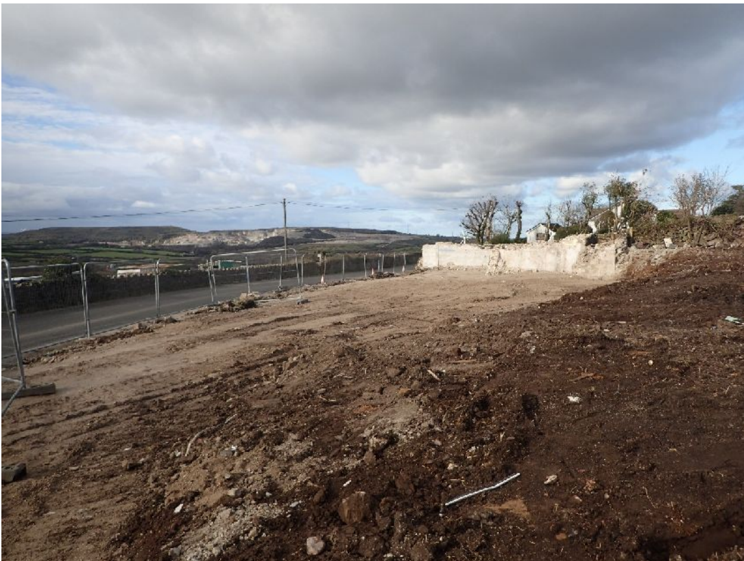
Plate 2. Site of the former Methodist chapel shortly after demolition from east
