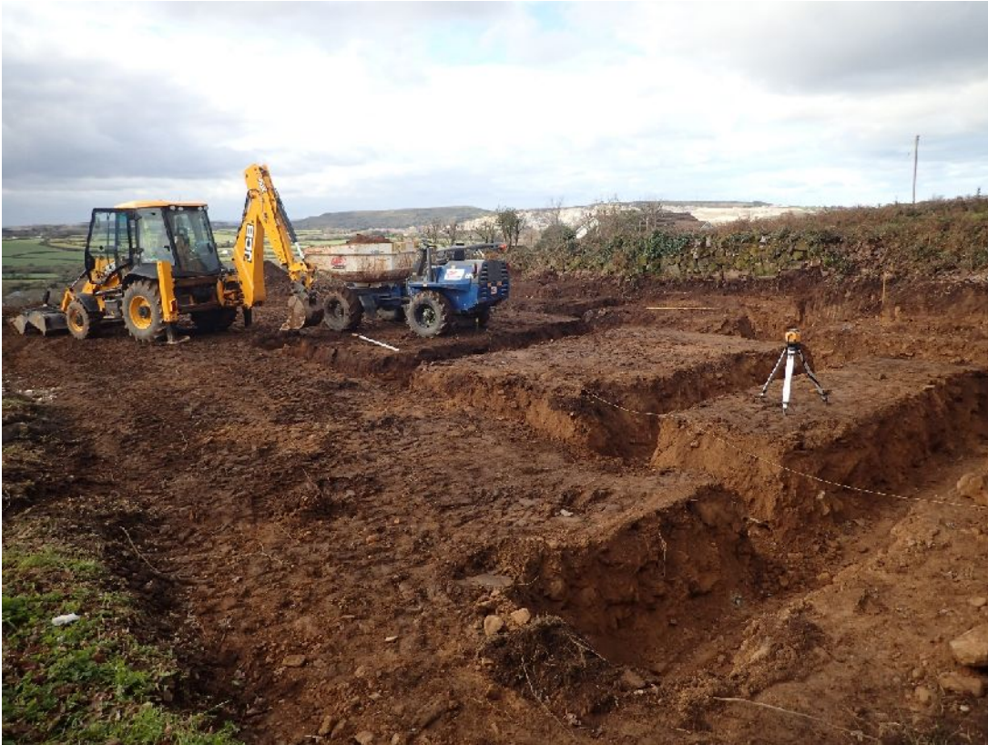
Plate 1. General view across the site during foundation excavations from north-east
