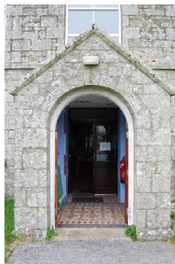
Plate 18. Front porch to church (1 x 2m scale; from SE)
