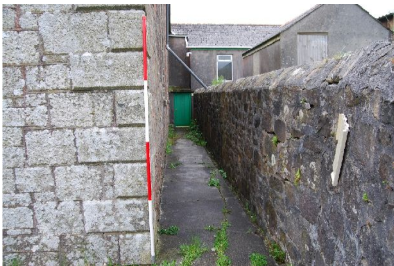
Plate 17. Walkway from front of church to outside w.c. & store (1 x 2m scales; from SE)
