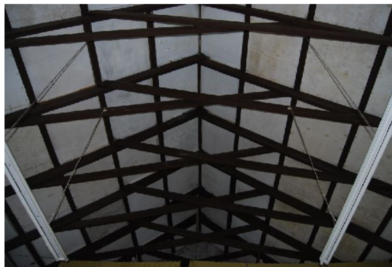
Plate 28. Scissor trusses of Sunday School hall (from SE)
