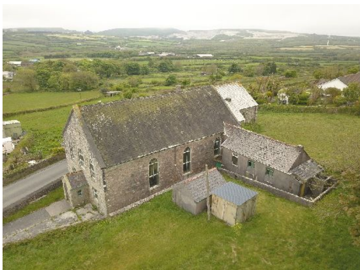
Plate 15. NE side of church showing mid-C20 extension & detached stores in foreground (from NE)
