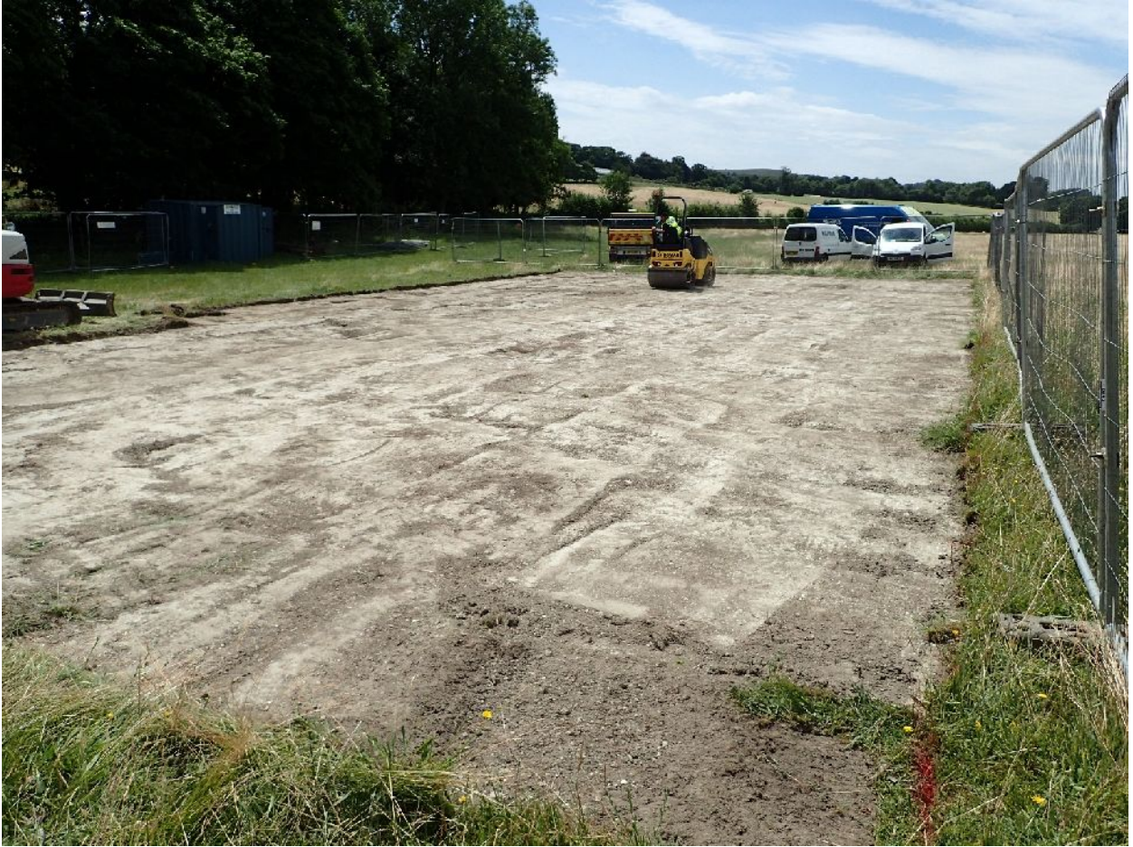
Plate 1. Compound with turf removed (facing S)
