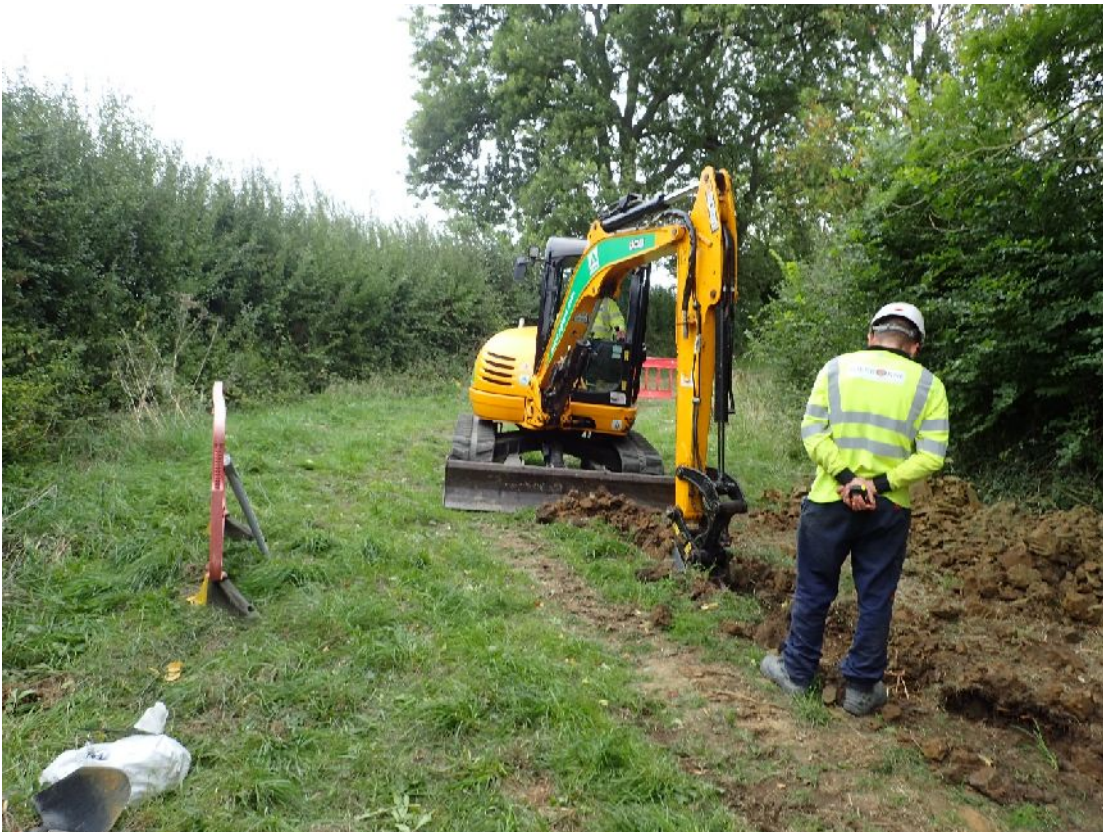
Plate 2. Working shot of open cut pipe trenching (from S, no scale)
