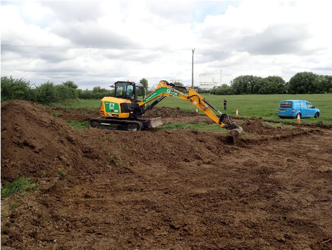
Plate 1. Site compound excavations (from S, no scale)
