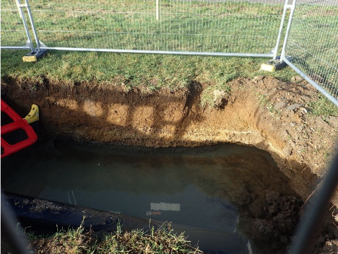
Plate 3. Drill pit 4 (facing SW)
