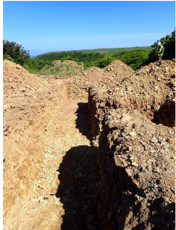
Figure 4. Foundation trenches (facing N; 1m scale)
