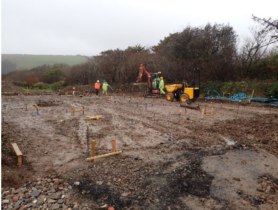
Figure 2. General shot across Site prior to ground reduction (facing NE)
