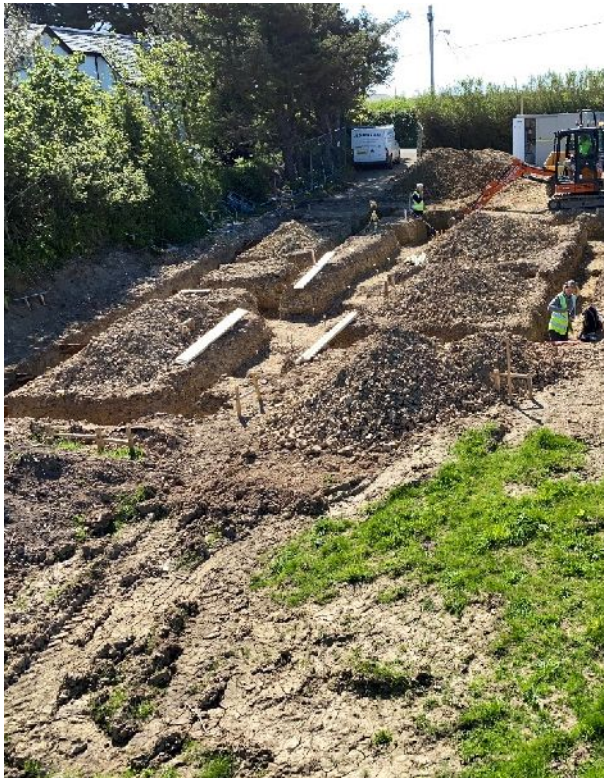
Figure 3. Foundation trenches (facing SSE)
