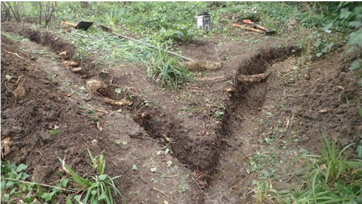
Plate 2. Trench to existing kiosk (facing W)
