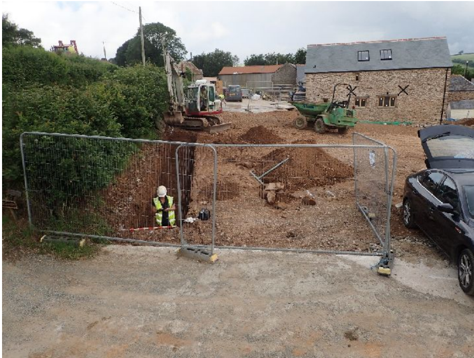
Figure 2. Working shot during trench excavations (facing W)
