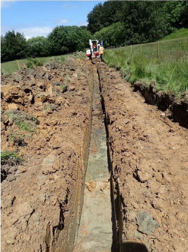
Plate 3. General view across the Site showing open-cut trenching from the south-east
