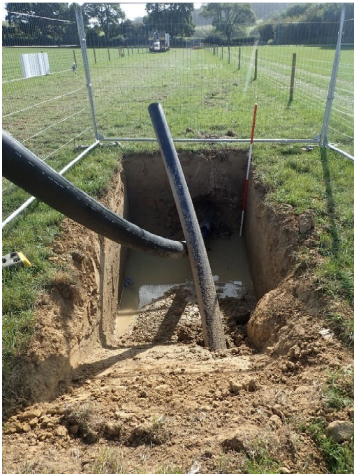
Figure 3. Directional drill pit 6 from the west showing typical intervention
