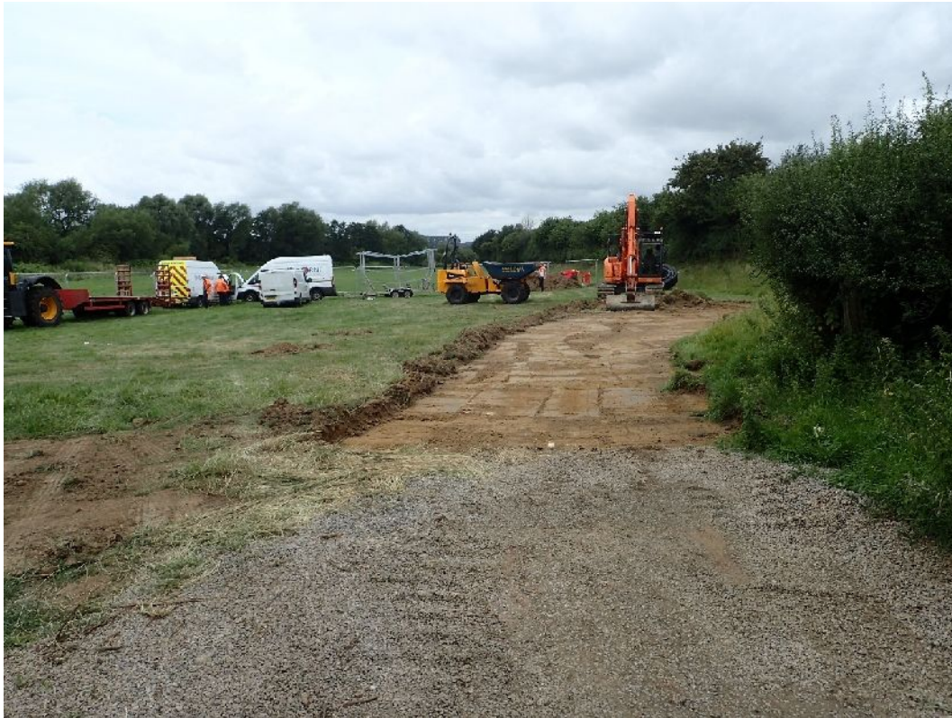
Figure 2. View showing topsoil stripping across the compound from the east
