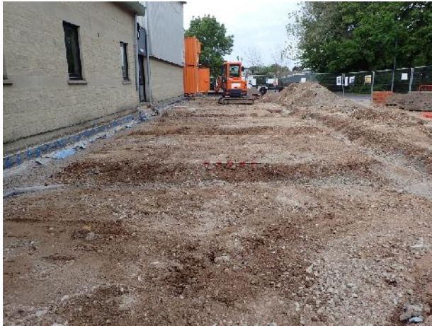
Figure 3. Foundation raft excavations (1m scale; from the W)
