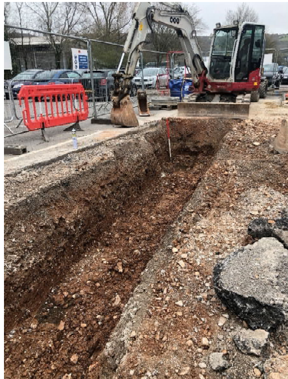
Figure 4. General shot of service trench excavations (1m scale; looking ENE)
