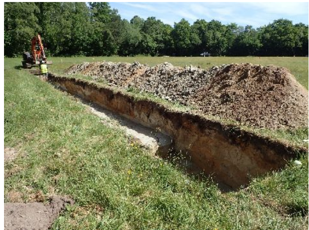
Figure 14. Working shot of Tr7 excavation (from the SW)
