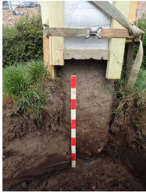
Figure 3. SE face of cross below ground level (looking NW; 1m scale)
