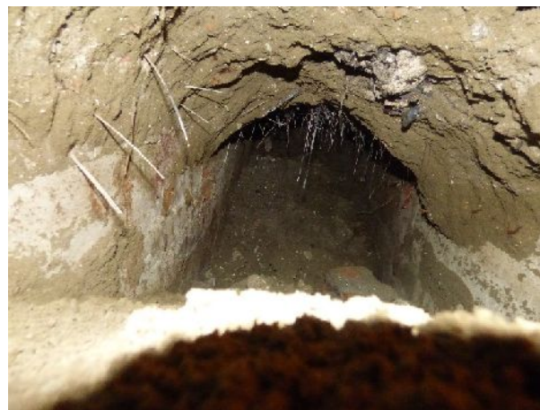
Figure 12. Interior of vault showing lime rendered walls & soil adhering to roof with coffin furniture protruding (looking W)
