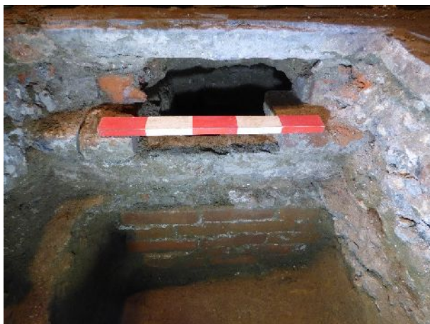
Figure 11. TH8 showing vault (looking S; 0.5m scale)
