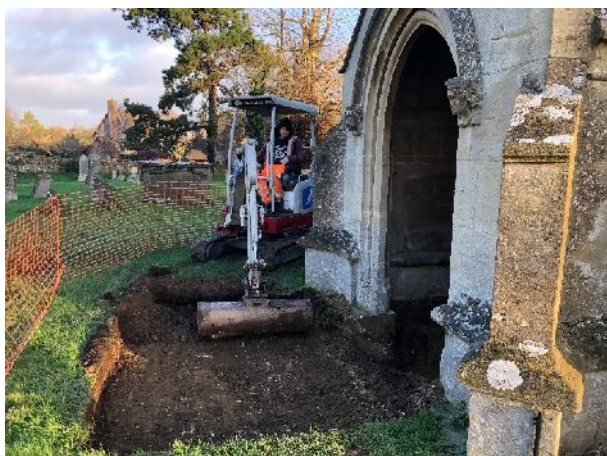
Figure 2. Ground reduction for new path adjacent to W porch (from S)
