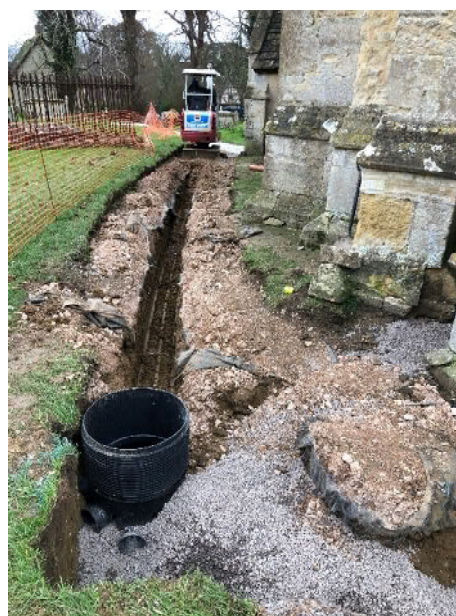
Figure 5. Pipe trench along N side of church (from WSW)
