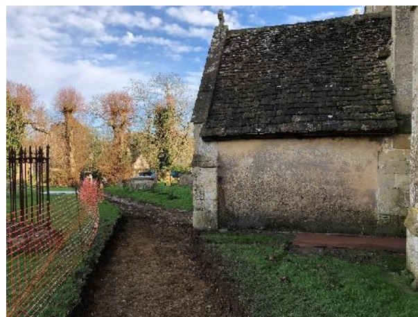
Figure 3. New path adjoining existing path to N porch (from W)
