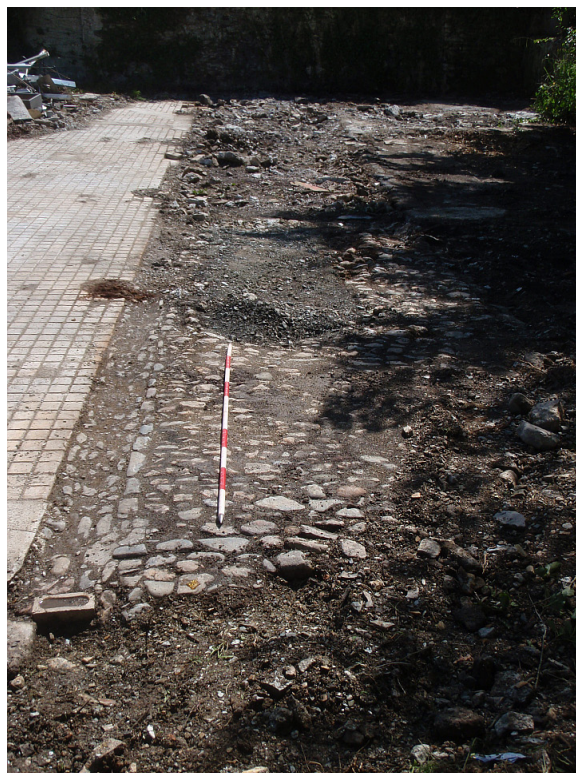
Plate 9. Cobbled alleyway (102)/(107) viewed from the west, with floor (115) and iron column bases (116), (117), (118) and (119) on the left.
