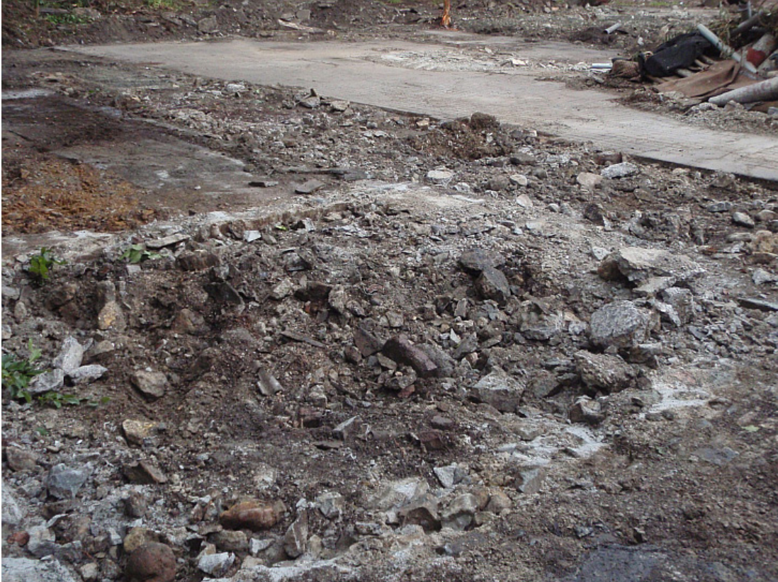
Plate 6. Southern Bone Mill building, viewed from the south east across sump (122).
