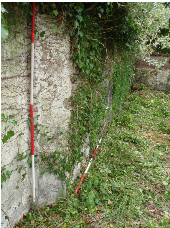
Plate 8 . Wall (101) viewed from the north showing chamfered corner of doorway.
