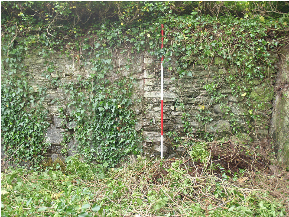
Plate 7. Blocked doorway near southern end of wall (101), viewed from the west.
