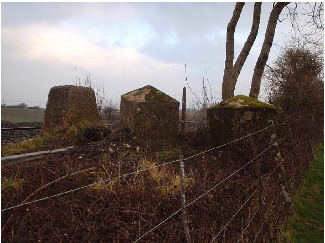
Plate 8: Northwest-facing view of anti-tank blocks straddling the railway line in Area B
