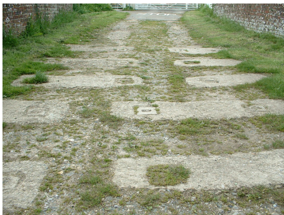
Plate 9: Roadblock sockets in Crofton on Kennet and Avon Canal; probably for a hedgehog vertical rail road block (Wikipedia 2010)
