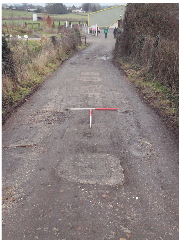
Plate 11: Vertical rail anti-tank sockets recorded on the northern edge of Axminster, during a walk over survey undertaken by COAS as part of a recent desk-based assessment (Hawtin, forthcoming)
