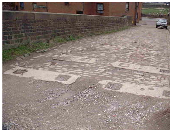
Plate 10: Roadblock sockets in Macclesfield, Cheshire; probably for a hedgehog vertical rail road block (Pillboxes.co.uk 2010)
