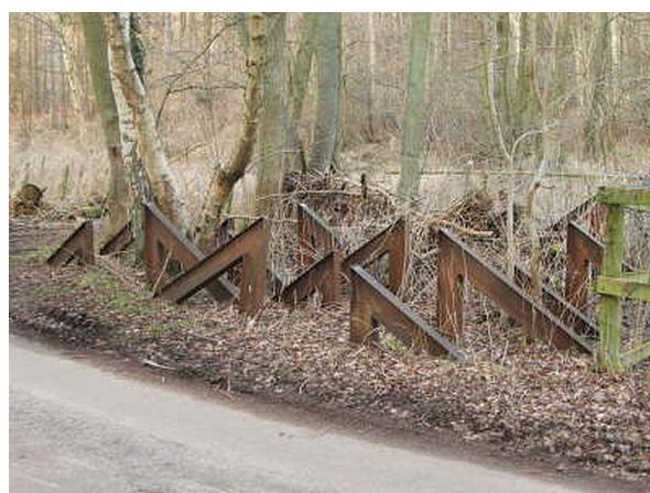
Plate 8: Welded RSG hairpins in Narborough, Norfolk (Pillboxes.co.uk 2010)
