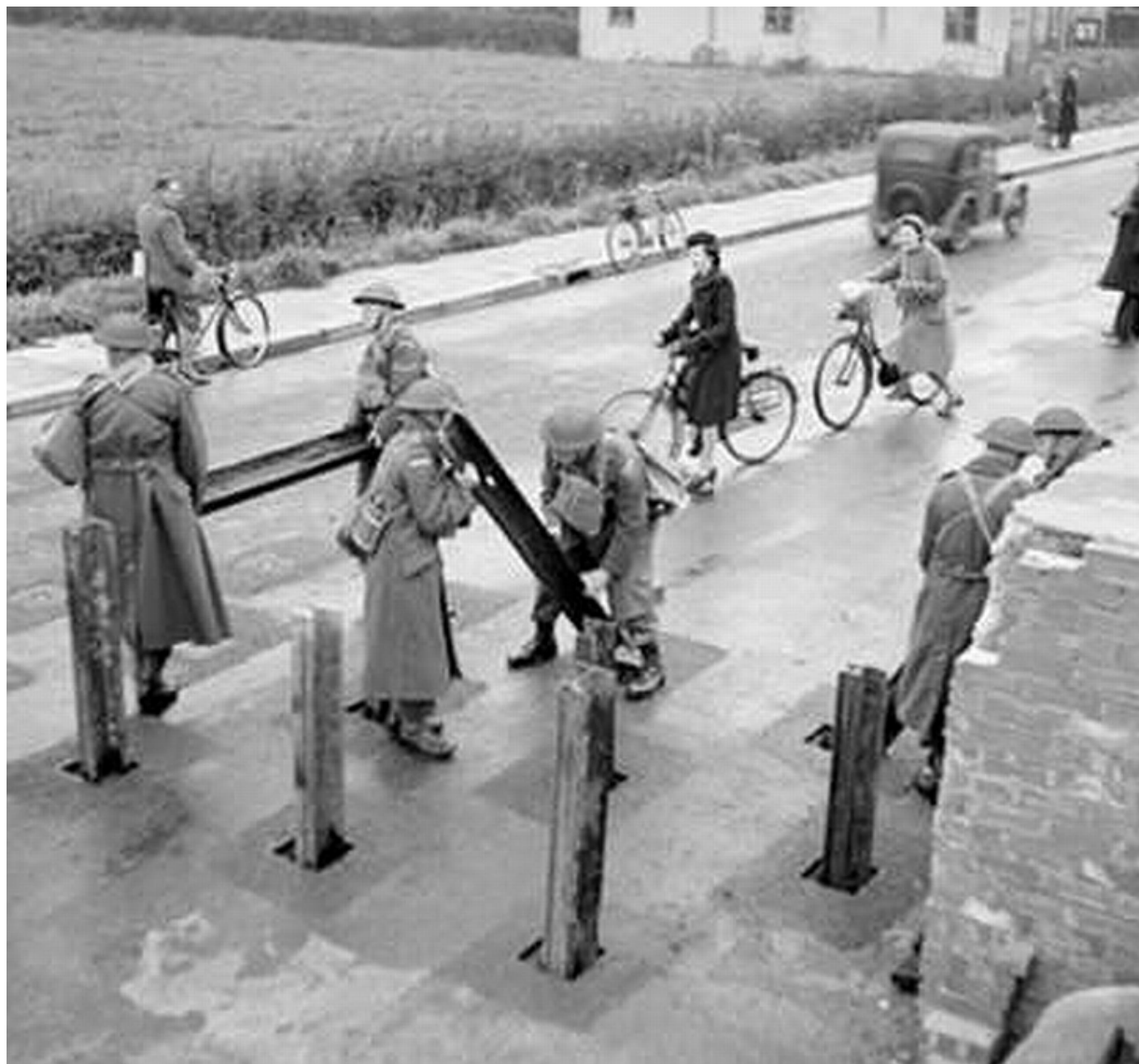
Plate 6: 'Hedgehog' or vertical rail anti-tank road block in use (Pillboxes.co.uk 2010)
