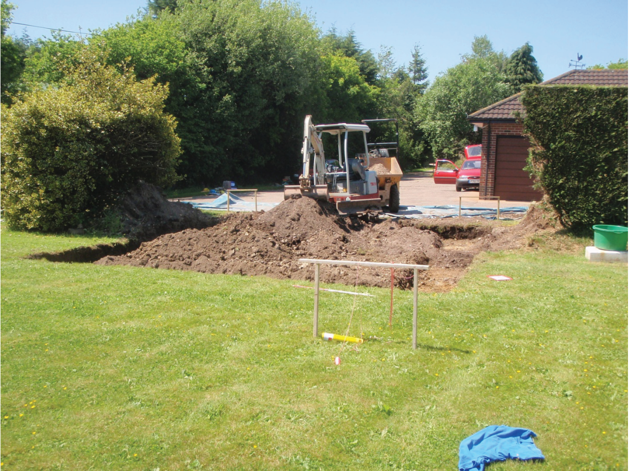
Plate 1: General shot showing the nature of the groundworks
