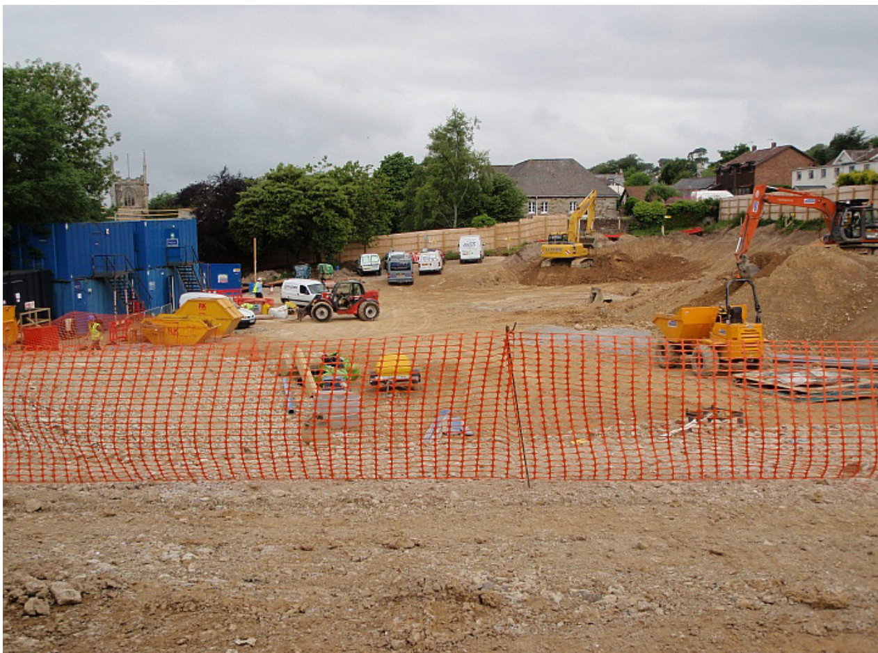
Plate 1: General shot showing ground reduction
