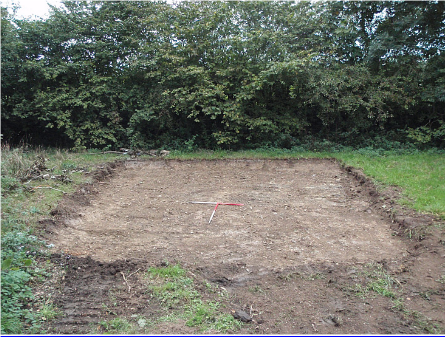
Plate 3. Stripped area for proposed location of utility block
