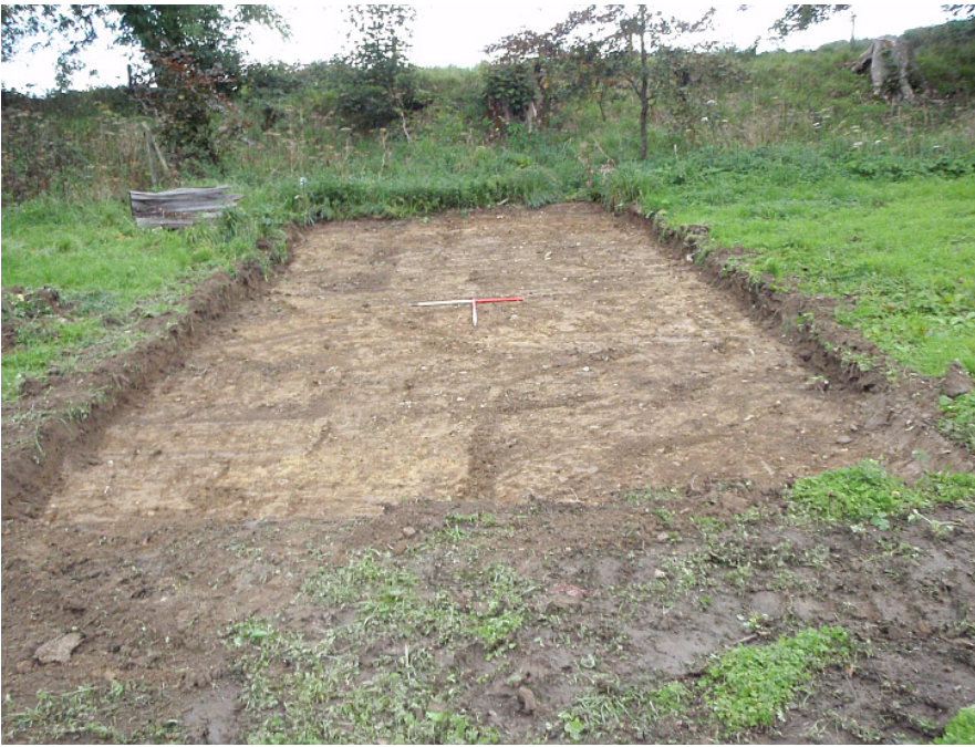
Plate 2. Stripped area for proposed location of static caravan 2
