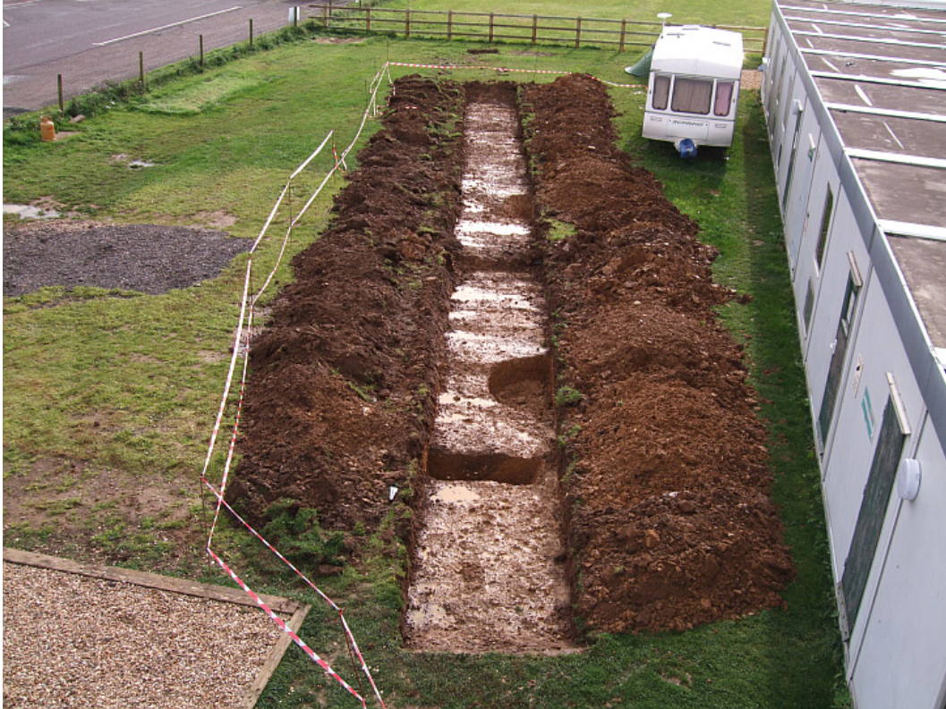
Plate 2. View of excavated pits in trench, (View from the north)
