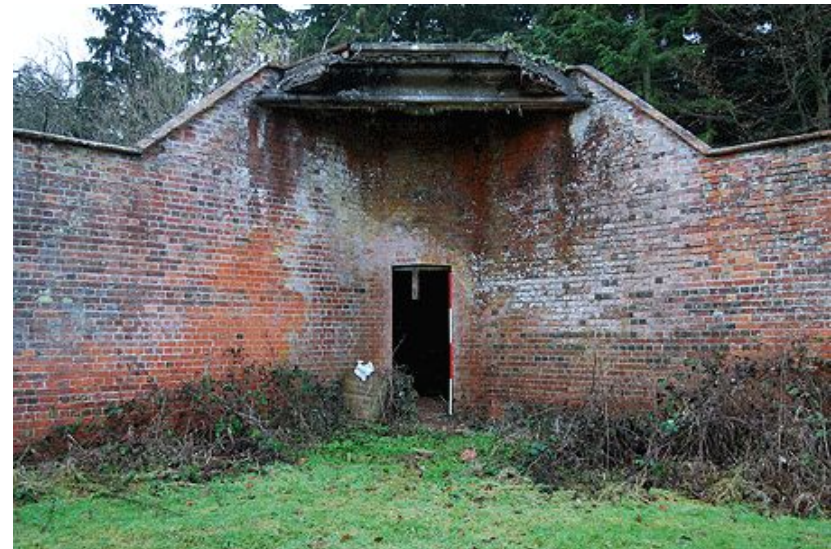
Plate 20. Observation turret from the north-east
