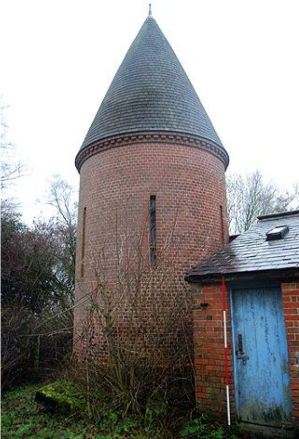
Plate 33. North-east tower from the north-west (stables)
