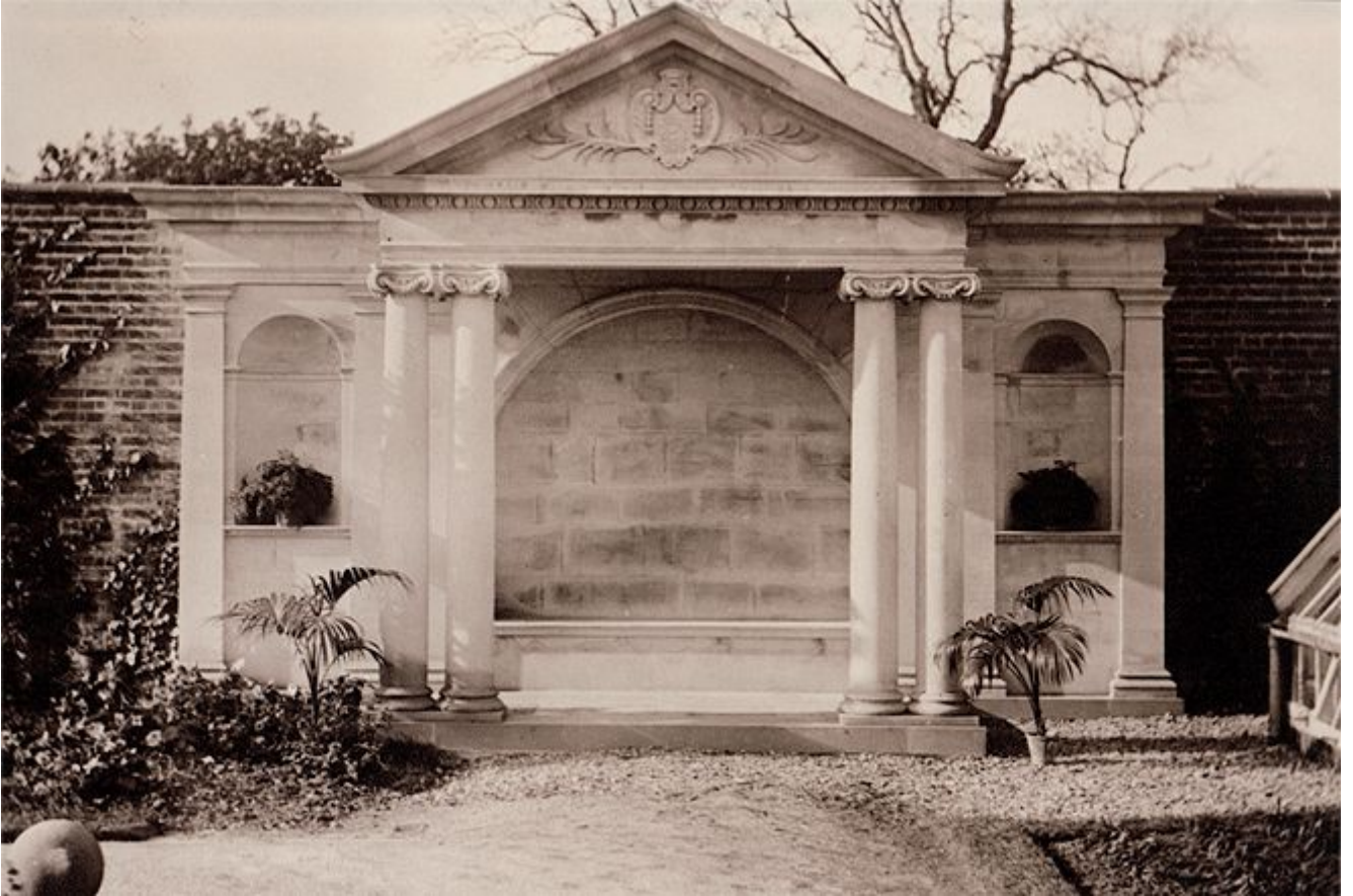
Plate 7. The summerhouse on the west wall in the early 20th century (© Rushmore Estate)
