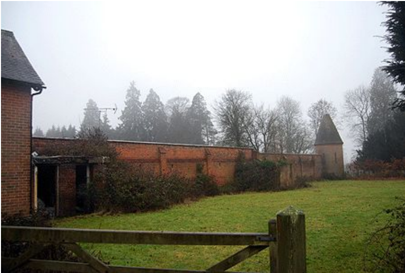
Plate 25. Outbuildings and north-west tower from the north-east
