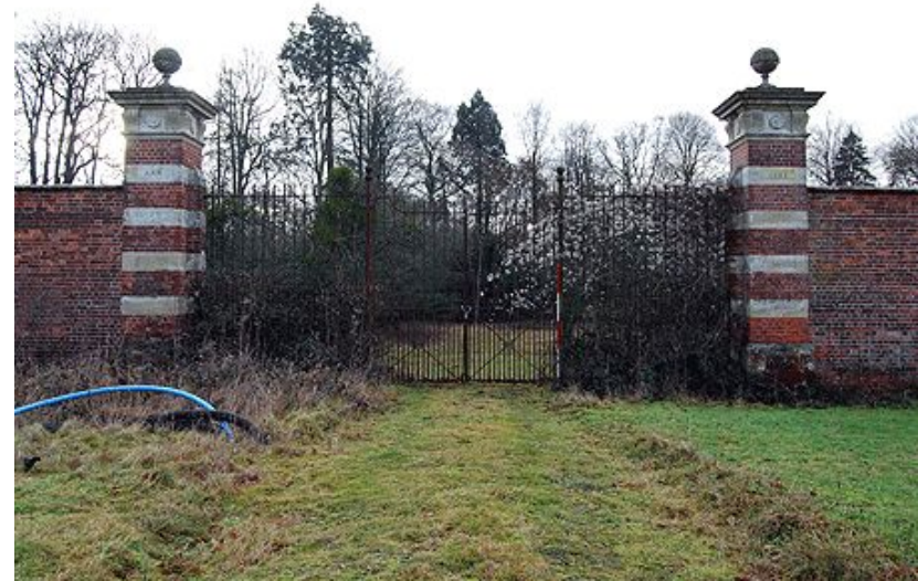
Plate 18. Southern entrance and gate piers from the north
