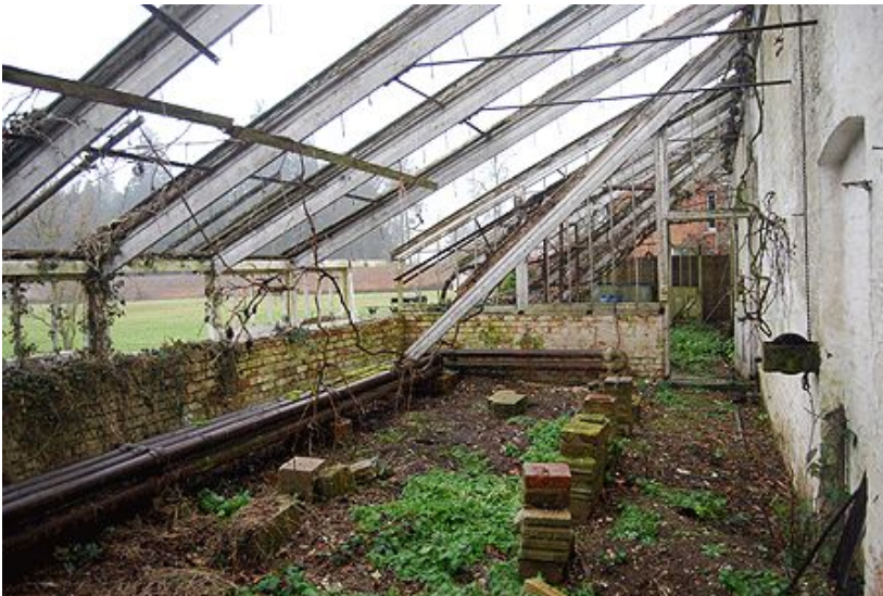
Plate 19. Interior of glasshouse from the east
