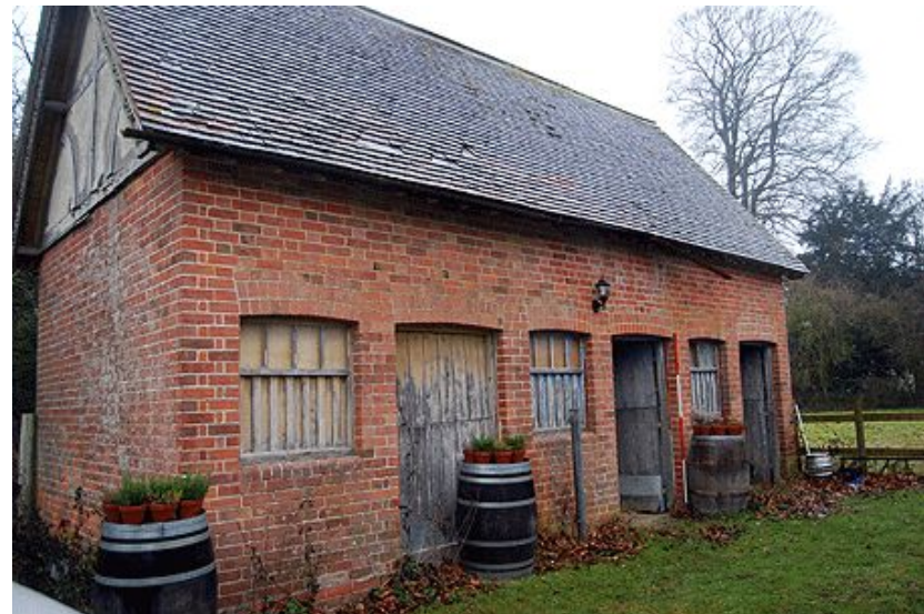
Plate 24. Stables from the south-west
