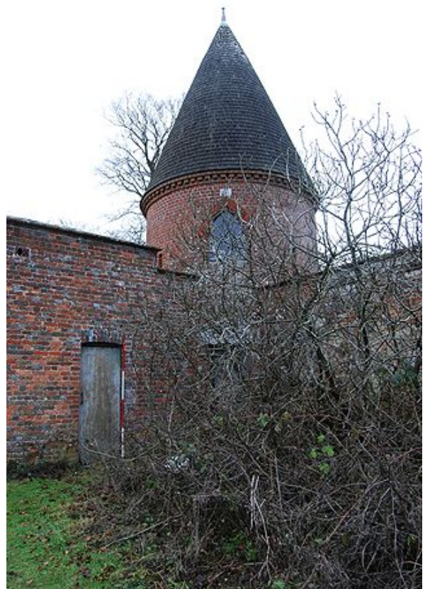
Plate 32. North-east tower from the south-west (garden)
