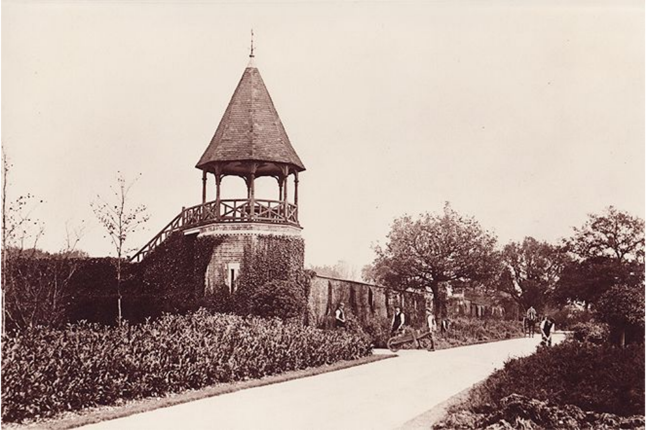
Plate 11. The observation turret in the south-west corner from the orchard in the early 20 th century (© Rushmore Estate)
