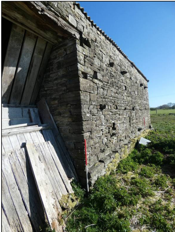
Plate 2: South elevation, east part, detail of plinth, looking E (photo 1/203).
