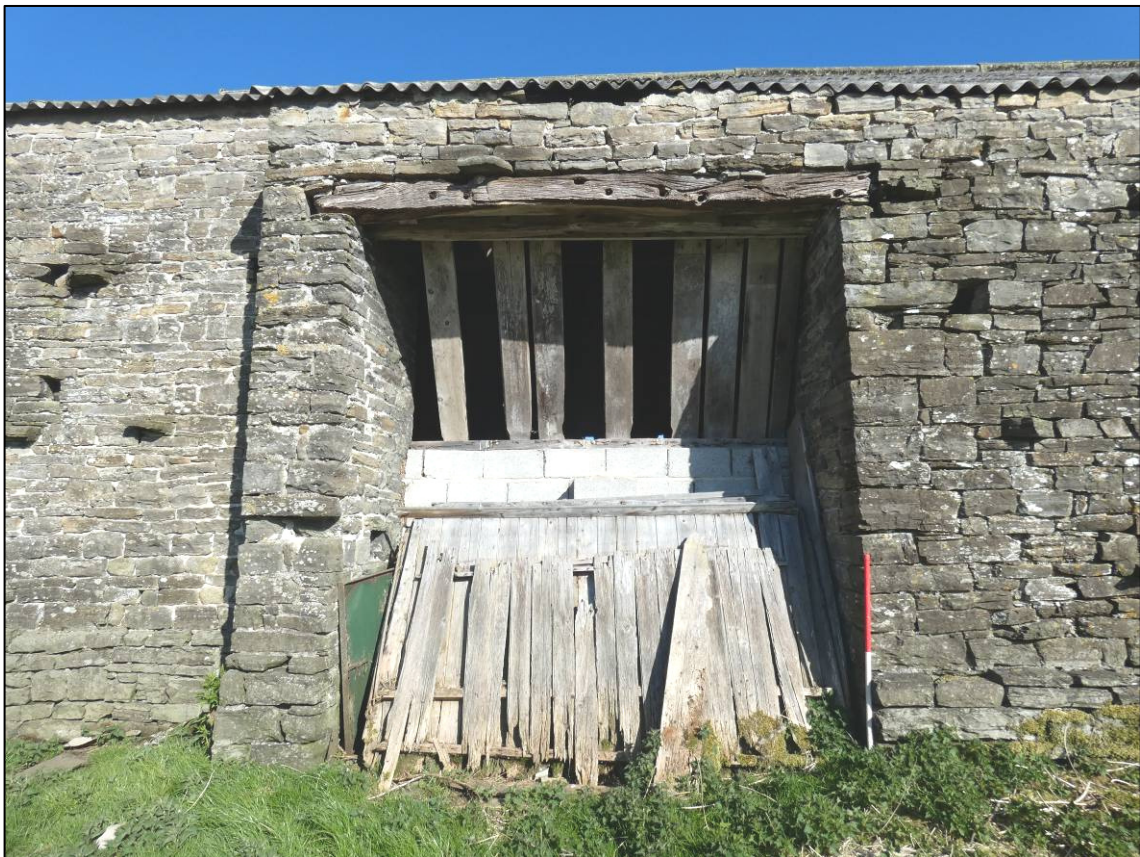
Plate 9: South elevation, cart entrance, looking N (photo 1/201).
