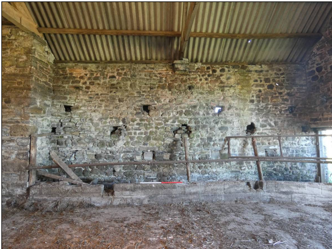
Plate 11: North internal wall, east part, looking N (photo 1/227).
