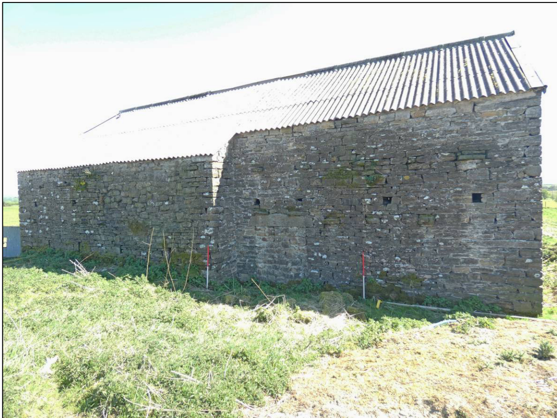
Plate 5: North elevation, looking S (photo 1/213).
