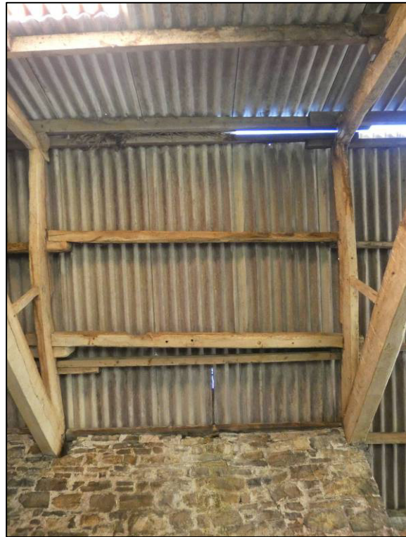
Plate 14: West central roof bay, north slope, looking N (photo 1/253).
