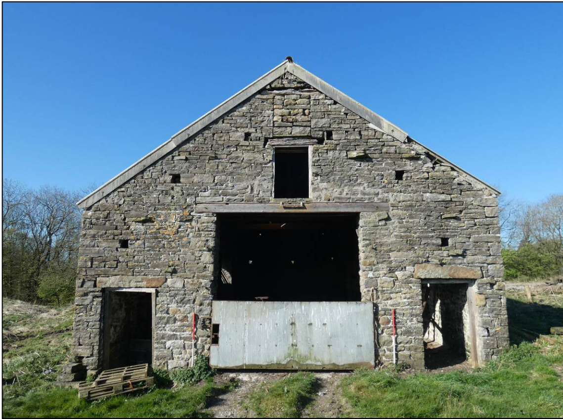
Plate 4: East gable, looking W (photo 1/190).
