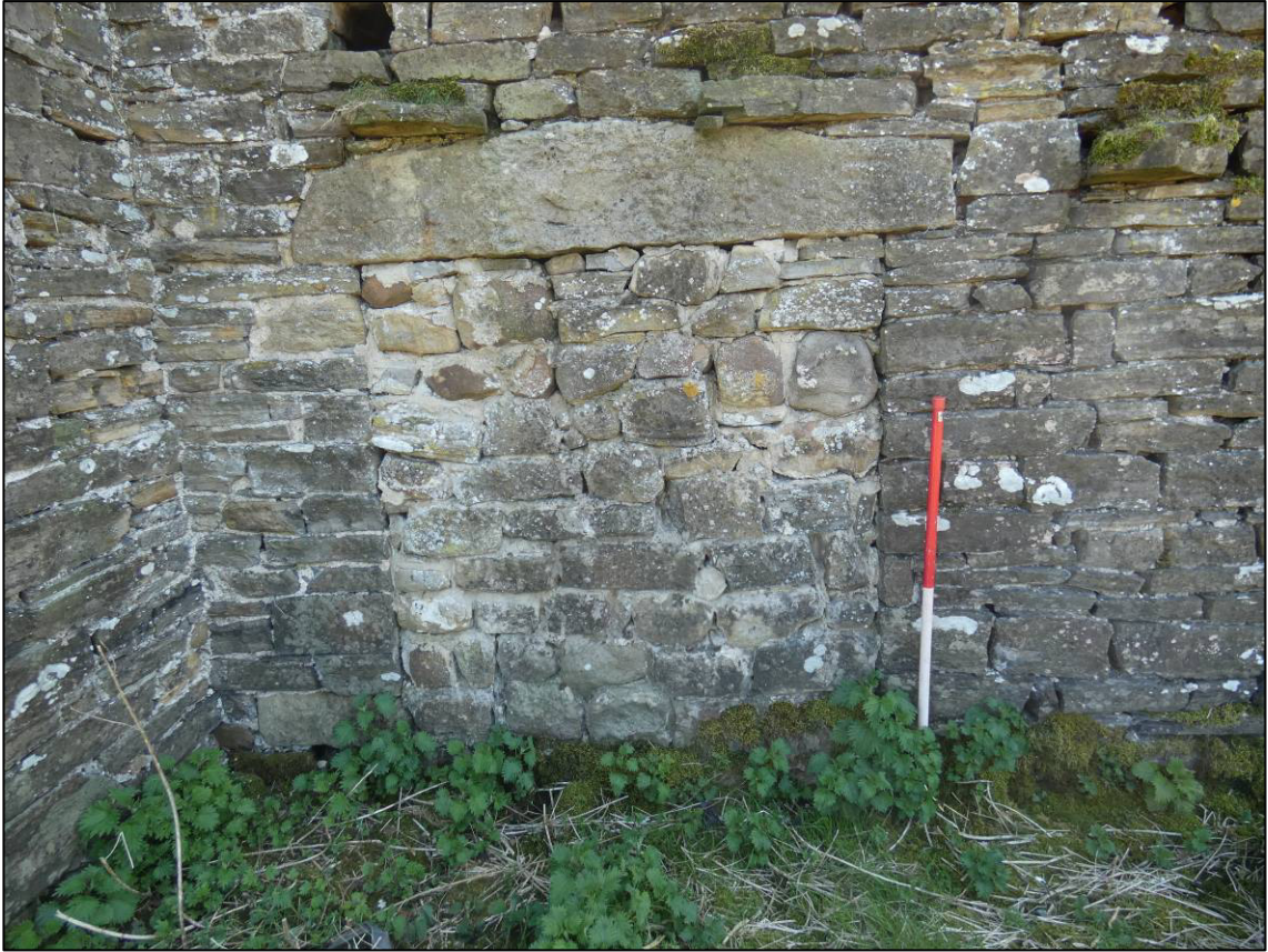
Plate 6: North elevation, west part, blocked doorway, looking S (photo 1/215).
