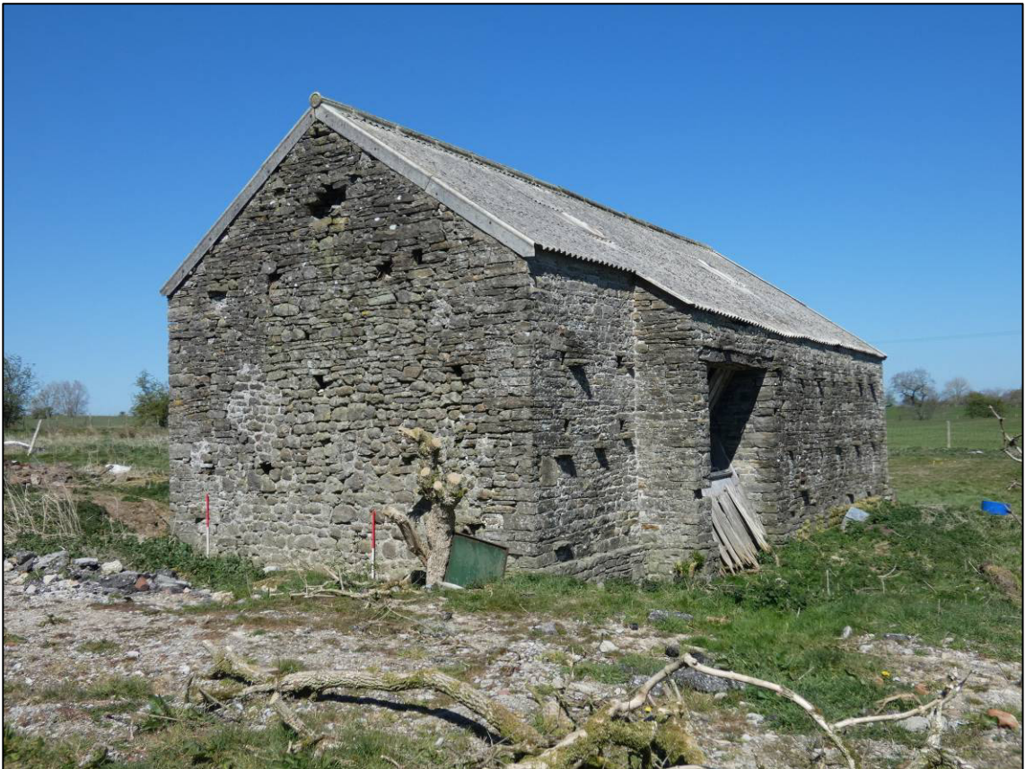
Plate 7: West gable and south elevation, looking NE (photo 1/210).
