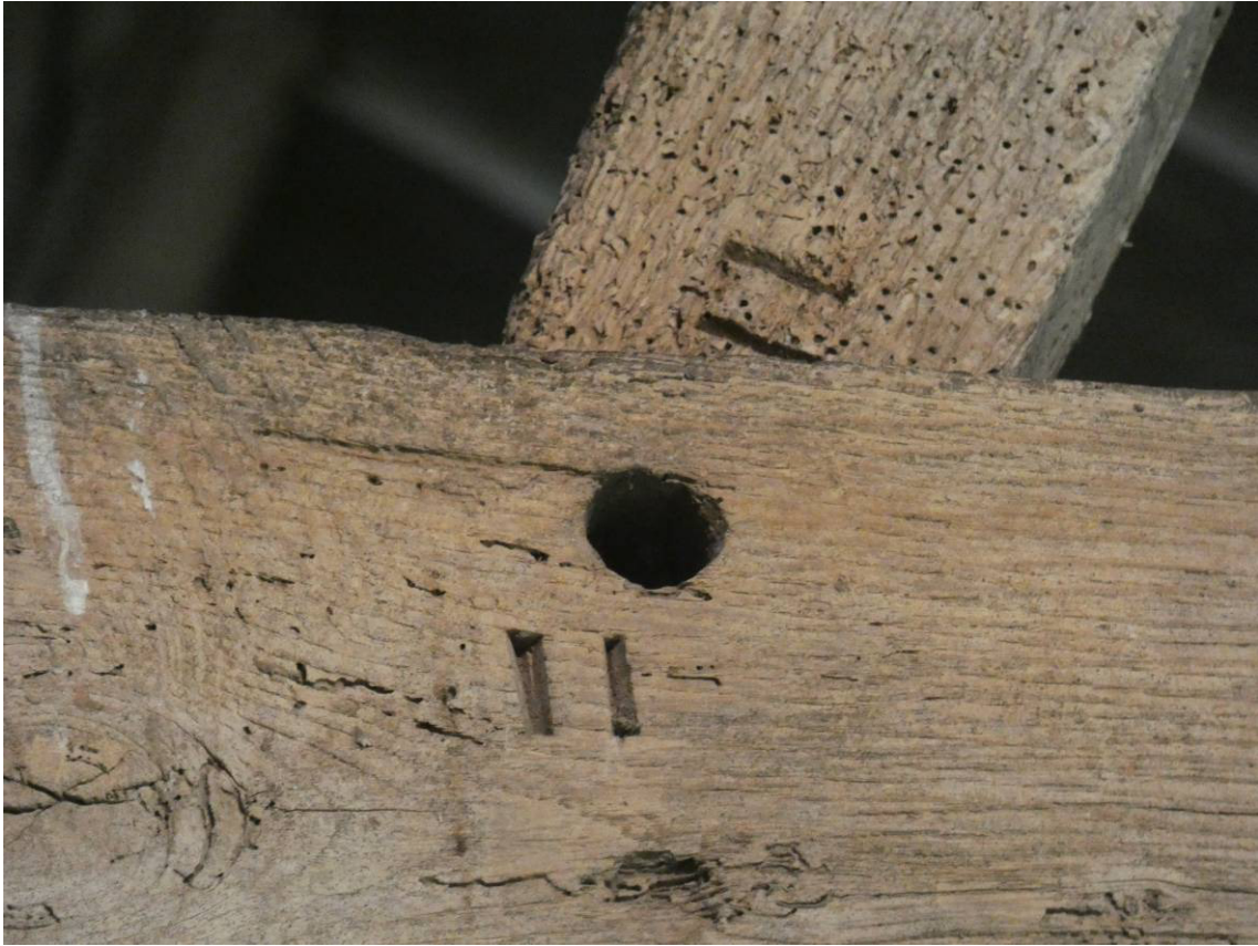
Plate 17: Central roof truss, west face, detail of numbering, looking E (photo 1/257).
