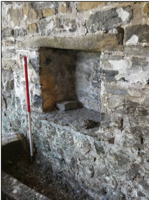
Plate 13: South internal wall, recess to east part, looking SE (photo 1/237).
