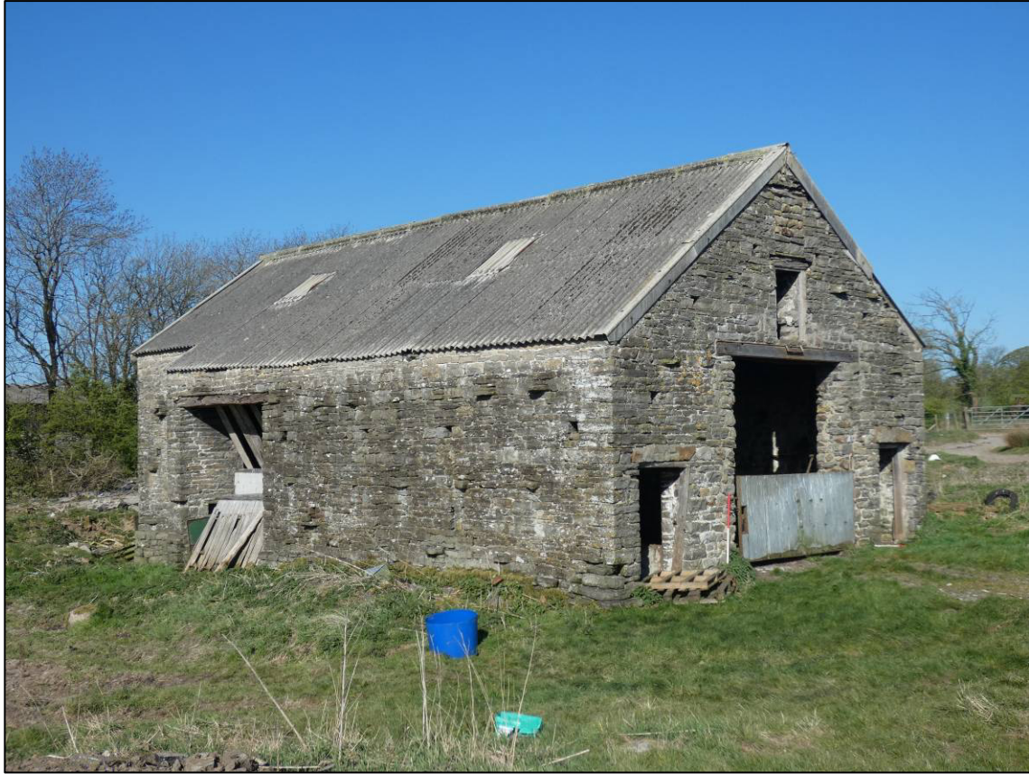
Plate 1: East gable and south elevation, looking NW (photo 1/194).
