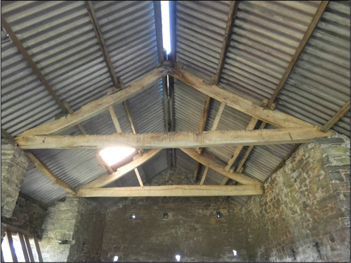
Plate 15: Central roof truss, east face, looking W (photo 1/259).
