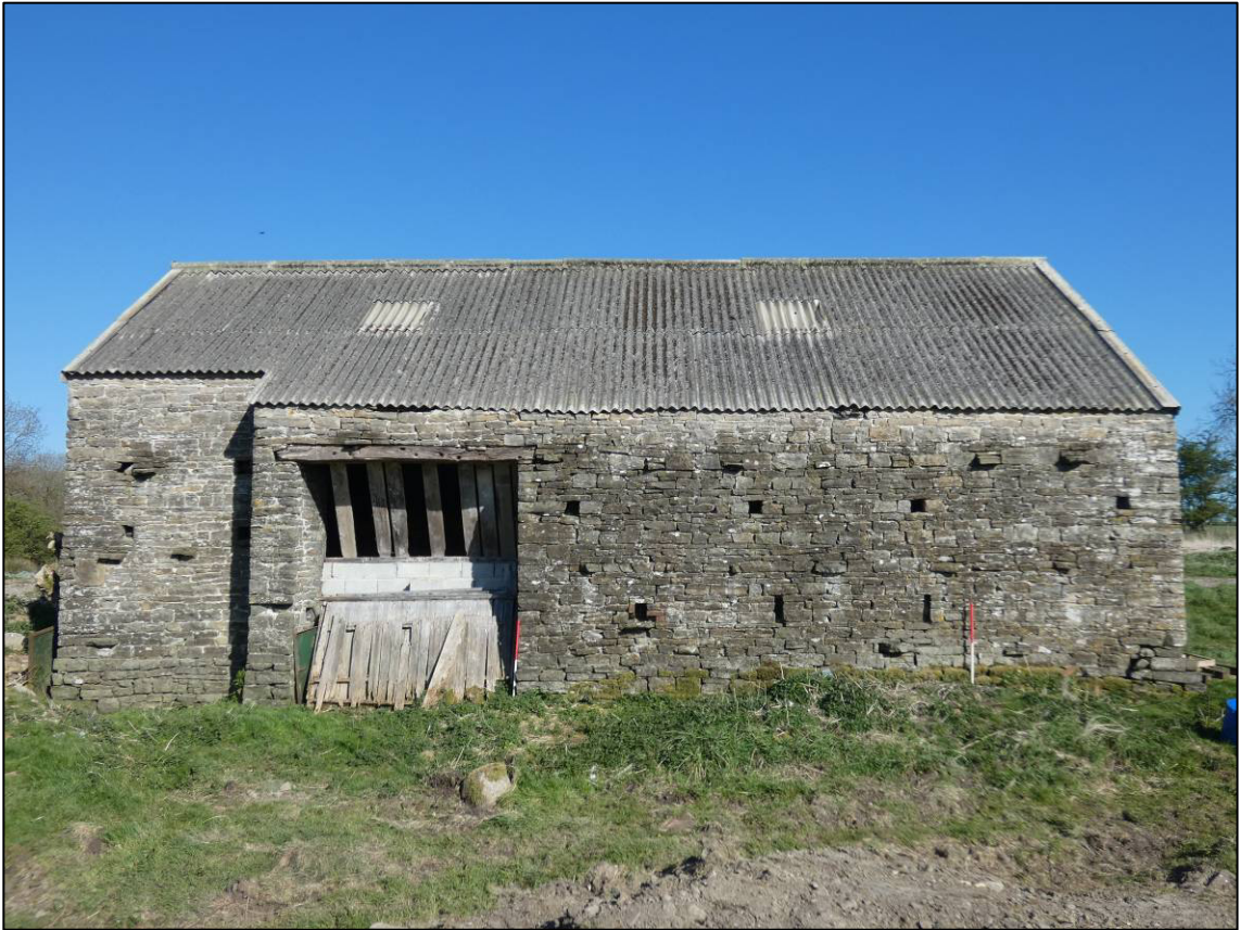
Plate 8: South elevation, looking N (photo 1/197).
