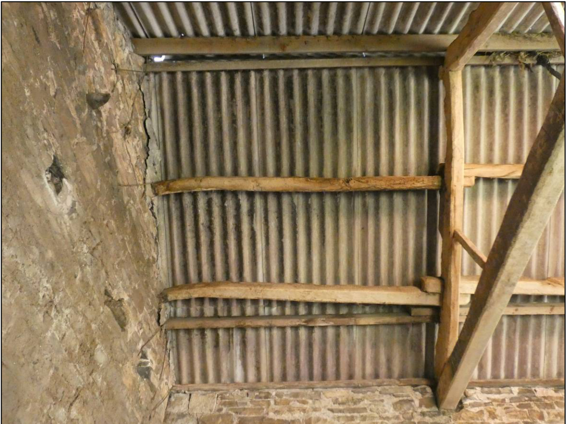
Plate 16: West roof bay, north slope, looking N (photo 1/248).
