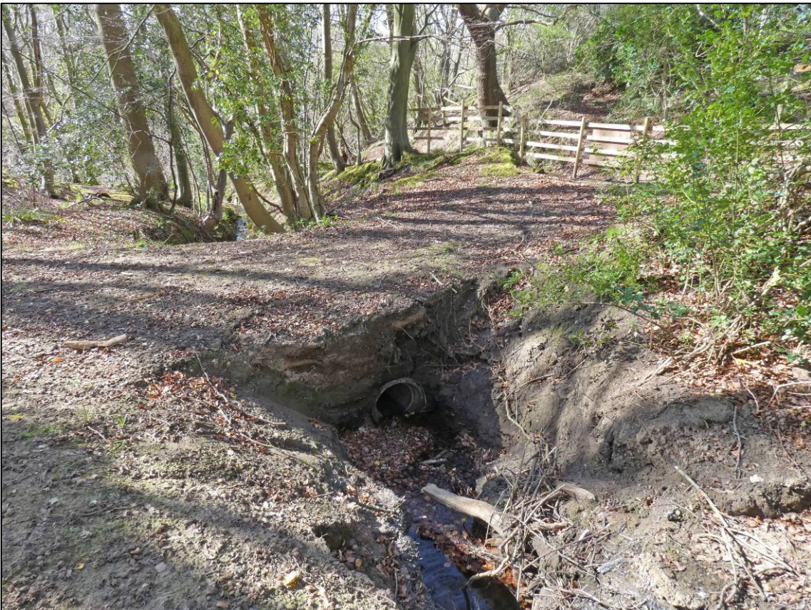
Plate 2: Bridge over tributary stream (north side), looking S (photo 1/481, April 2020).
