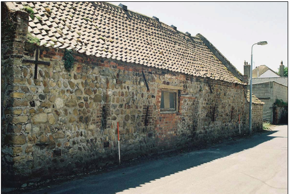
Plate 4: North elevation of barn, showing wall tie-plates, slit breathers and blocked doors, looking SW (photo 1/21).
