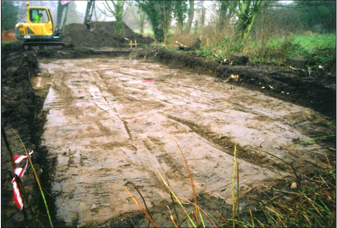
Plate 7: Stripped main construction area, looking NW.
