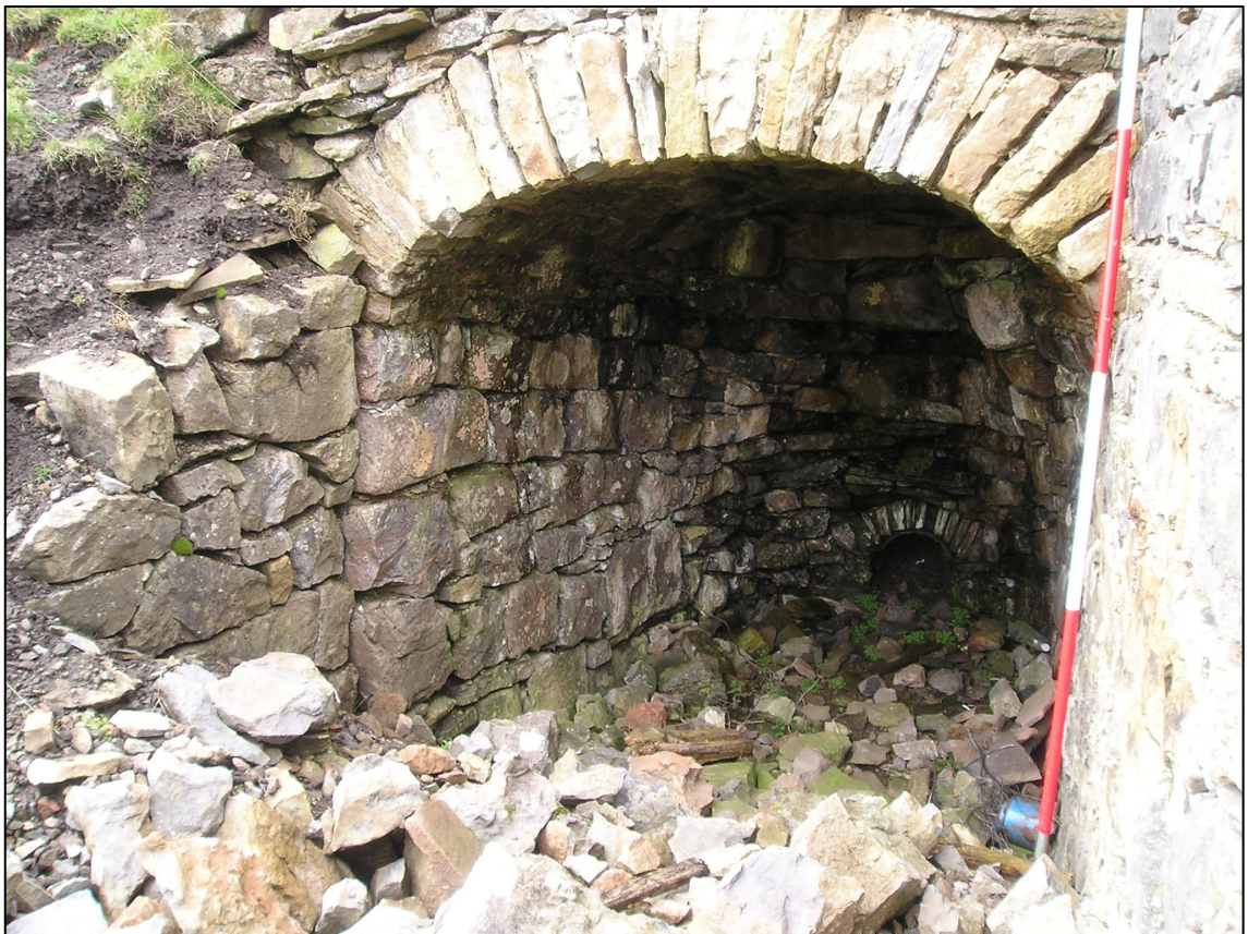
Plate 6: Draw-hole arch and interior of lime kiln (Site 9), before consolidation, looking NW.
