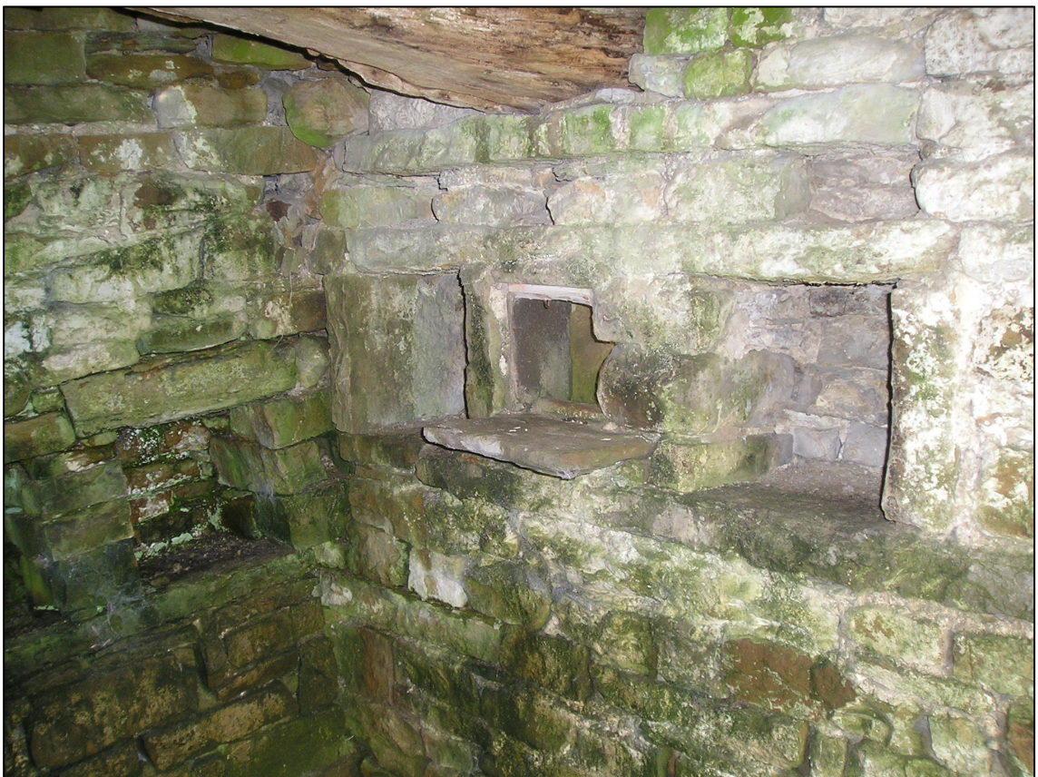
Plate 8: Internal east wall of hen house (Site 28) showing recesses and pop-hole, looking NE.
