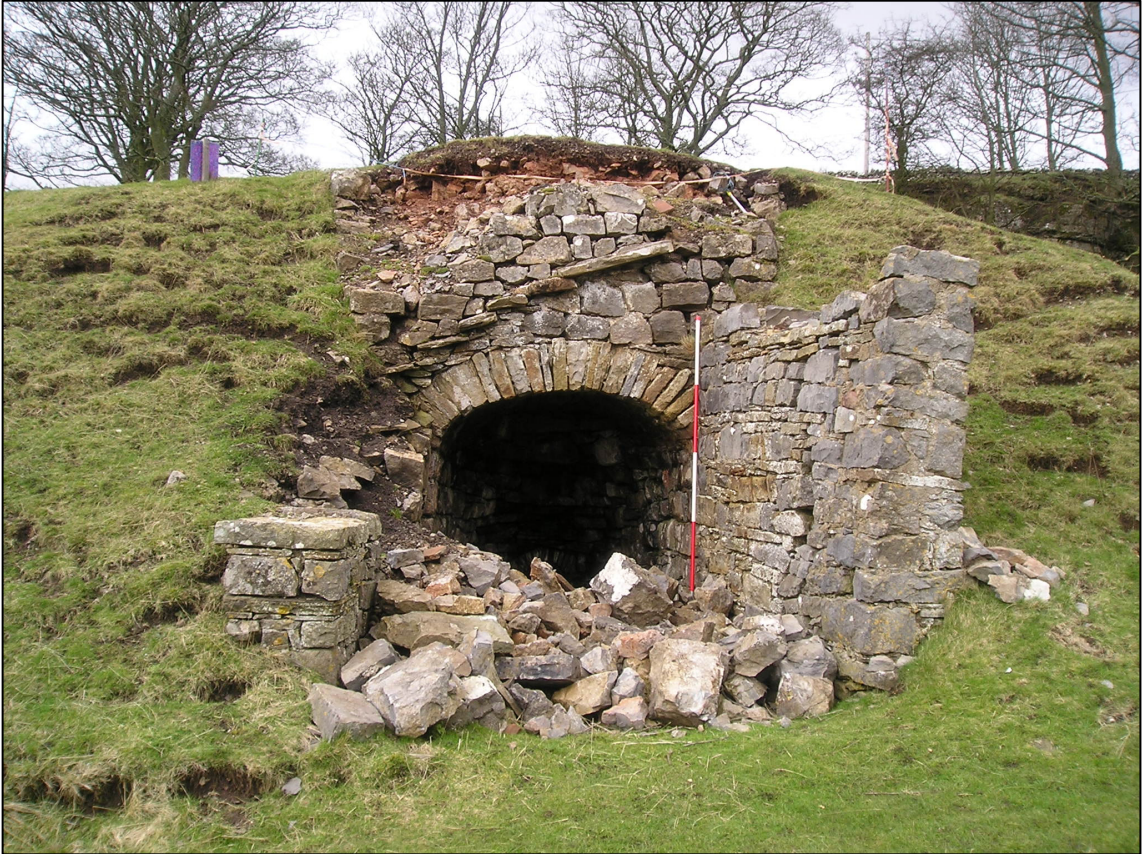
Plate 5: Lime kiln (Site 9), before consolidation, looking N.
