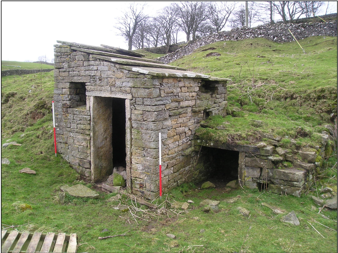
Plate 7: General view of hen house and attached structure (Site 28), looking NW.
