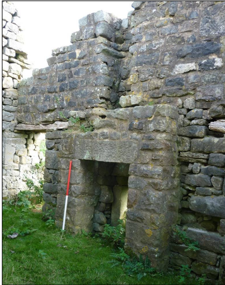
Plate 3: Fireplace, east wall of west cell, looking NE (photo 1/18).
