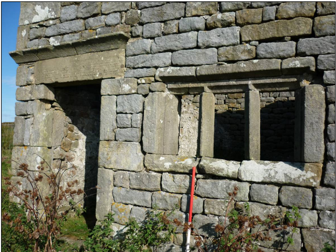
Plate 2: Doorway and west window, south elevation, looking NW (photo 1/03).
