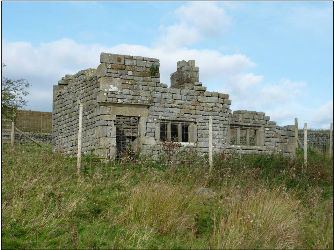
Plate 1: General view of house, looking NE (photo 1/41).
