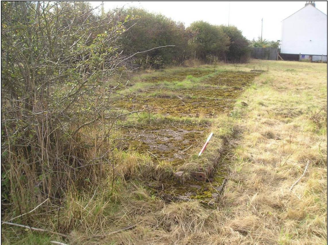
Plate 12: Second World War hut base (part of Site 22), looking E.
