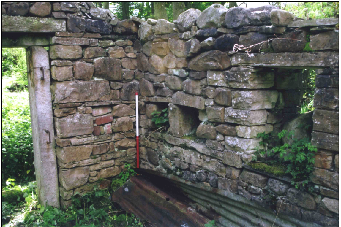
Plate 4: Internal south-west corner of hen house, looking SW.
