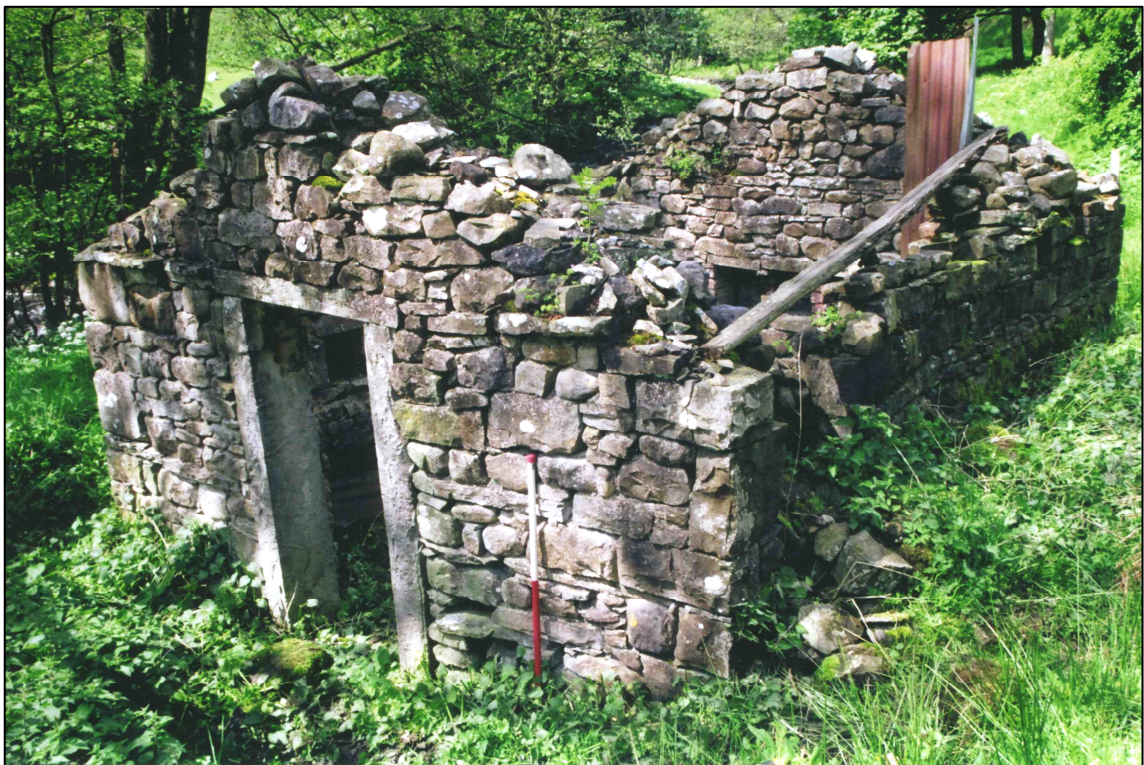
Plate 2: South elevation of hen house, looking NW.
