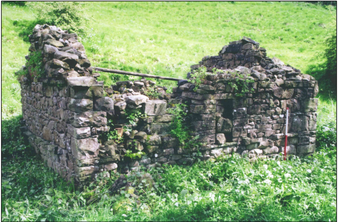
Plate 1: West elevation of hen house, looking E.
