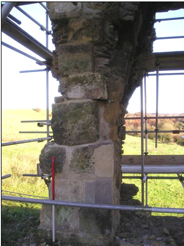
Plate 13: Repairs to north side of first floor fireplace.
