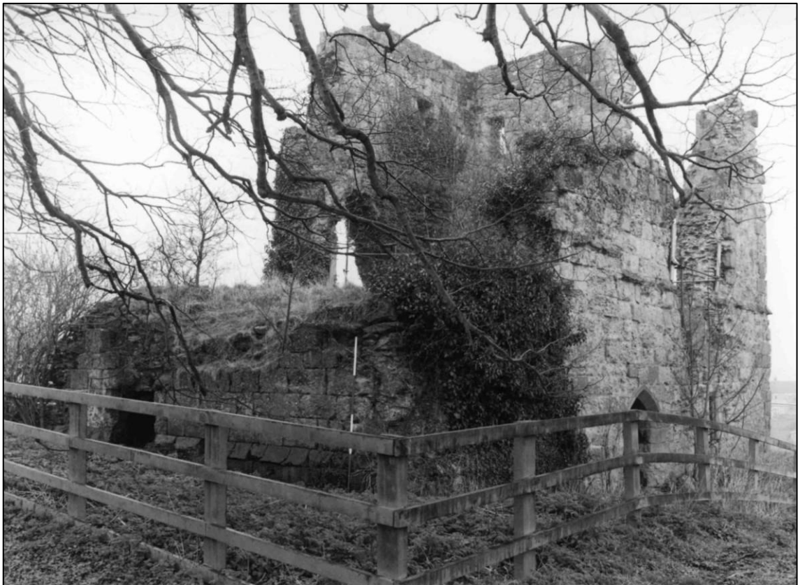
Plate 5: Ayton Castle looking east, prior to 2006 repairs.
