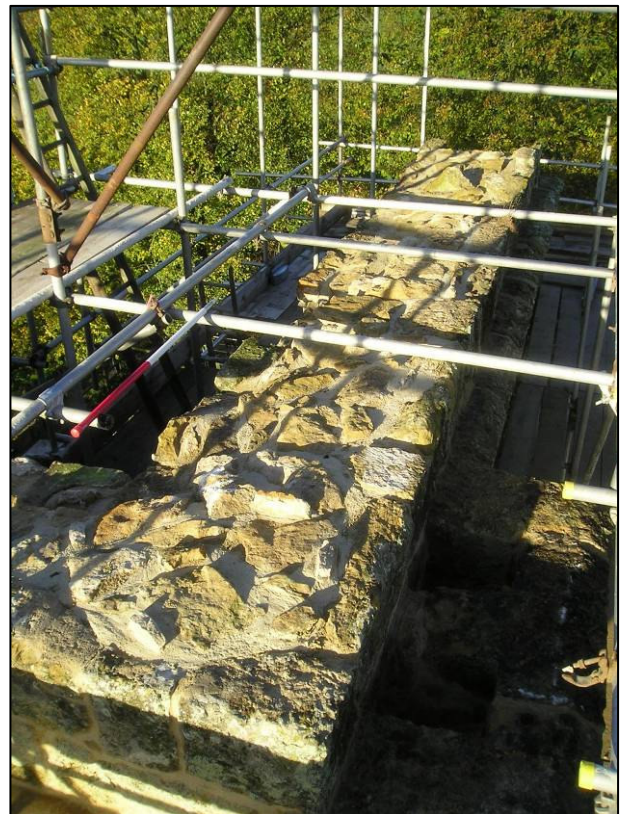
Plate 14: Repairs to wall tops.
