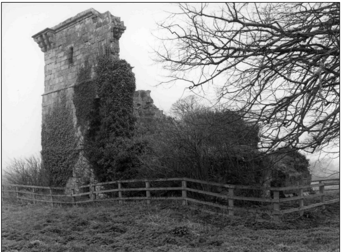
Plate 6: Ayton Castle looking south, prior to 2006 repairs.
