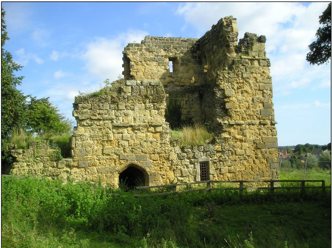
Plate 2: Ayton Castle, west elevation, looking north-east.
