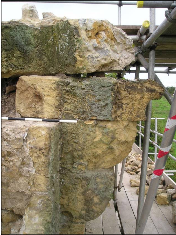
Plate 11: Detail of corbels and machicolations, prior to repair.
