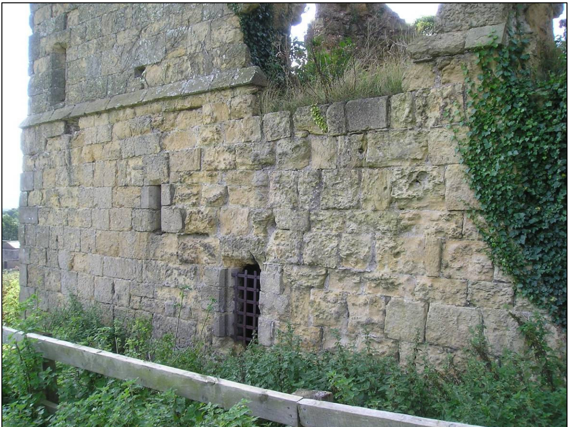
Plate 10: Lower part of east elevation, looking south.
