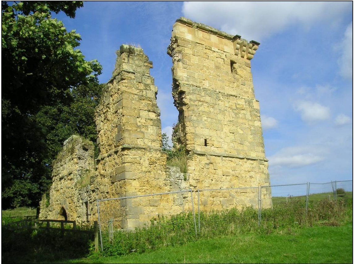
Plate 15: Completed Phase 1 repairs, south elevation, looking north.
