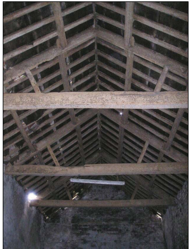
Plate 10: Roof trusses in barn, looking S (photo 3/25).
