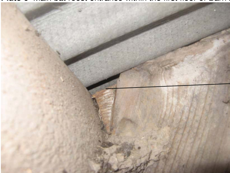
Plate 6 Main bat roost entrance within the first floor of Barn A
