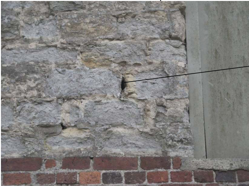
Plate 2 Crevices for bat access into a potential bat roosts within the stone wall of Barn A (northern elevation)
