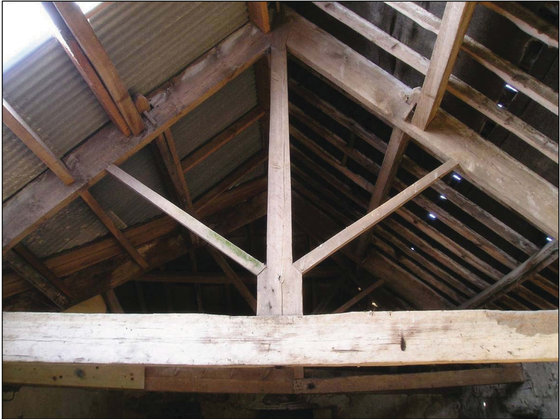
Plate 3: Typical roof truss in cart shed, looking W (photo 3/57).
