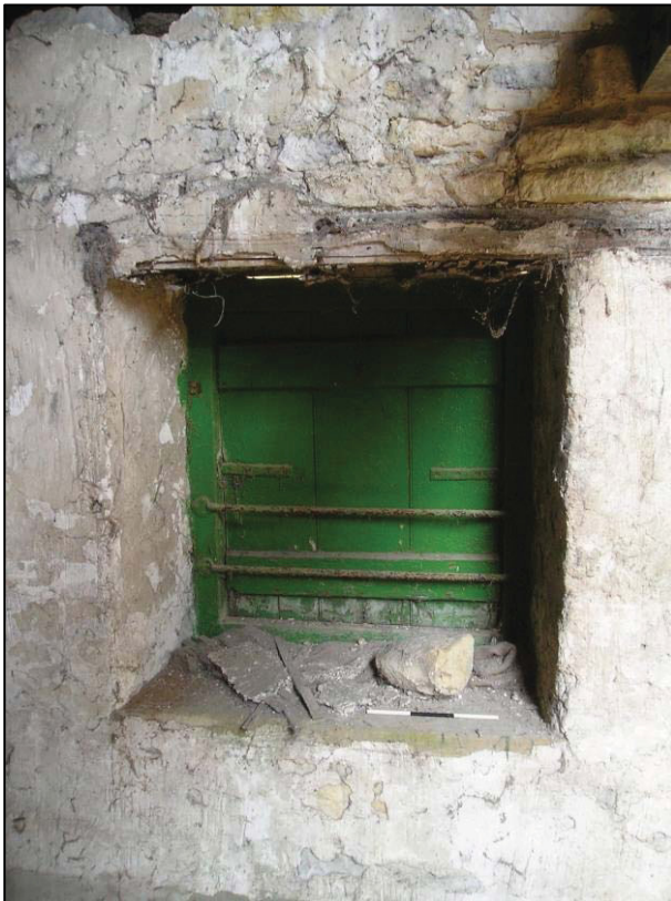
Plate 4: Internal detail of typical window, first floor of cart shed (photo 3/49).
