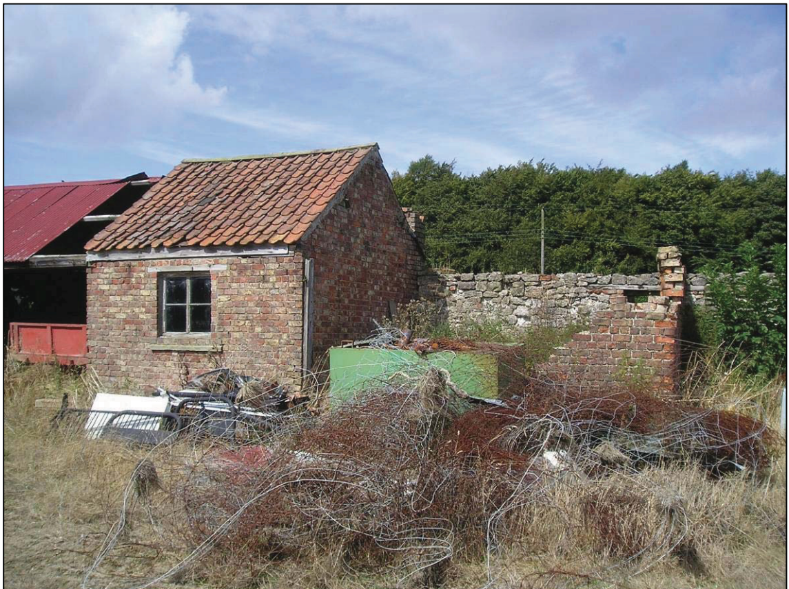
Plate 12: Wold Ranger's house (roofed), looking N (photo 3/117).
