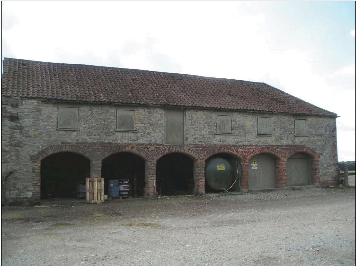
Plate 1: North elevation of cart shed, looking SW (photo 3/89).
