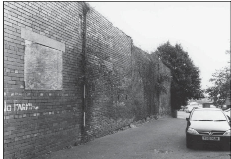
Plate 4: W side of range, Building A in foreground, looking SE (photo 1/13).
