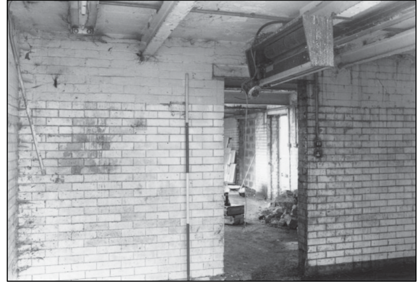
Plate 26: Building A, S part of GF, looking N (photo 9/5).
