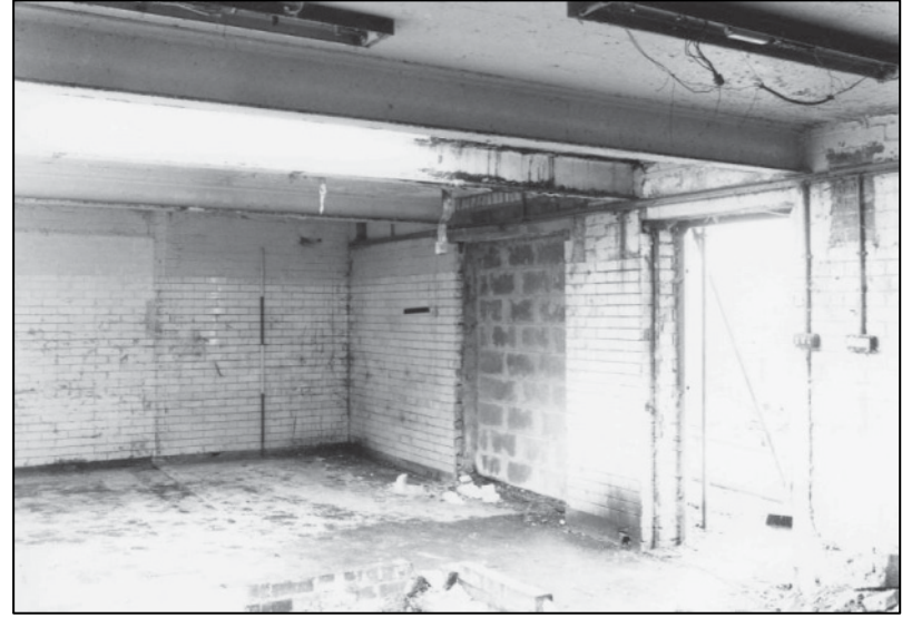
Plate 18: Building A, N part of GF, looking N (photo 10/6).
