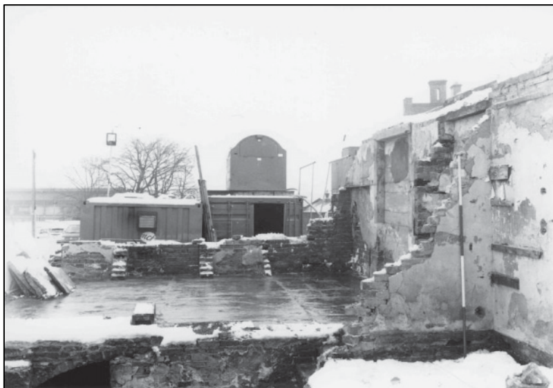
Plate 115: Building D, S GF room after partial demolition, looking SE (photo 6/13).
