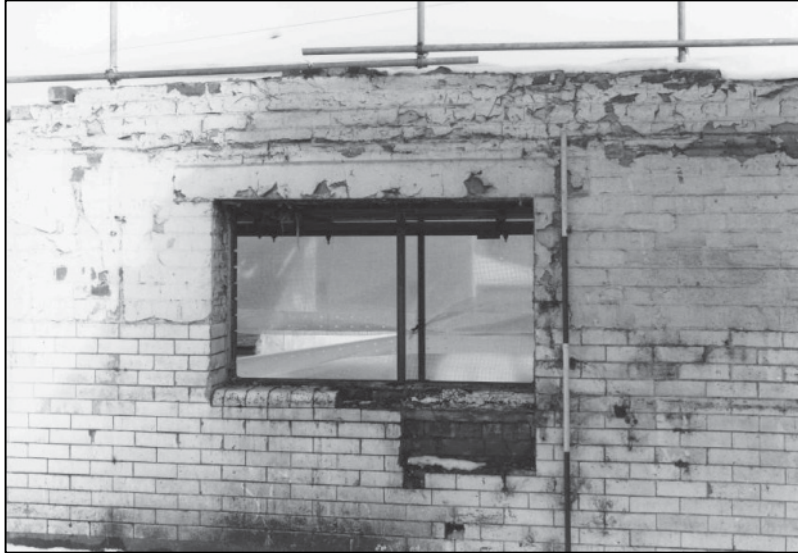
Plate 37: Building A, 1F, showing typical window, looking E (photo 8/18).
