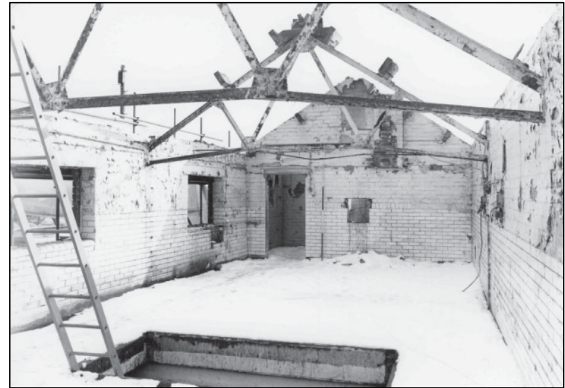
Plate 36: Building A, 1F, looking S (photo 8/16).
