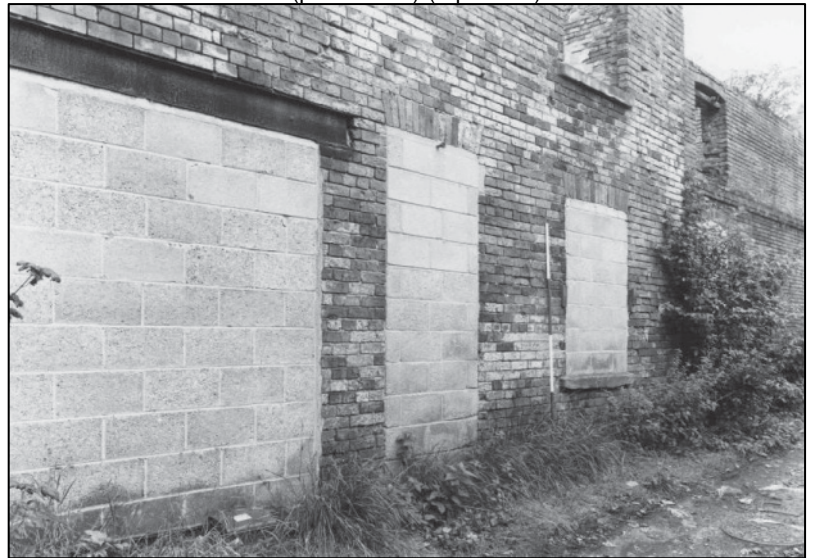
Plate 96: Building D, GF E elevation, looking W (photo 1/15).
