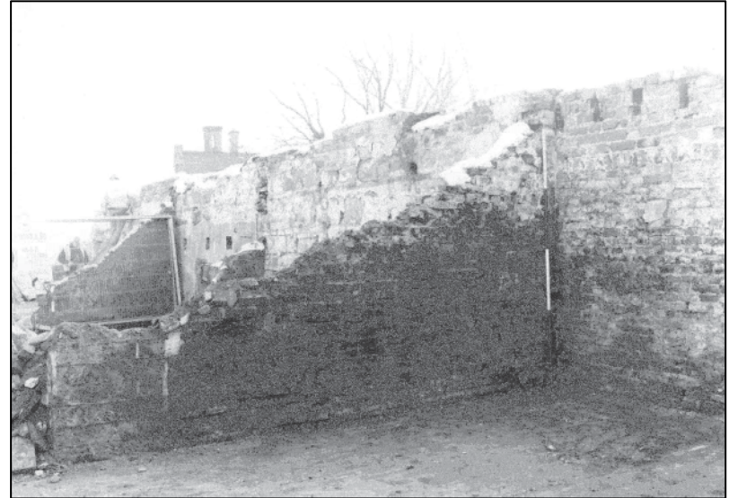
Plate 54: Building B, GF after partial demolition, looking S (photo 10/12).
