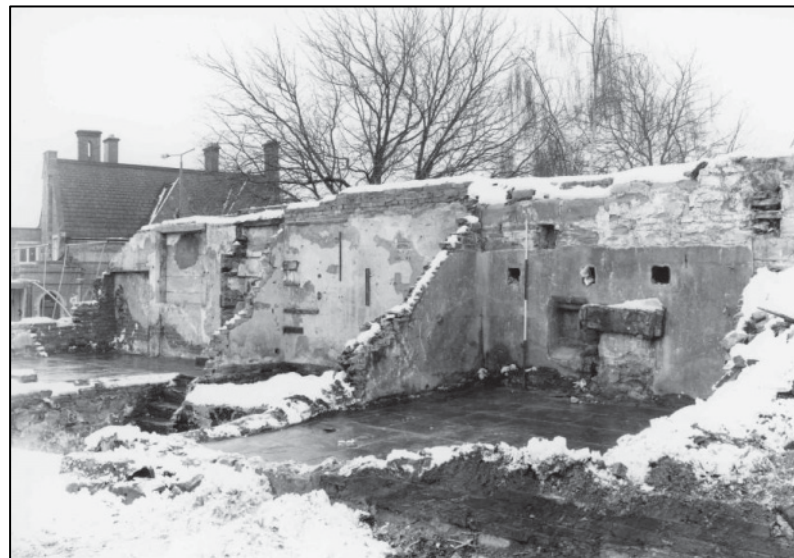
Plate 114: Buildings C & D, GF after partial demolition, looking S (photo 6/2).
