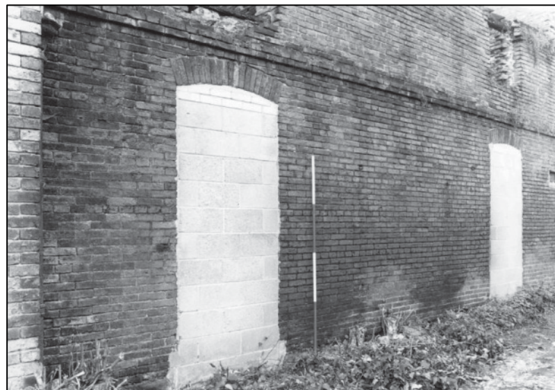
Plate 64: Building C, E elevation, looking NW (photo 3/2).
