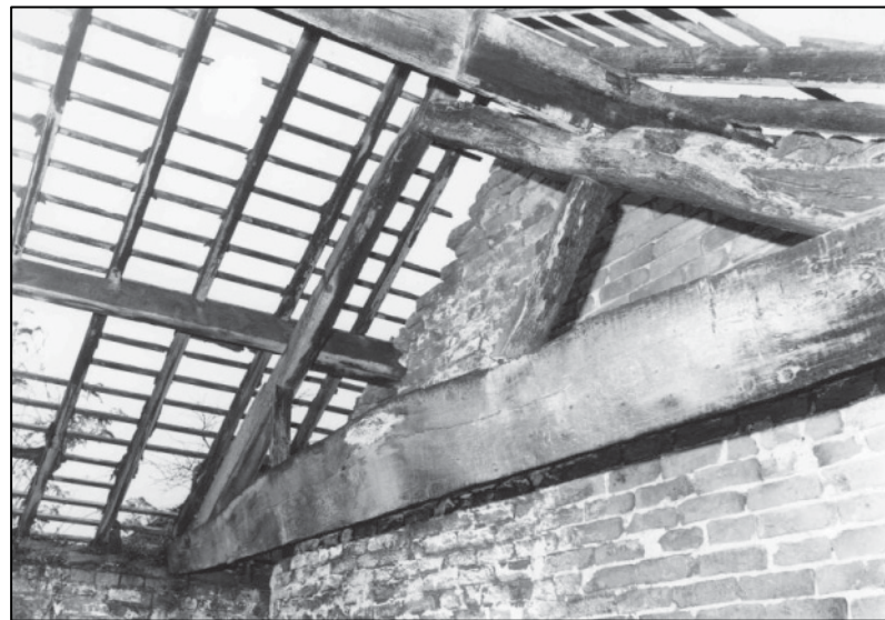
Plate 90: Building C, roof truss, S 1F room, looking NW (photo 4/11).
