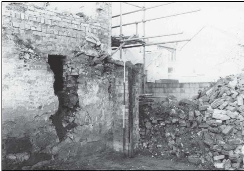
Plate 47: Building B, GF after partial demolition, looking N (photo 10/11).
