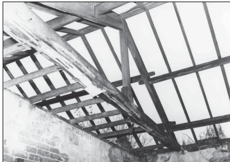
Plate 124: Building D, roof truss, N 1F room, looking SW (photo 5/3).
