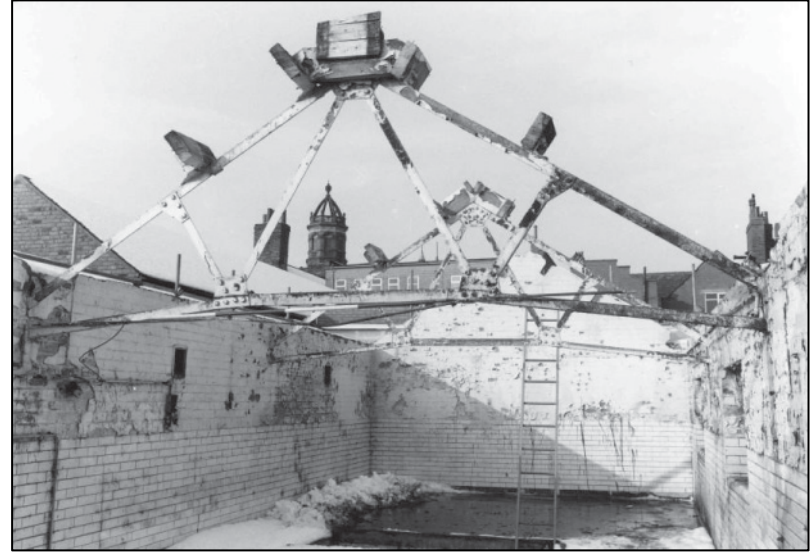
Plate 38: Building A, 1F showing typical roof truss, looking N (photo 8/7).
