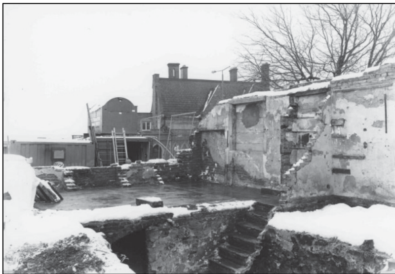
Plate 113: Building D, GF after partial demolition, looking S (photo 6/1).
