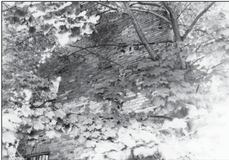
Plate 95: Building D, S gable, looking NW (photo 3/8).
