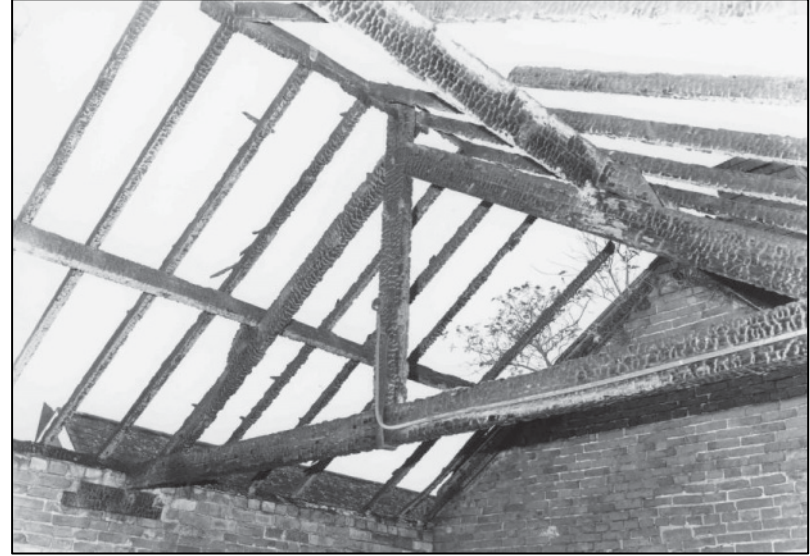
Plate 58: Building B, roof truss over 1F room, looking NW (photo 4/2).
