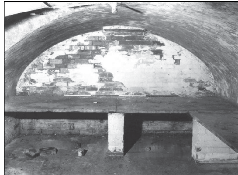
Plate 16: Building A, cellar, looking SE (photo 7/10).
