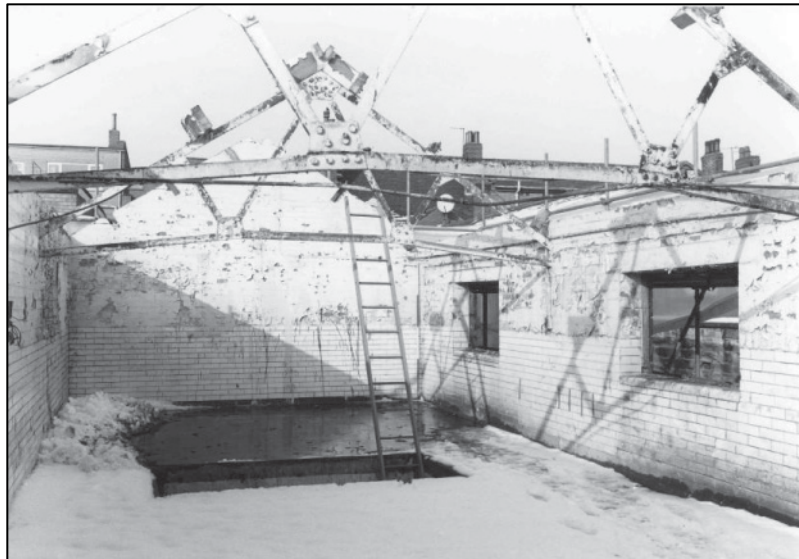
Plate 39: Building A, 1F, looking NE (photo 8/10).
