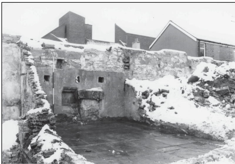
Plate 79: Building C, S GF room after partial demolition, looking W (photo 6/5).
