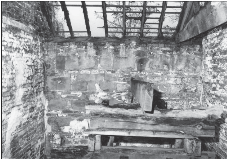
Plate 87: Building C, S 1F room, looking W (photo 4/16).
