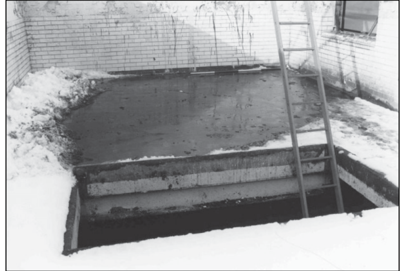
Plate 30: Building A, 1F, former stair position, looking N (photo 8/14).
