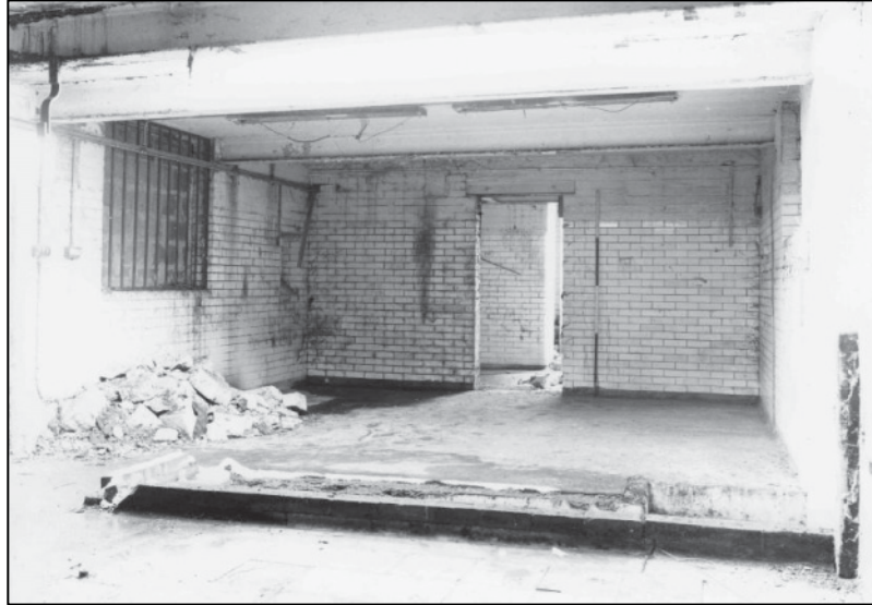
Plate 17: Building A, N part of GF, looking SE (photo 10/2).
