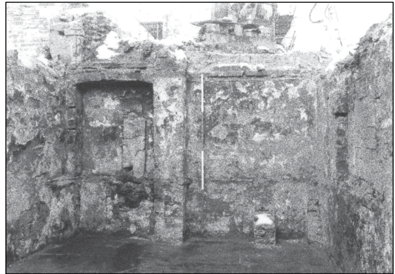
Plate 112: Building D, N wall of N cellar space, looking NW (photo 7/7).
