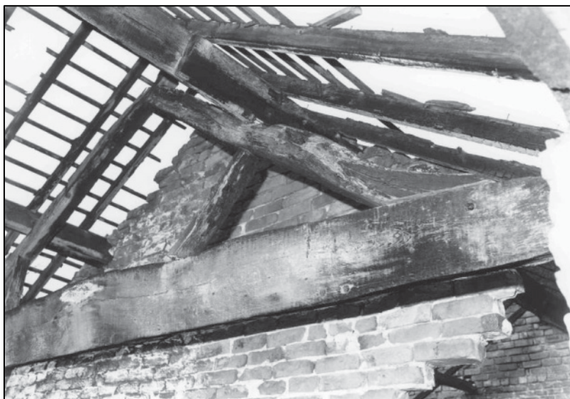
Plate 91: Building C, roof truss, S 1F room, looking NW (photo 4/12).
