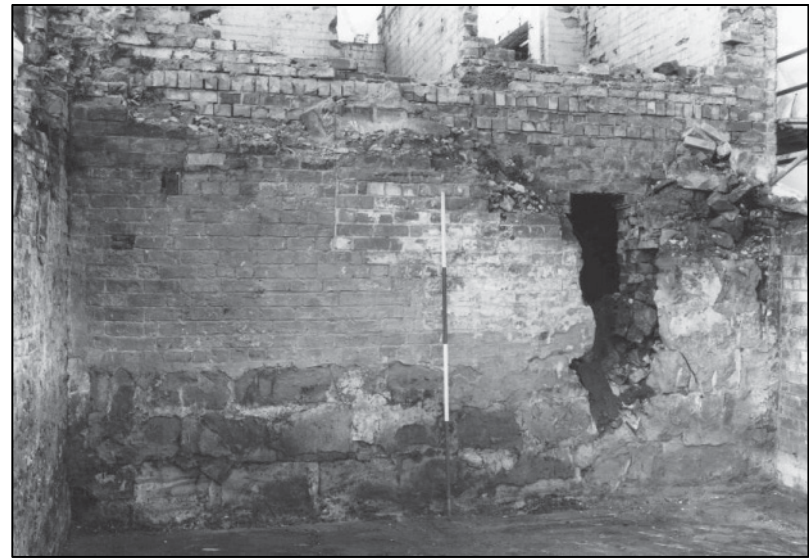
Plate 48: Building B, GF after partial demolition, looking NW (photo 10/10).
