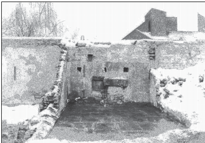
Plate 83: Building C, S GF room after partial demolition, looking SW (photo 6/4).
