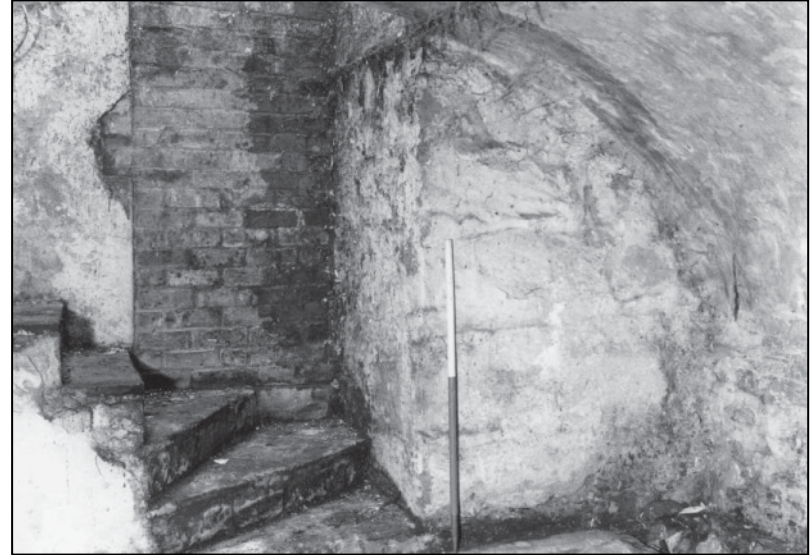
Plate 14: Building A, cellar, looking NW (photo 7/12).
