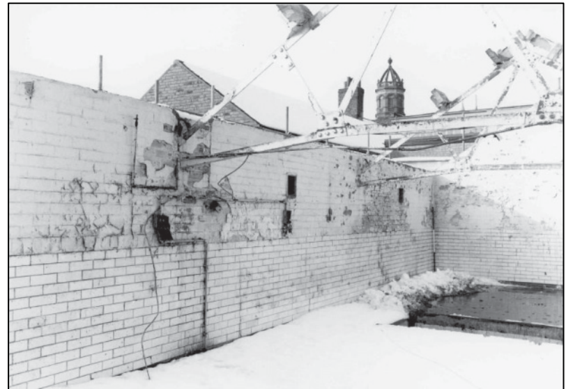
Plate 40: Building A, 1F, looking NW (photo 8/12).
