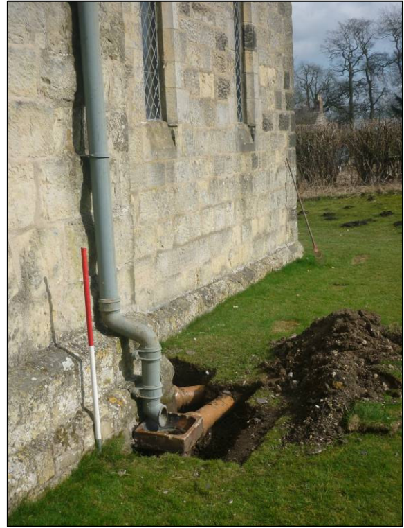
Plate 2: General view of Gullies 4/5, looking E.
