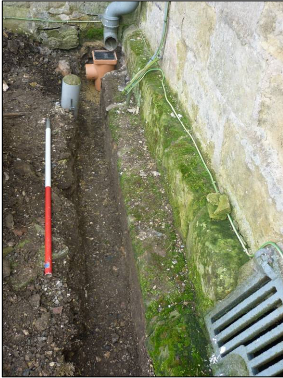
Plate 1: Gully 1 adjacent to church showing stepped plinth, looking E.
