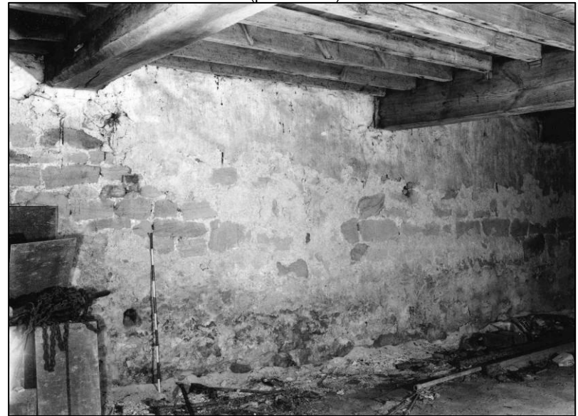
Plate 32: Recesses for cow stalls, E face of ground floor spine wall, looking W (photo 3/16).
