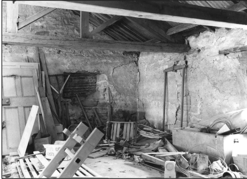
Plate 49: SW corner of first floor, looking S (photo 5/4).
