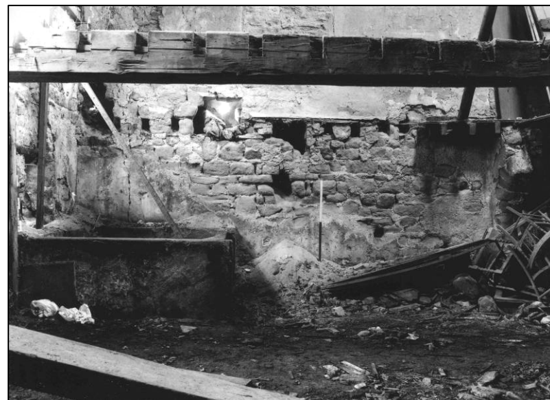
Plate 24: Complete stepping tank and ground floor S wall, looking SE (photo 3/5).
