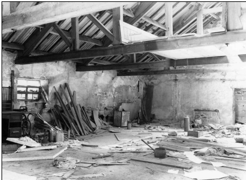
Plate 55: General view of first floor, looking W (photo 5/11).
