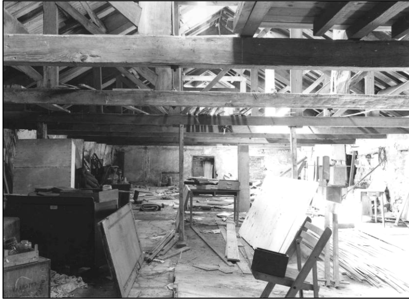
Plate 53: General view of first floor, looking NW (photo 5/7).
