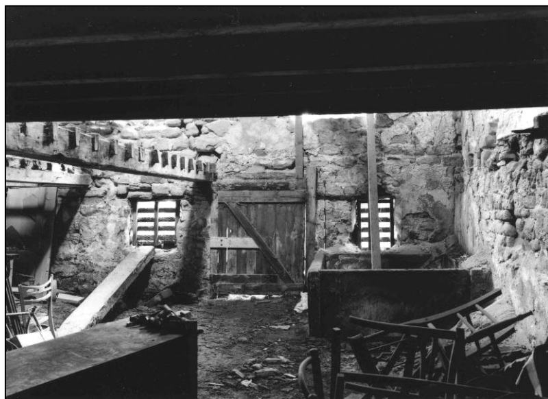
Plate 23: Complete stepping tank, SE corner of ground floor, looking NE (photo 3/4).
