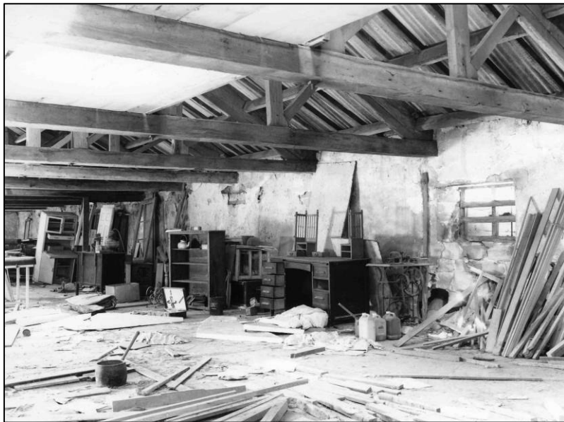
Plate 51: General view of first floor, looking W (photo 5/12).
