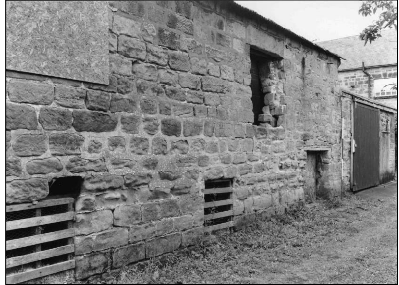
Plate 10: N end of E elevation, looking NW (photo 2/6).
