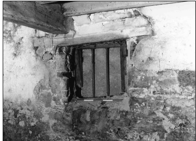
Plate 44: Original window, ground floor area W of spine wall, looking SW (photo 4/15).
