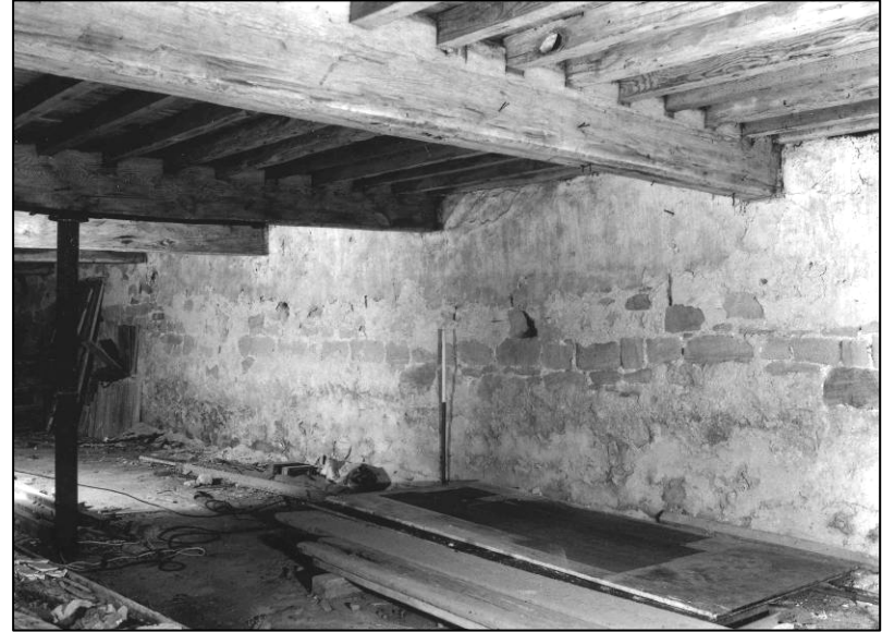
Plate 26: Recesses for cow stalls, E face of ground floor spine wall, looking S (photo 4/1).
