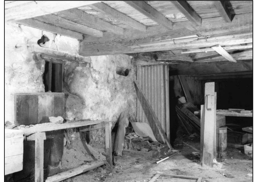
Plate 38: Joiner's bench and stove base, W wall of ground floor area W of spine wall, looking W (photo 4/8).
