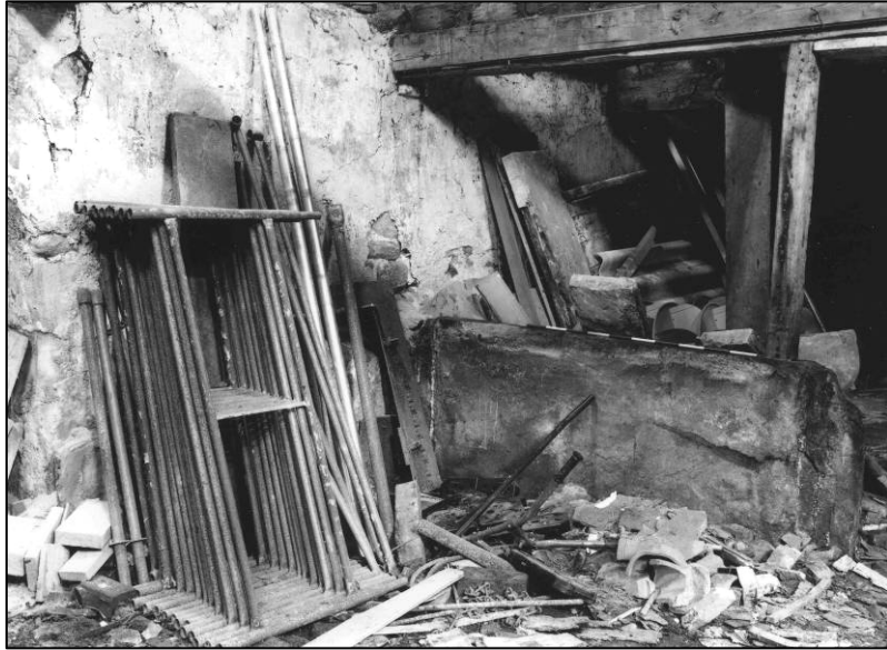
Plate 25: Incomplete steeping tank, SE corner of ground floor, looking W (photo 3/8).
