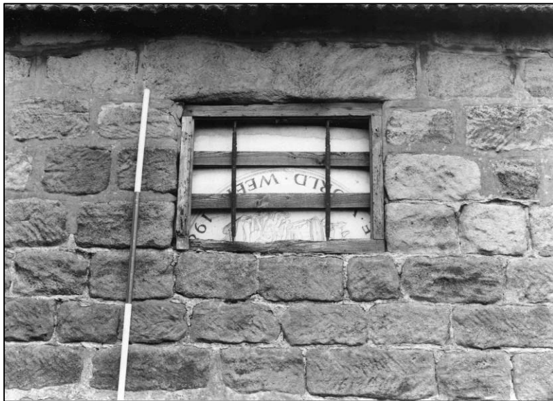
Plate 11: First floor E elevation, window with original fittings, looking SW (photo 2/11).
