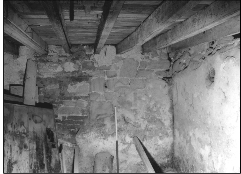
Plate 42: Blocked opening in W end of ground floor S wall, looking SE (photo 4/6).
