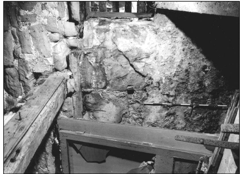
Plate 28: Possible blocked doorway, E wall of ground floor area E of spine wall, looking N (photo 3/11) (top to left).
