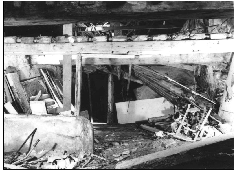
Plate 30: Incomplete steeping tank, SE corner of ground floor, looking NW (photo 3/10).
