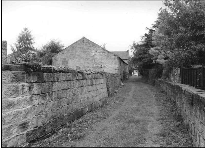
Plate 1: General view, looking NW along Prestons Ginnel (photo 1/18).
