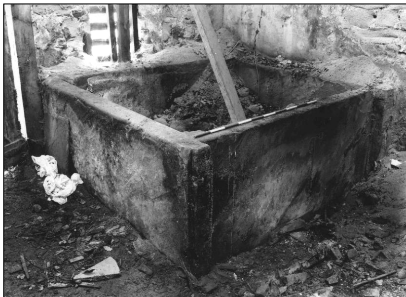
Plate 21: Complete stepping tank, SE corner of ground floor, looking E (photo 3/1).
