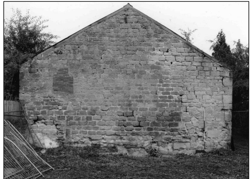
Plate 12: S gable, looking NW (photo 1/13).
