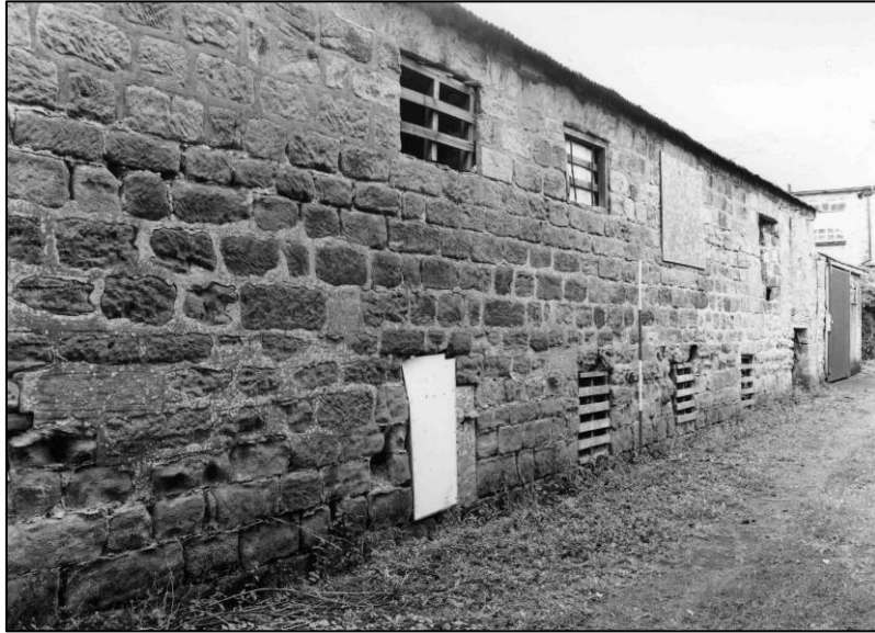
Plate 9: N end of E elevation, looking NW (photo 2/5).
