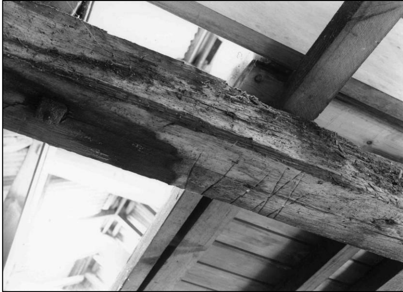
Plate 5: Typical incised mark to roof truss tie-beam, looking N (photo 5/5).
