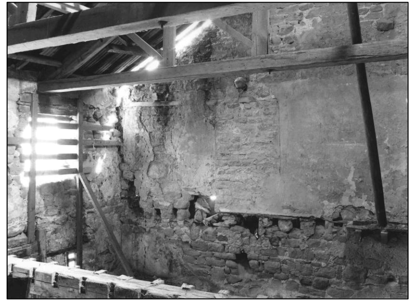
Plate 52: S wall of first floor, looking SE (photo 5/2).
