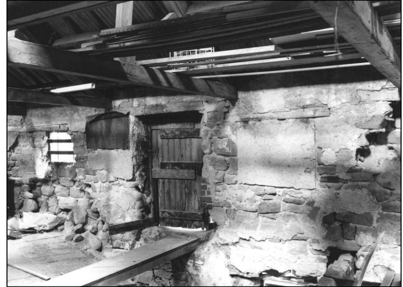
Plate 50: E wall of first floor (central part), looking N (photo 5/6).
