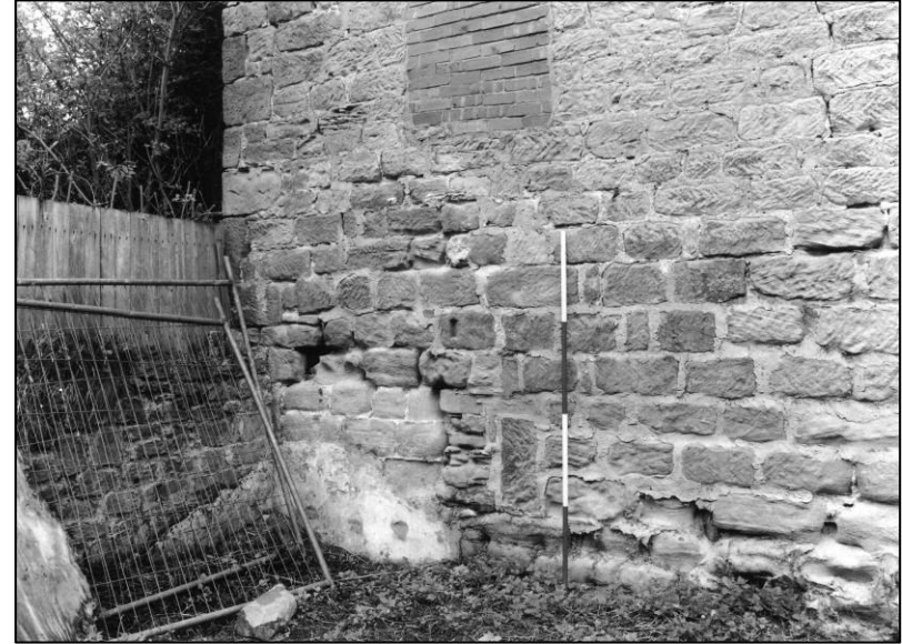
Plate 14: Detail of W end of S gable, looking W (photo 1/14).
