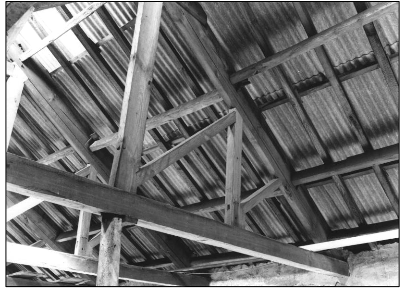
Plate 60: Detail of typical roof truss, looking NE (photo 5/16).
