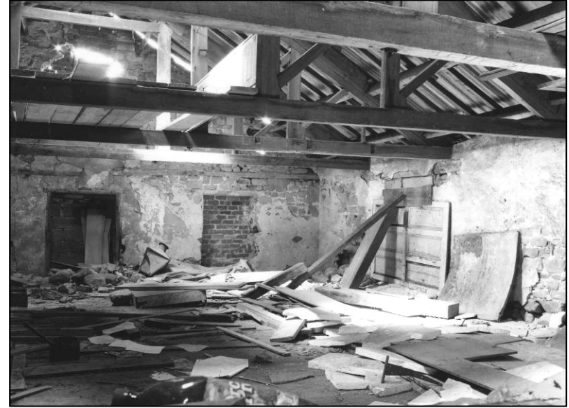
Plate 54: General view of first floor, looking N (photo 5/10).
