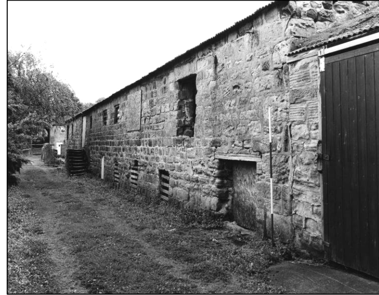
Plate 2: General view, looking S (photo 2/10).
