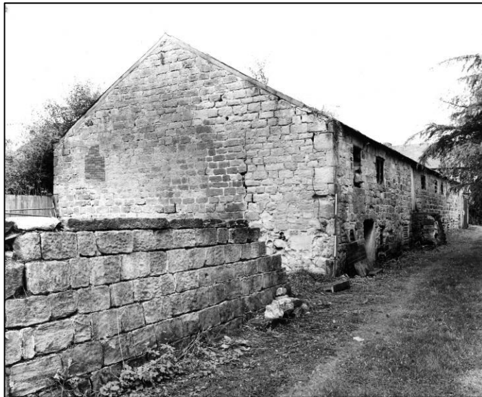
Plate 3: General view, looking W (photo 1/16).
