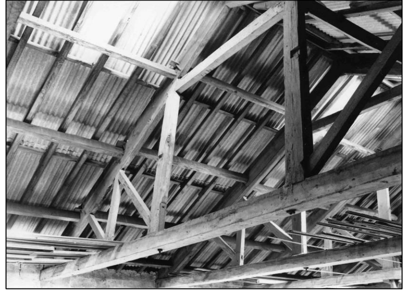
Plate 58: Typical roof truss, looking SE (photo 5/13).
