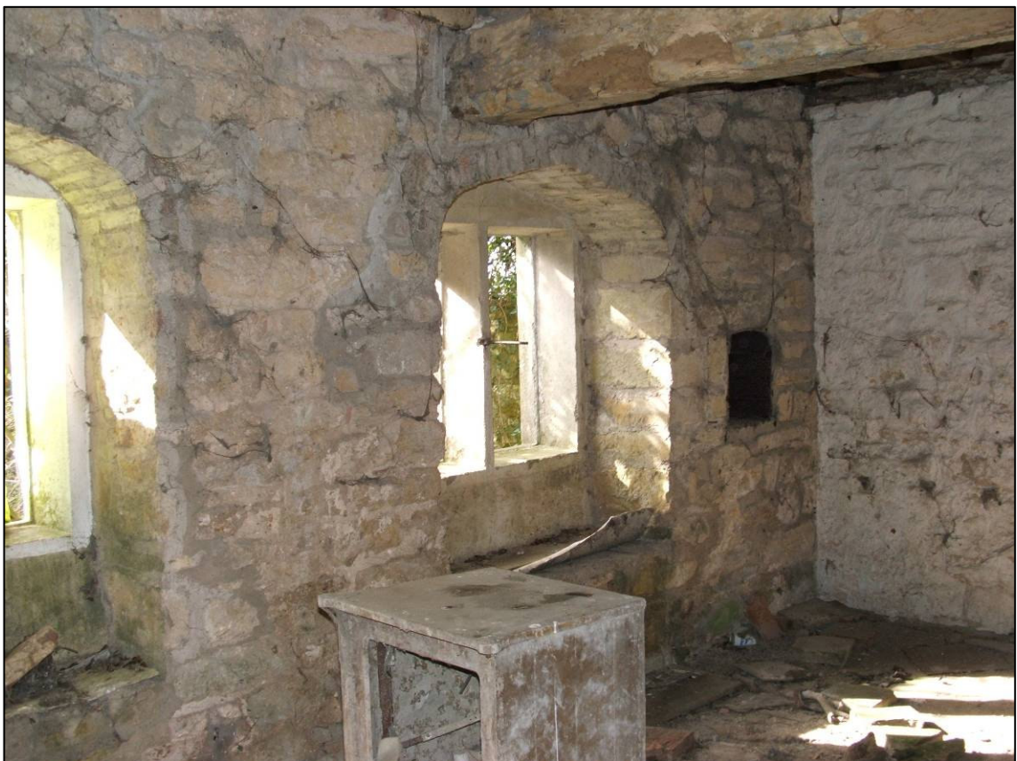
Plate 7: Ground floor of main building, looking SW.
