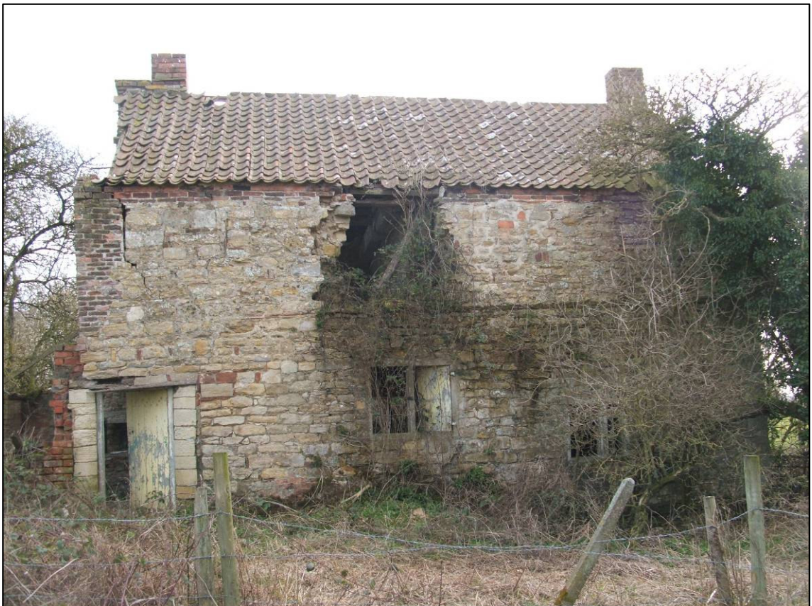
Plate 2: North elevation, looking S.
