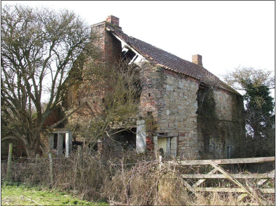
Plate 1: Abbey Cottage, looking SW.
