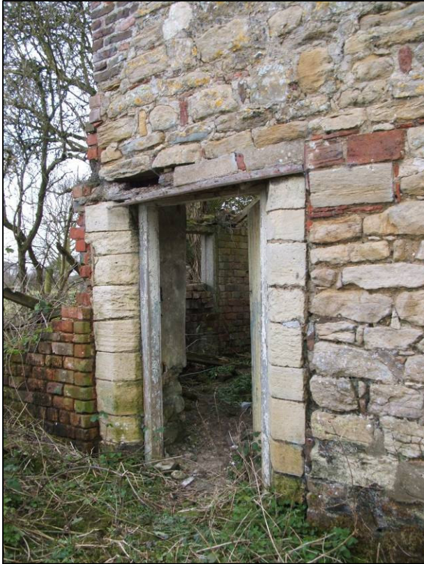
Plate 3: East doorway in north elevation, looking SW.
