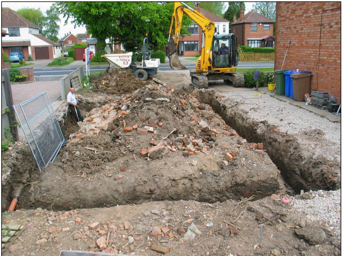
Plate 2: Completed foundation trenches for the house, looking N.
