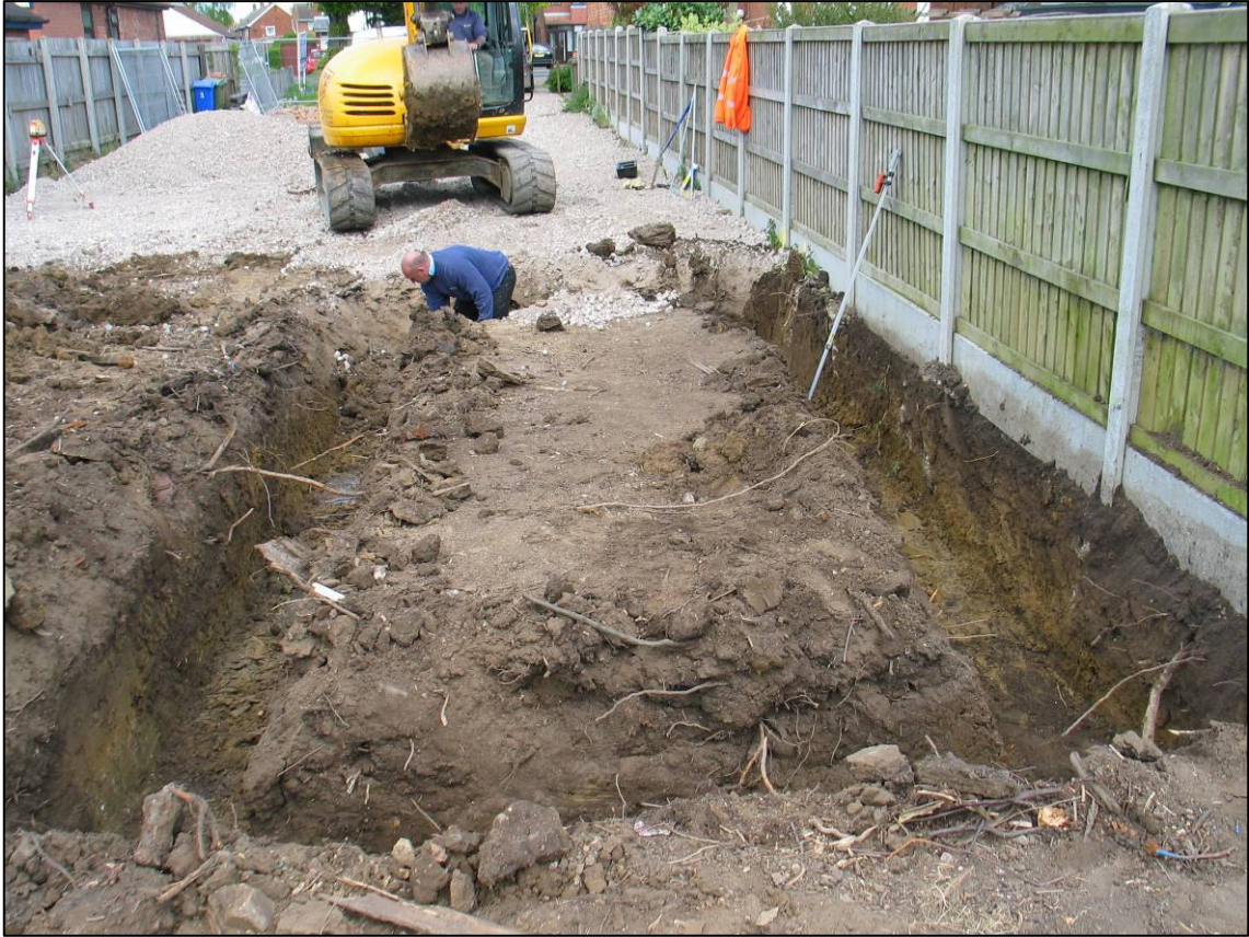
Plate 1: Excavating foundation trenches for the garage, looking N.
