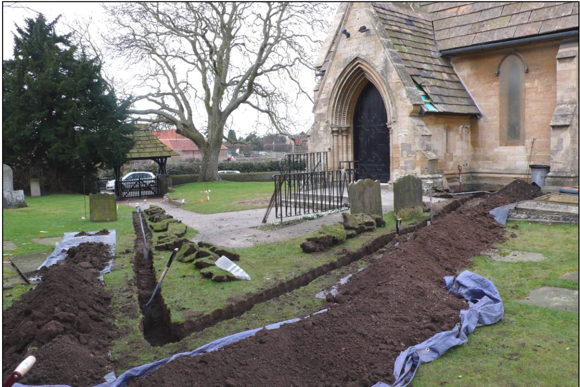
Plate 1: Trenches 2 and 3 under excavation, south side of the church, looking NW.
