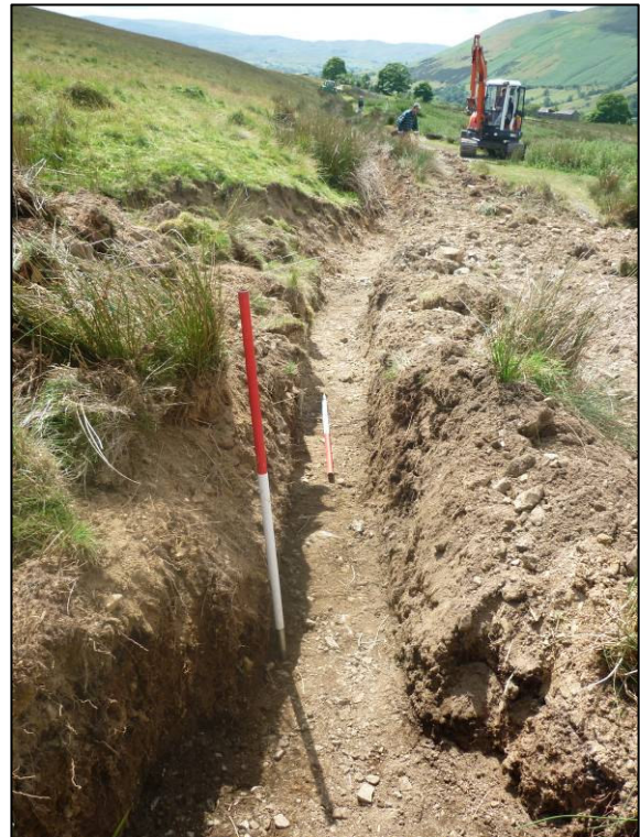
Plate 6: Re-cut ditch to north of culvert 2, looking SW.
