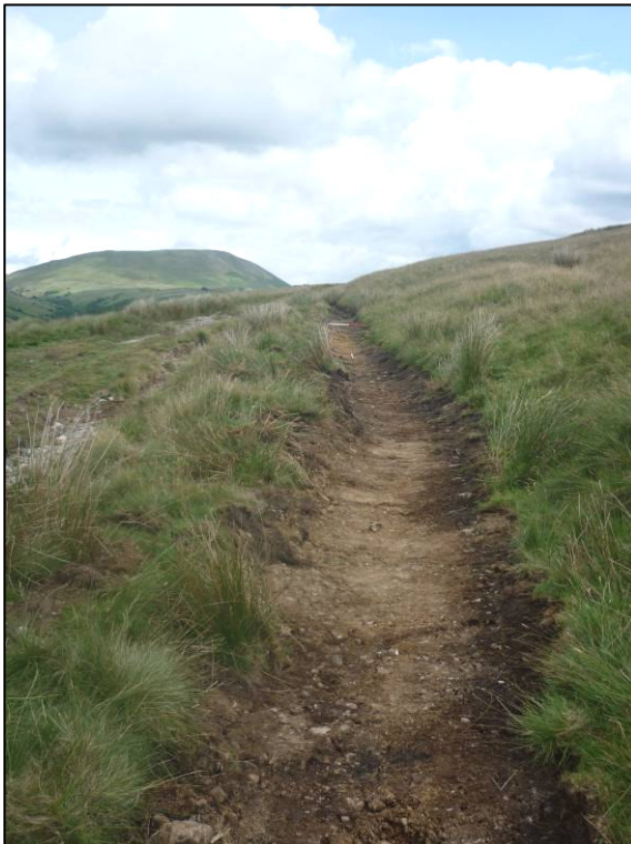
Plate 5: Re-cut ditch to north of culvert 1, looking NE.
