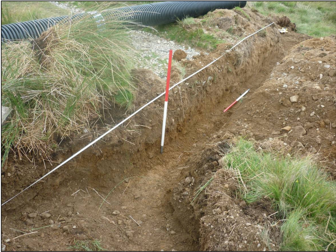
Plate 4: Trench for culvert 1, looking SE.
