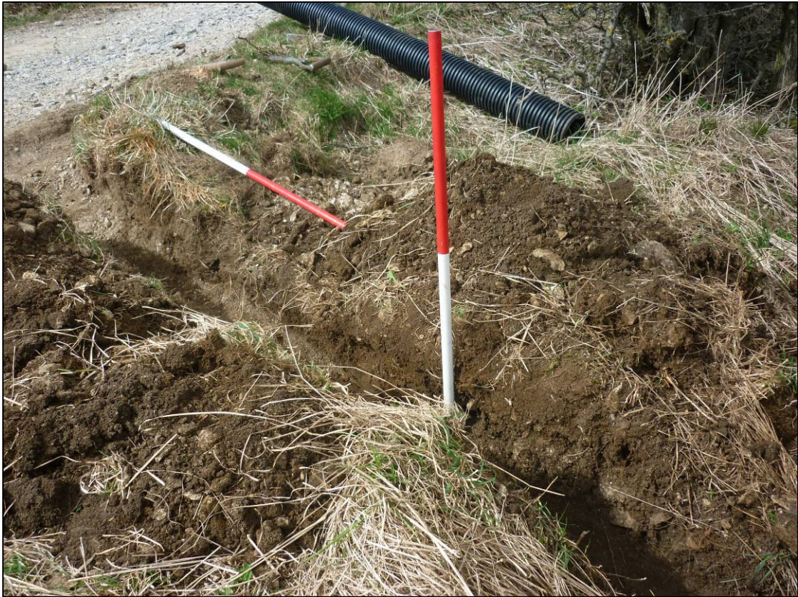
Plate 3: Excavated Trench 3, looking N.
