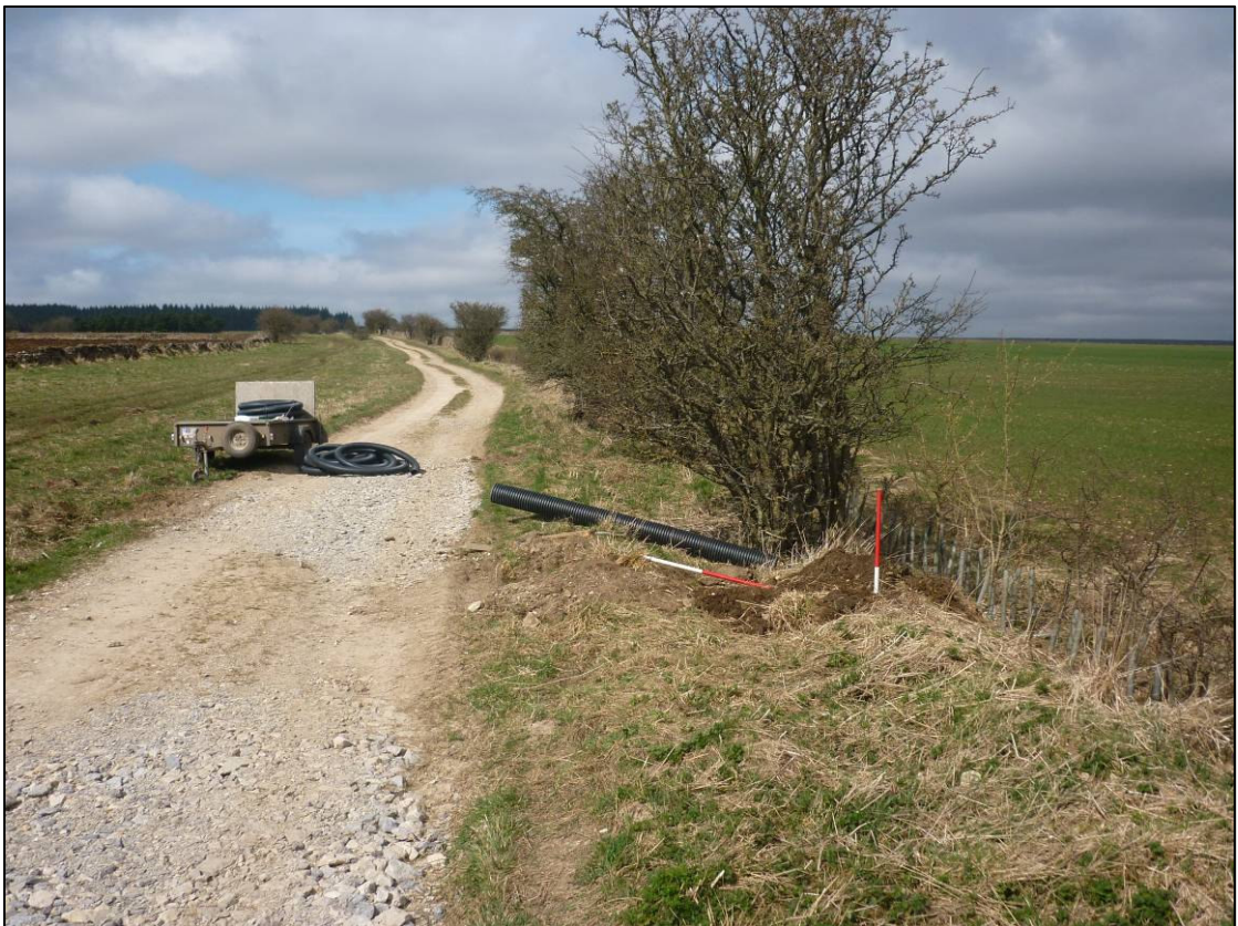
Plate 2: Trench 2 and Hambleton Road, looking N.
