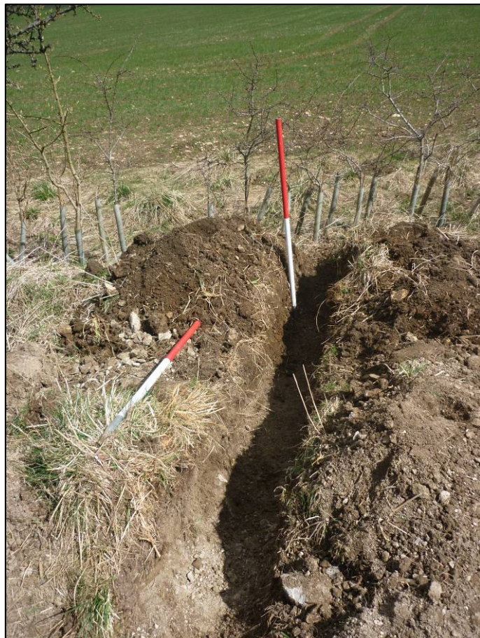
Plate 4: Excavated Trench 3, looking E.
