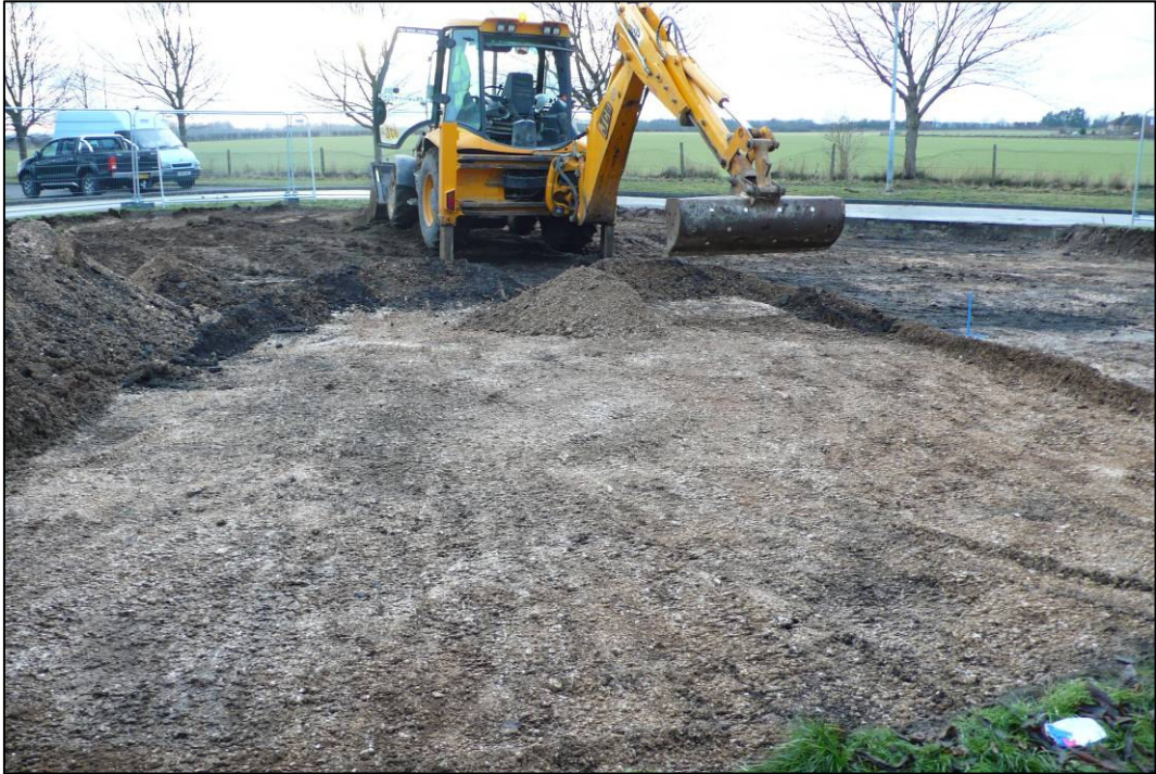
Plate 1: Topsoil strip in progress, looking SW.
