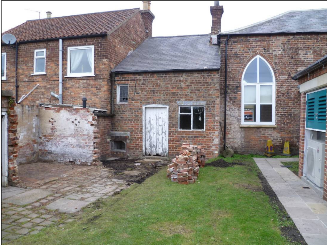
Plate 1: Rear of cottage prior to start of works, looking NW.
