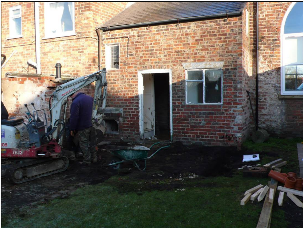
Plate 2: Excavations in progress, looking NW.
