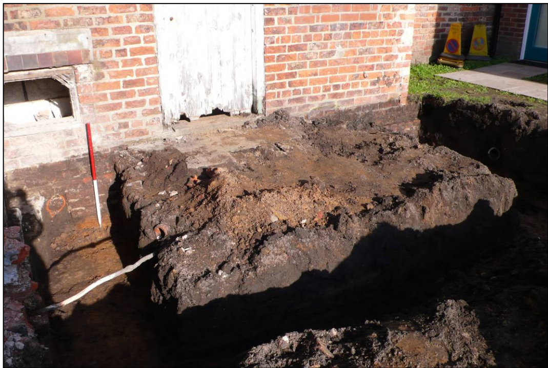
Plate 5: Excavations complete, looking NE.
