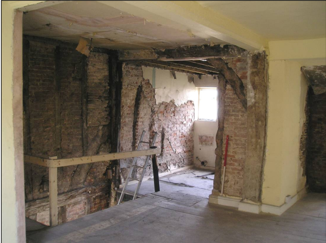
Plate 9: View into 1F7 showing scar of former lean-to roof and posts to east wall of 1F6, looking N (photo 33/12).
