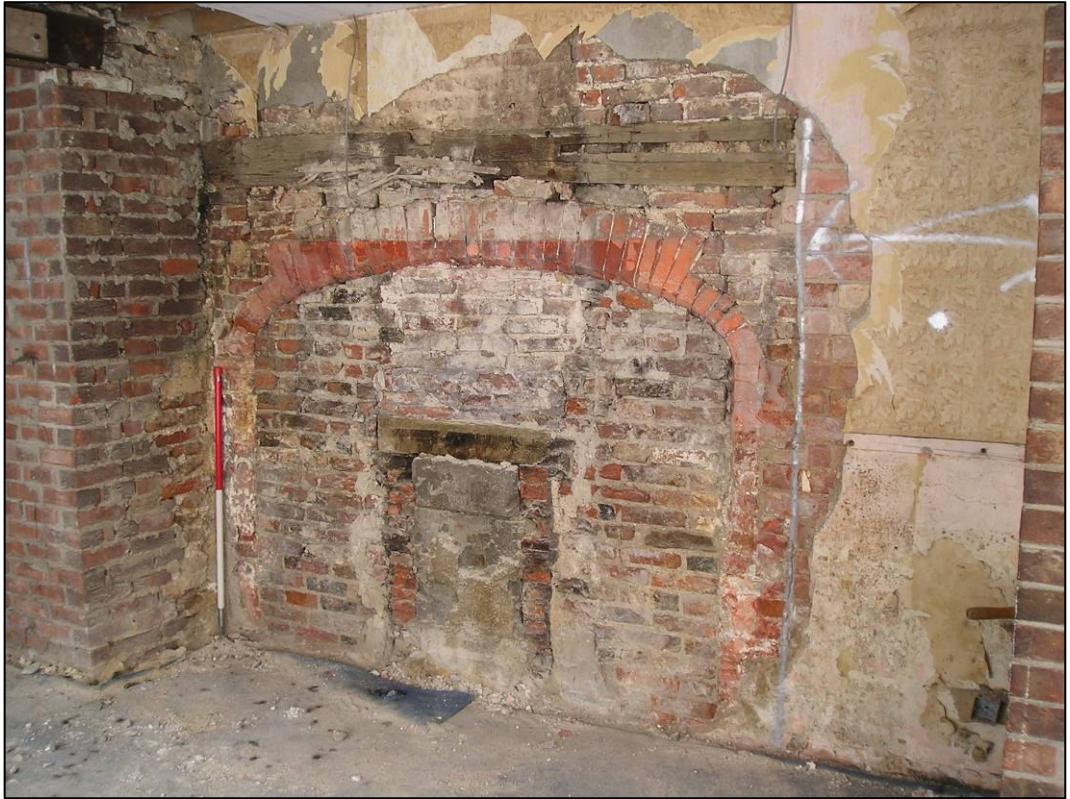
Plate 11: Fireplace in east wall of GF2 when first exposed, looking N (photo 31/22).
