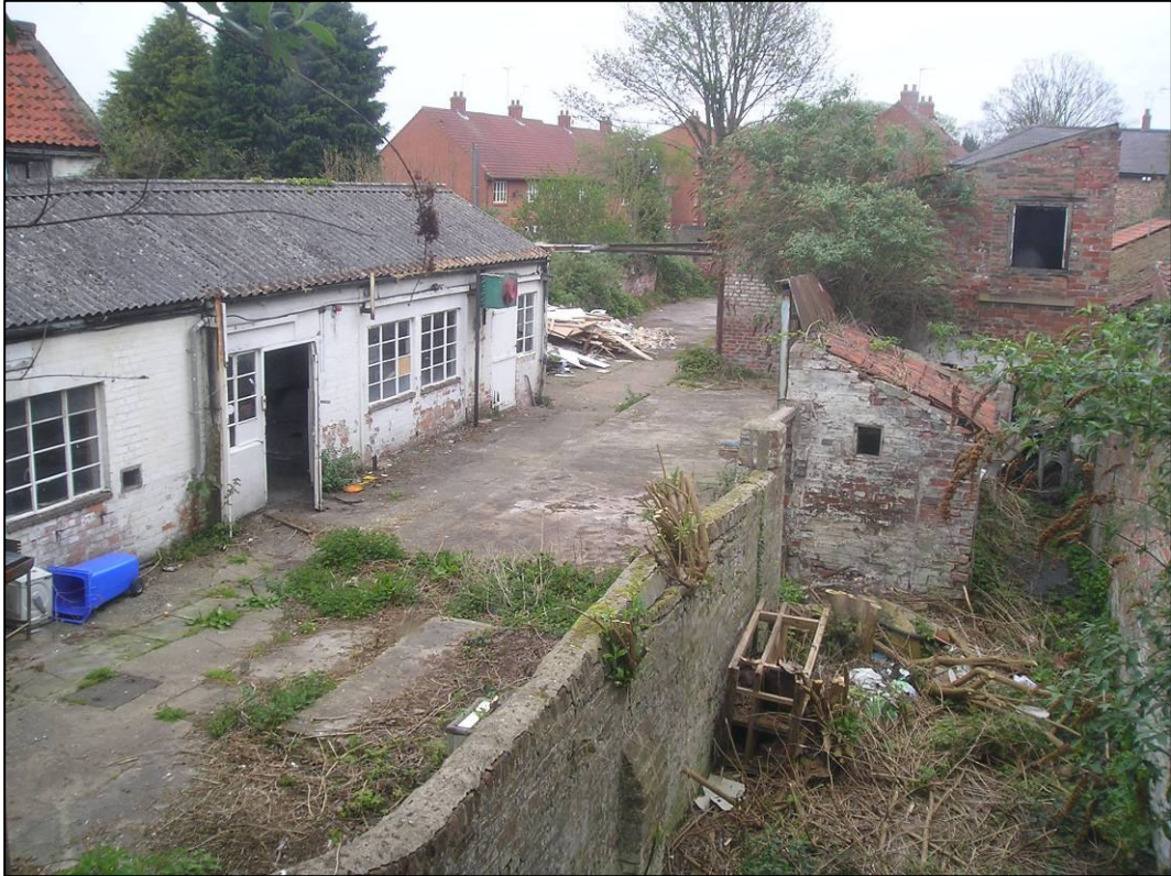
Plate 15: Rear yard, prior to clearance, showing Buildings A to G, looking NE (photo 30/5).
