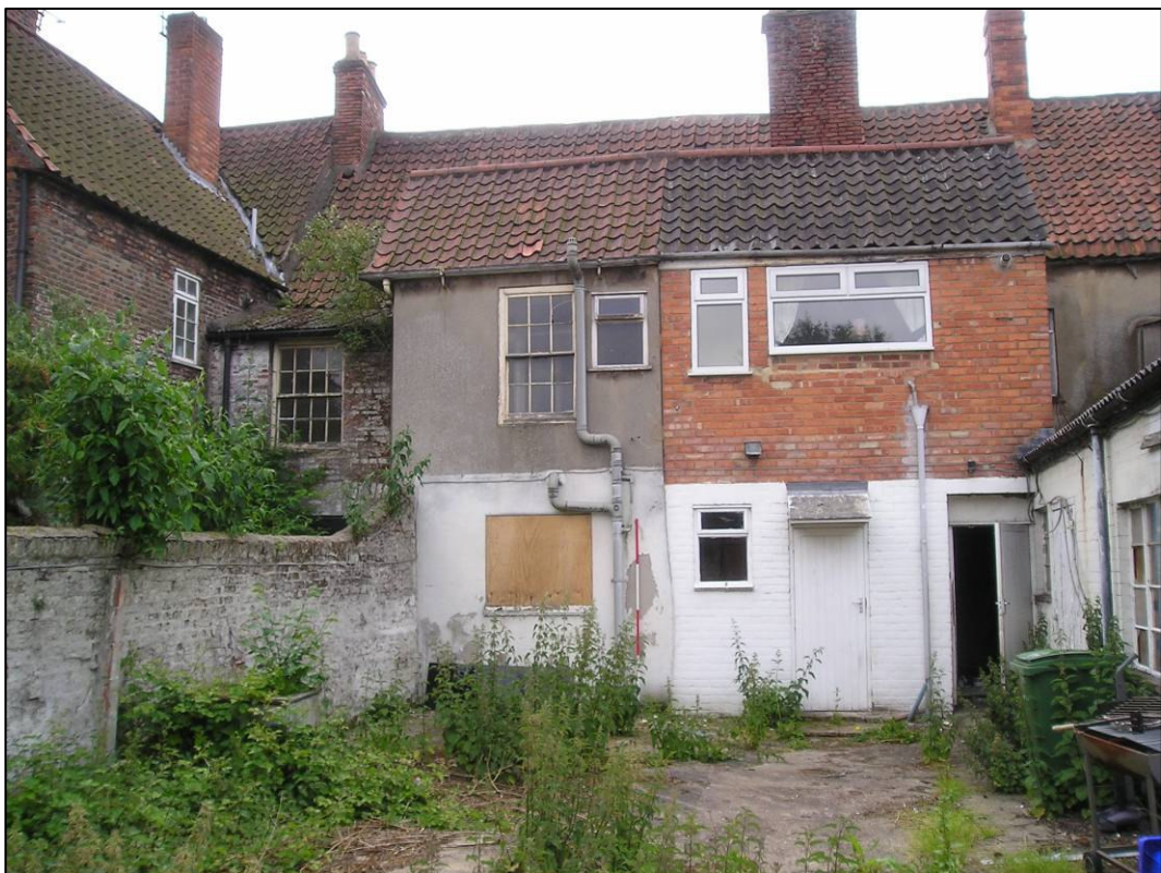
Plate 6: Nos. 32-36 North Bar Within, east (rear) elevation, looking W (photo 31/30).
