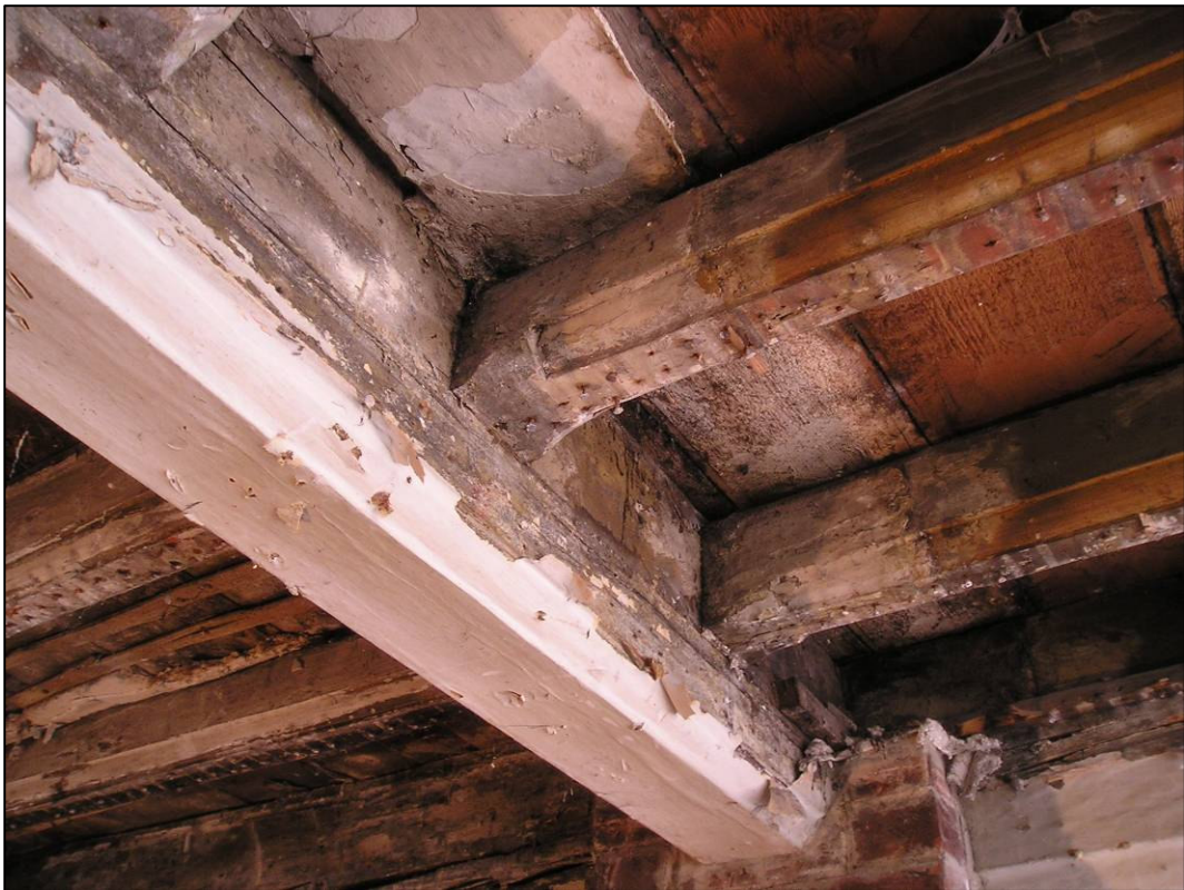
Plate 10: Moulded beams and joists over 1F6, looking W (photo 40/18).
