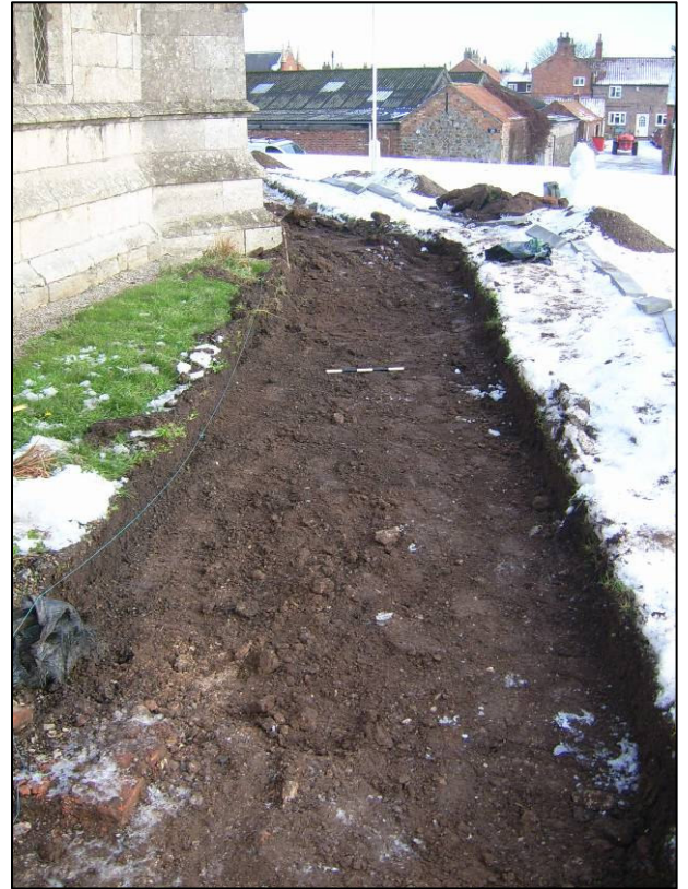
Plate 4: Excavations for new path, looking NE.
