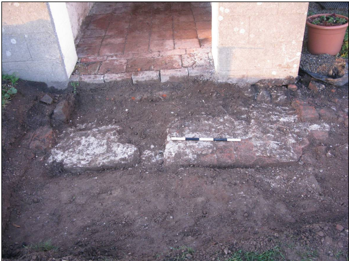
Plate 7: Foundations of earlier south porch, looking N.
