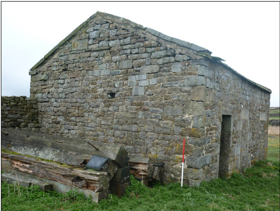
Plate 15: West gable of garage building, looking NE (photo 1/327).
