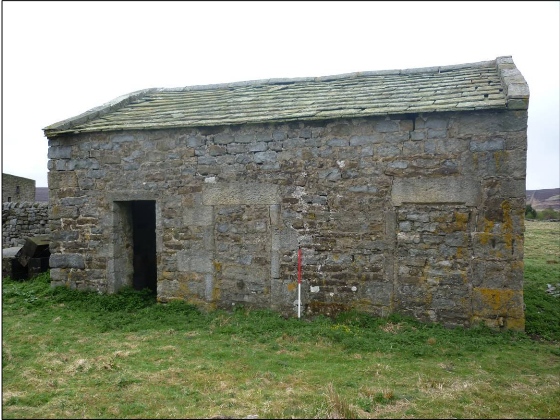
Plate 14: South elevation of garage building, looking N (photo 1/324).
