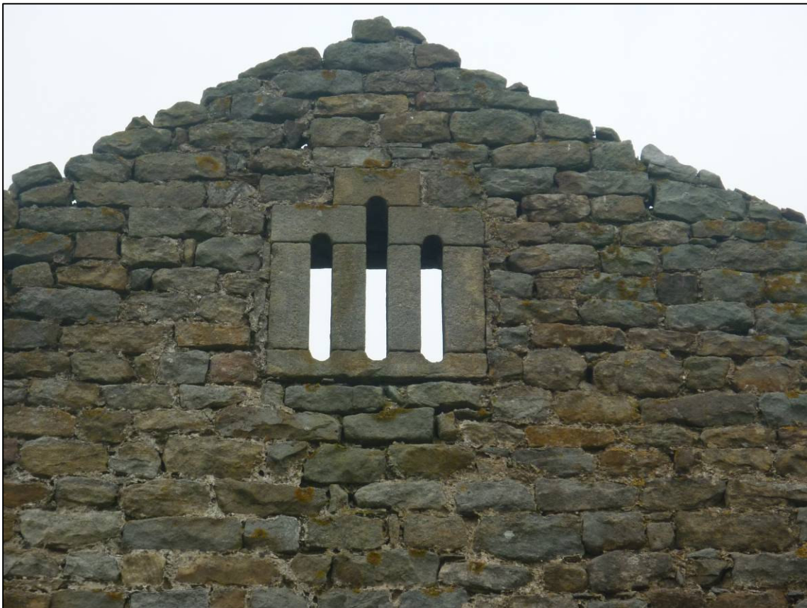
Plate 13: Detail of opening in apex of south gable of barn, looking N (photo 1/374).
