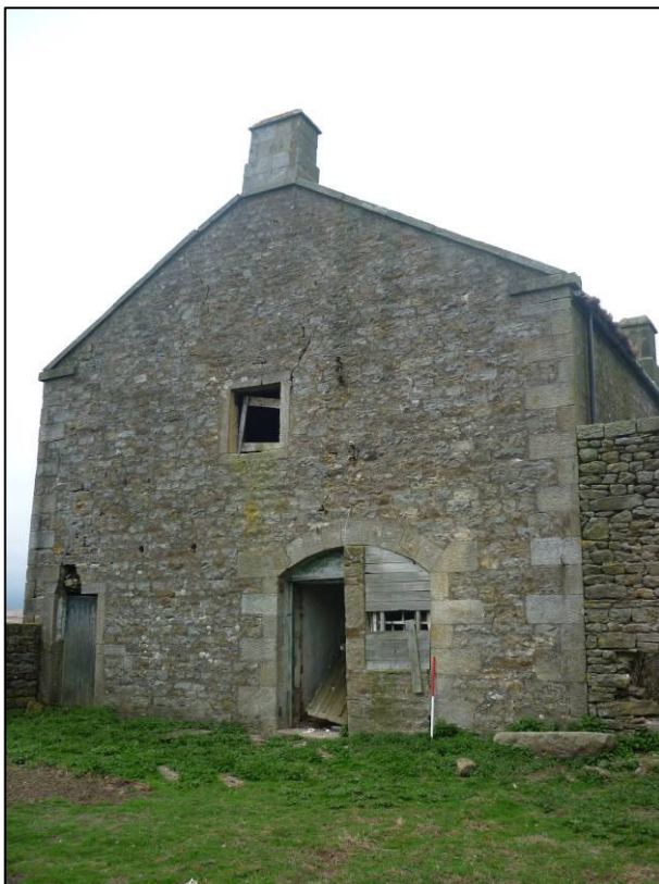
Plate 8: South gable of house, looking NW (photo 1/403).
