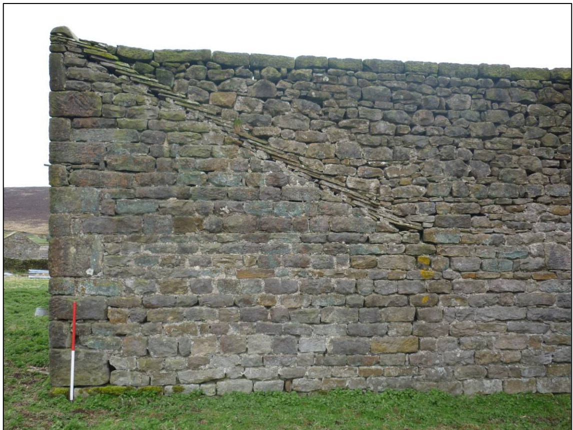
Plate 11: North gable of east range, looking S (photo 1/355).
