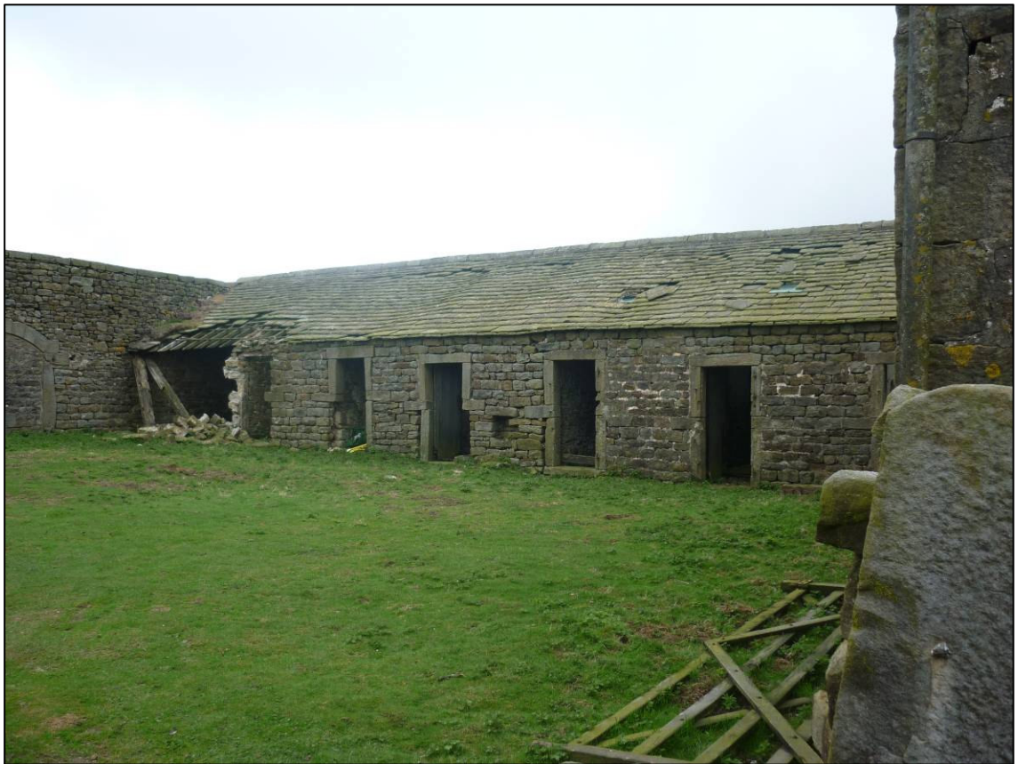
Plate 10: West elevation of east range, looking N (photo 1/380).
