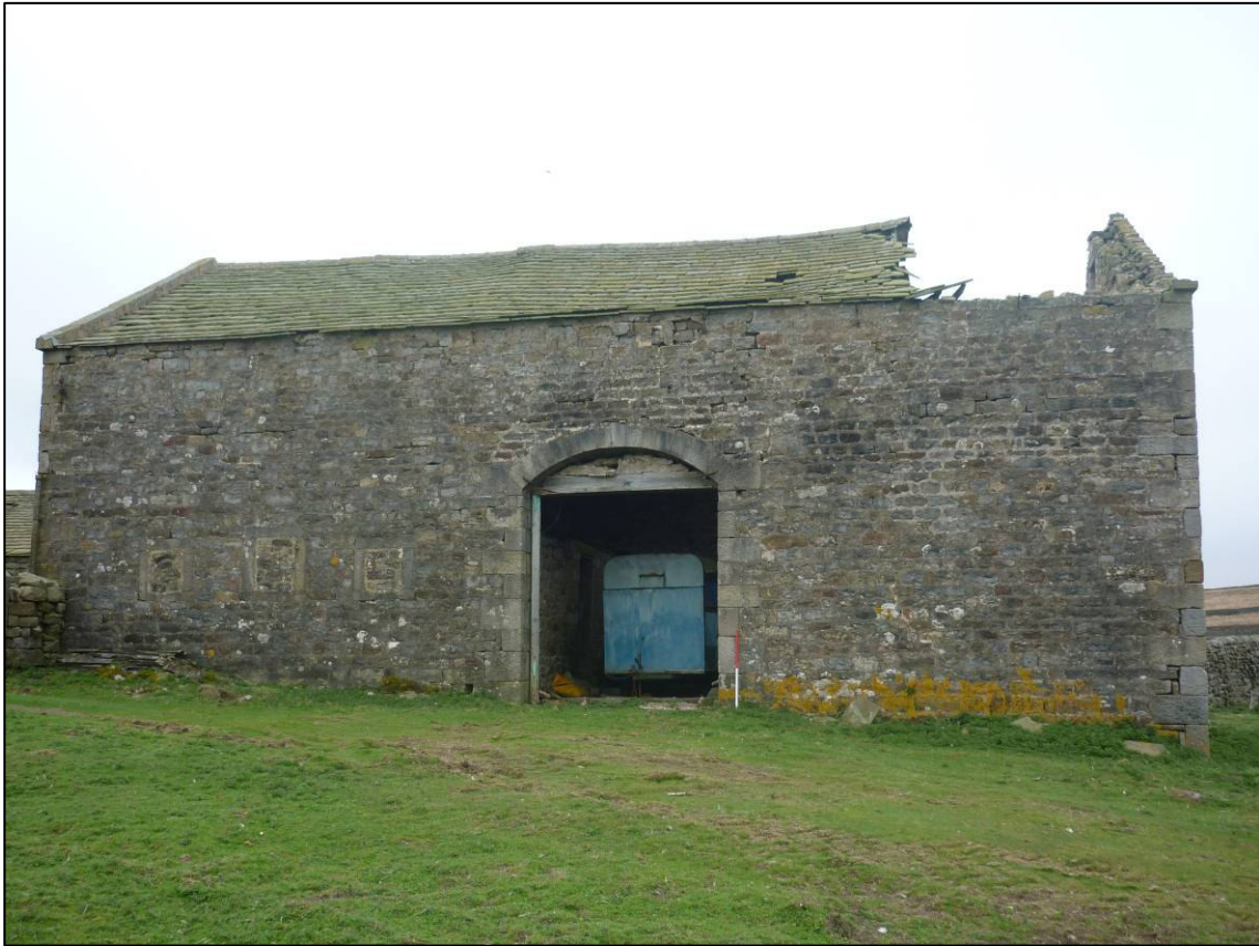
Plate 12: Barn, W elevation, looking E (photo 1/375).
