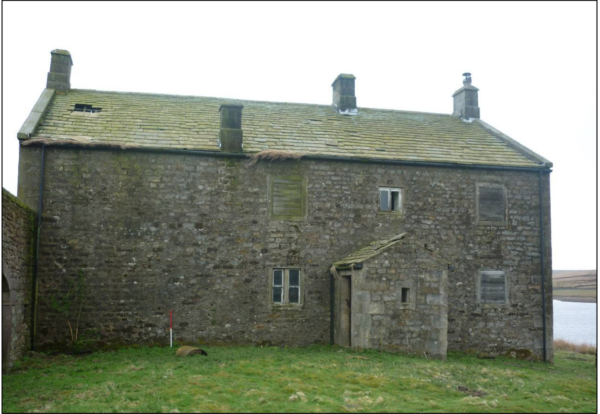
Plate 7: East elevation of house, looking W (photo 1/357).
