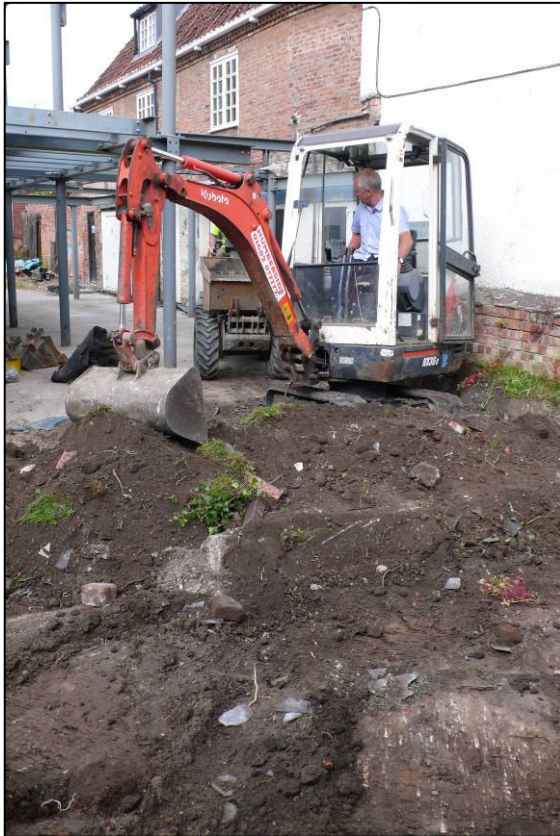
Plate 3: Topsoil strip in progress, looking W.
