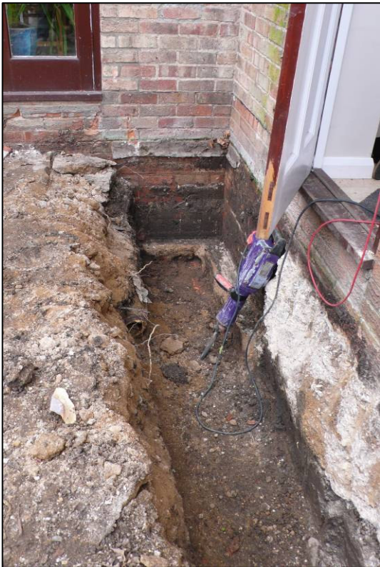
Plate 1: General view of North Trench, looking SW.
