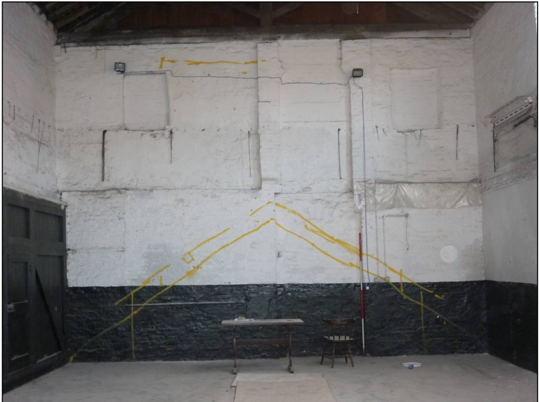
Plate 5: Internal west wall of standing building, looking SW.
