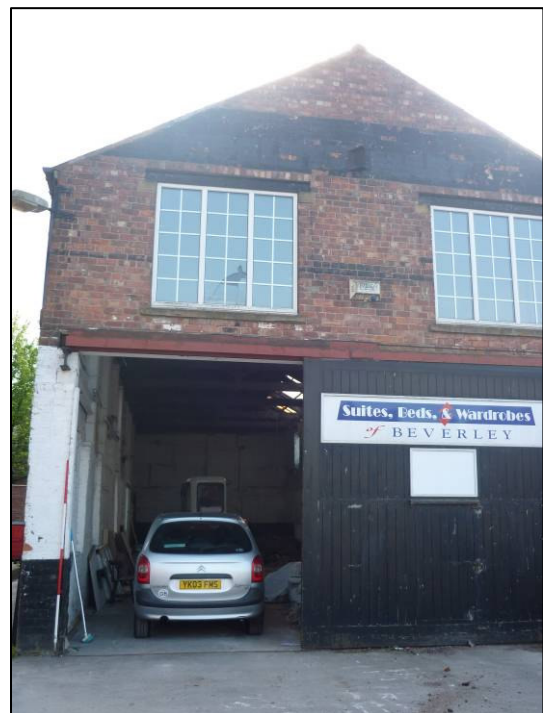
Plate 3: East gable of standing building, prior to conversion, looking W.
