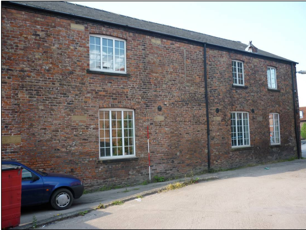
Plate 1: East end of south elevation of standing building, prior to conversion, looking N.
