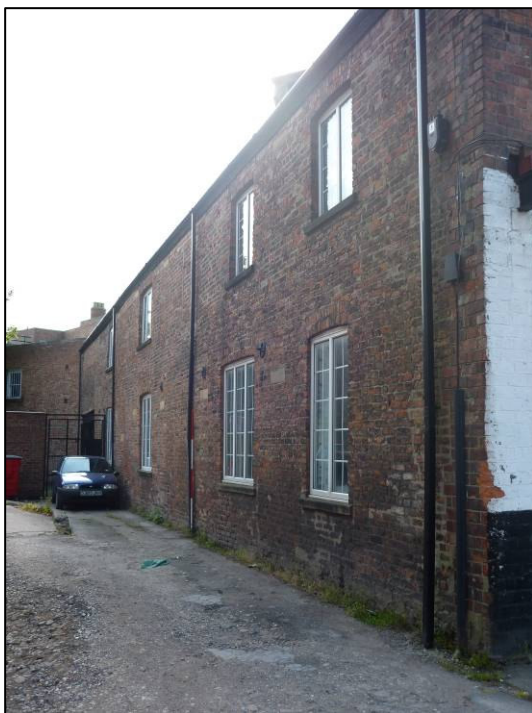
Plate 2: South elevation of standing building, prior to conversion, looking SW.
