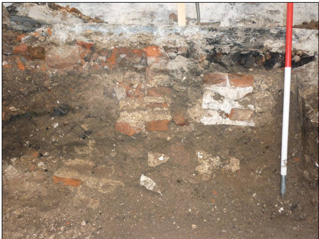
Plate 8: South side of Trench C (section 4), showing brick/chalk foundations [023 and 014], looking S.
