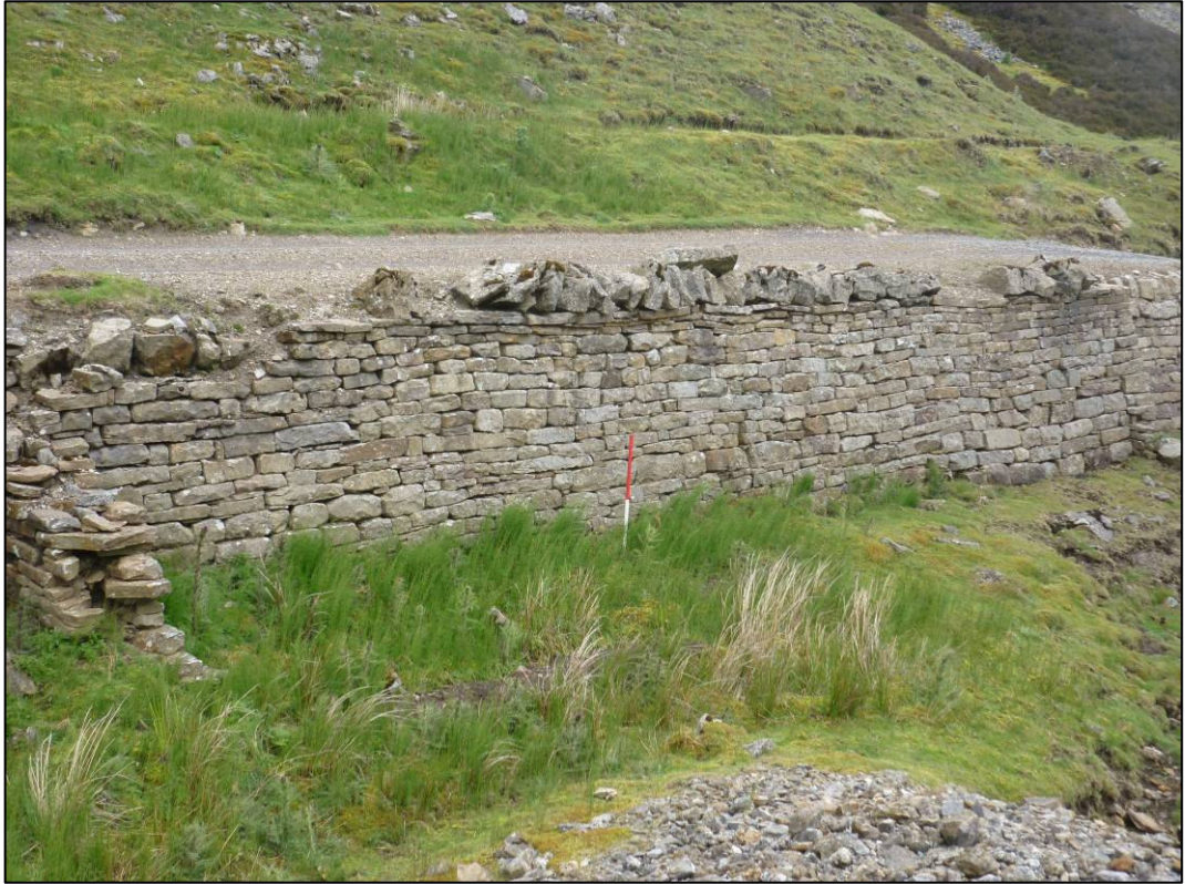
Plate 1: Retaining wall immediately to east of bouse teams, looking E (photo 1/392).
