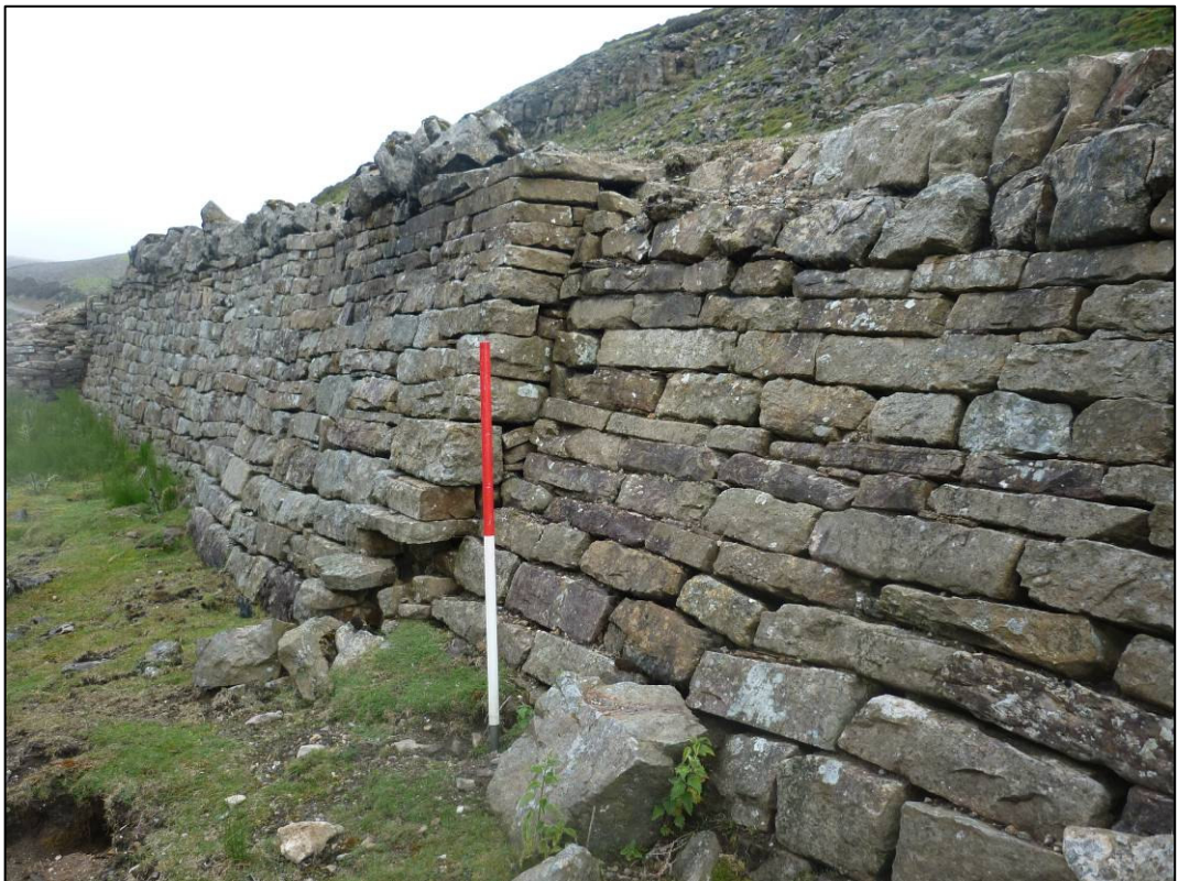
Plate 2: Step in retaining wall, looking N (photo 1/394).
