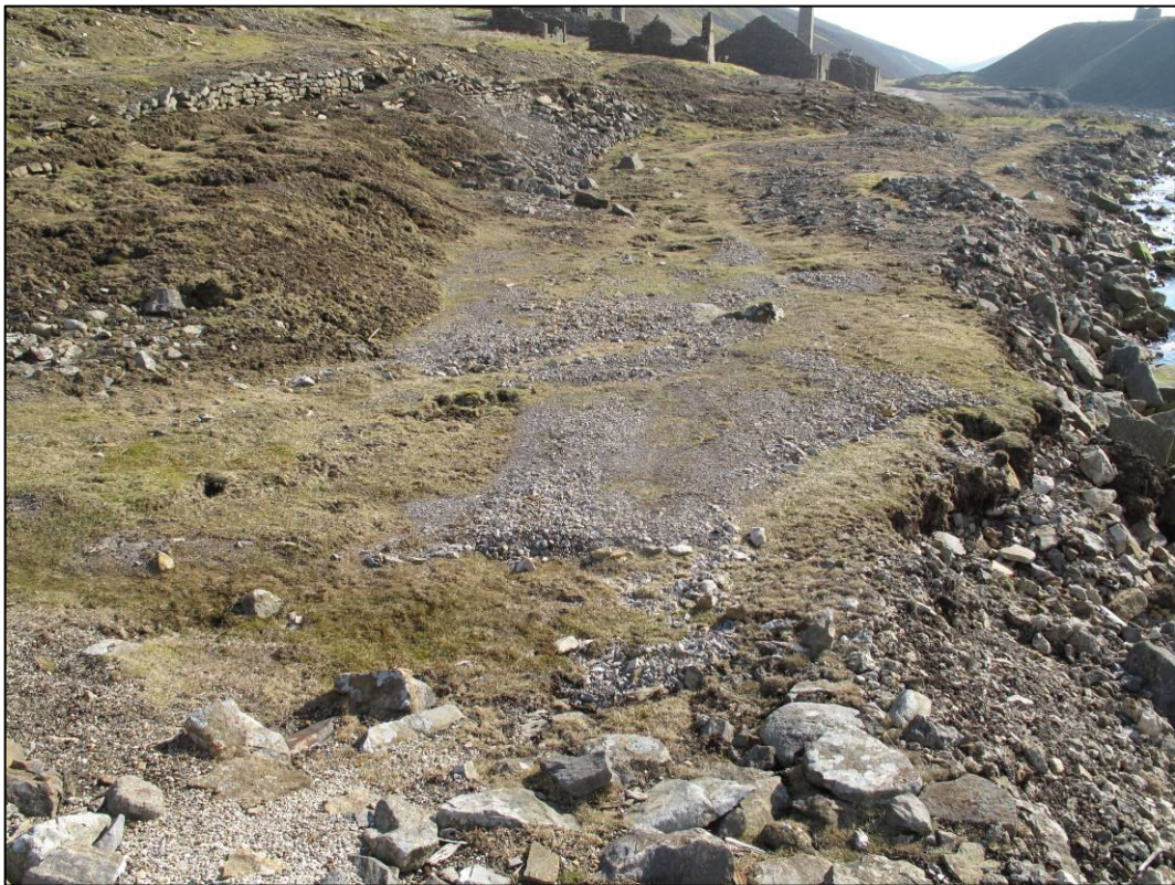
Plate 8: Limestone chippings washed off track onto dressing floor, March 2011 (YDNPA photo 2041).
