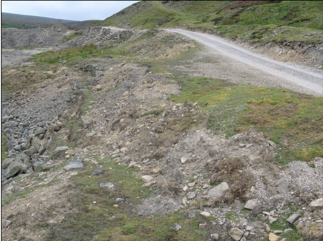
Plate 7: Dumping of material from unauthorised drainage works, September 2007 (YDNPA photo 1630).
